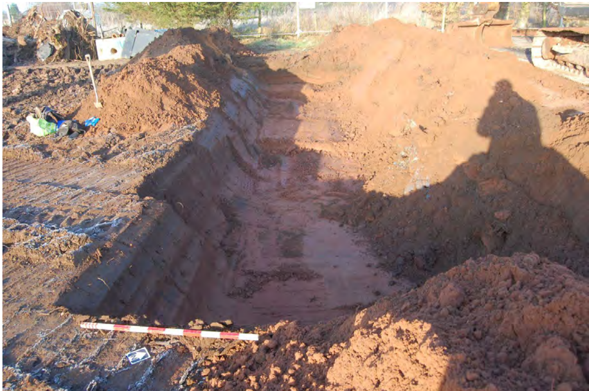
6. Trench T1, looking east
