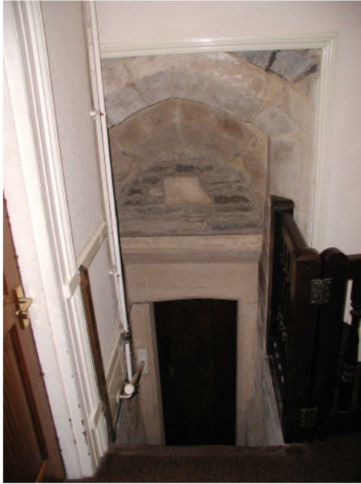
Fig 19: Arch stair to C1 in G9
