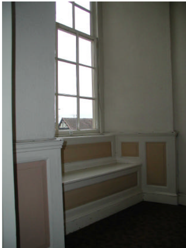
Fig 22: Dado panelling and window seat in F6
