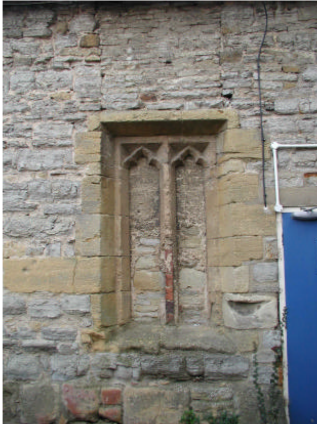
Fig 9: Two-light window in the N wall of the Cottage
