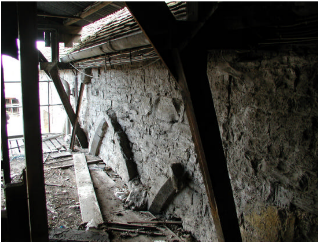
Fig 18: Series of vault arches (upper floor of timber store) G14b
