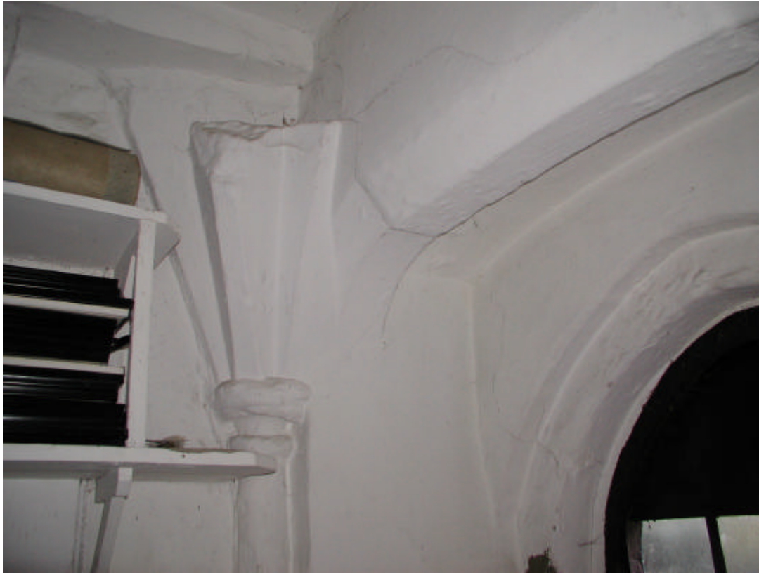
Fig 17: Column, capital and vault springing in G13a
