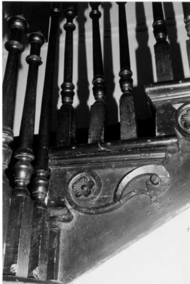
Fig 16: Stair 2: Scrolled brackets in G9
