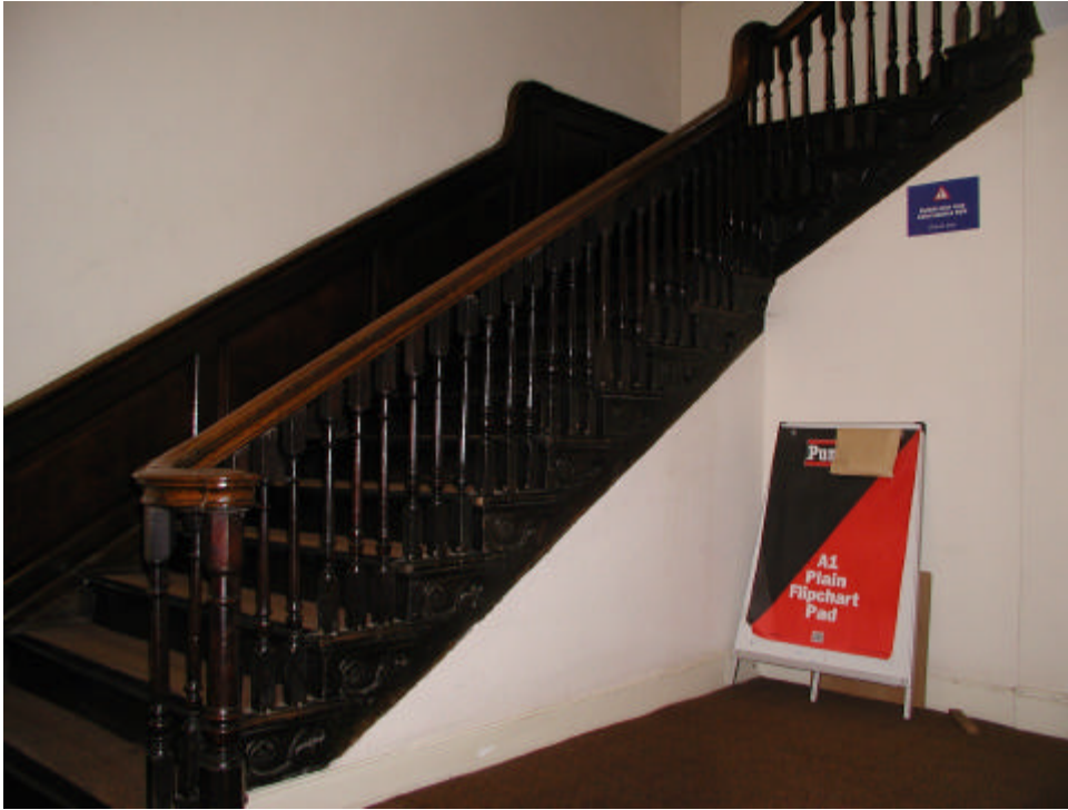
Fig 15: Stair 2: Principal stair in G9
