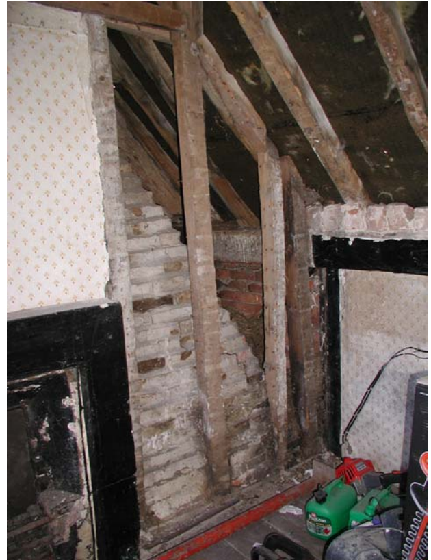
Fig 15: Inserted fireplace and chimney (U1)
