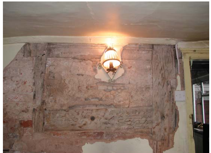
Fig 12: Timber frame in north wall (G3)
