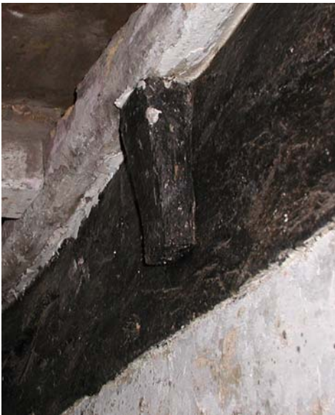
Fig 9: Detail of beam (G1)
