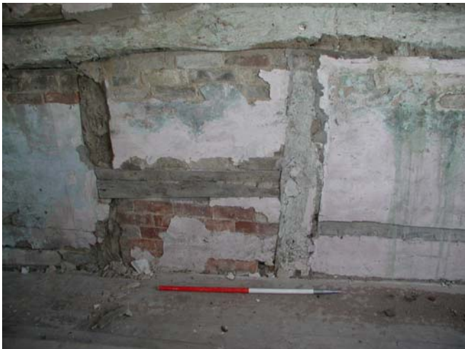
Fig 14: Detail of timber frame in north gable wall (U2)
