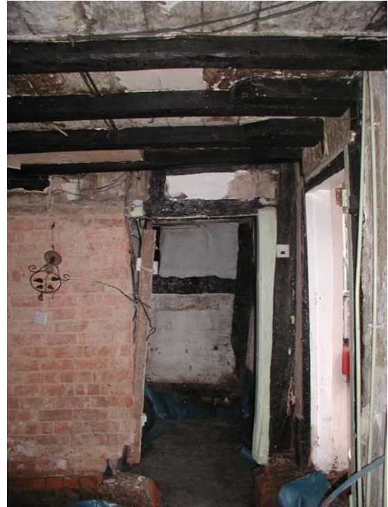
Fig 11: Exposed beams and doors (G1 and G2)
