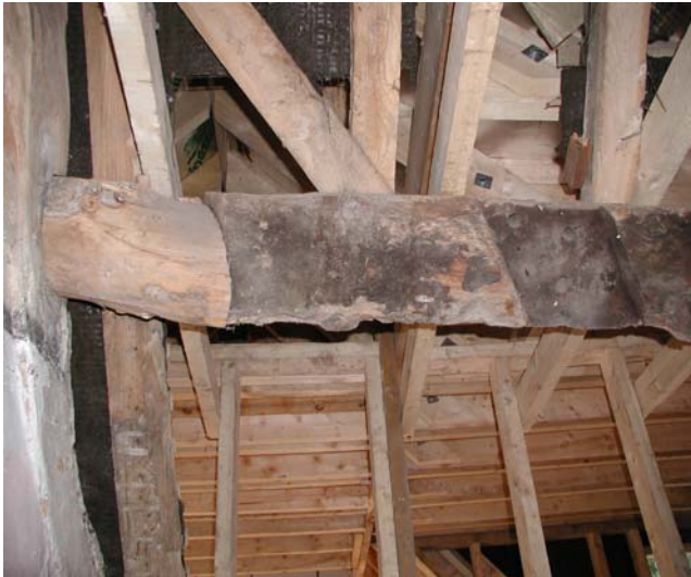
Fig 22: Reused roof beam (U2)
