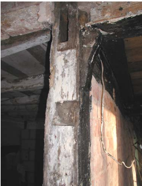
Fig 10: Detail of doorframe (G1)
