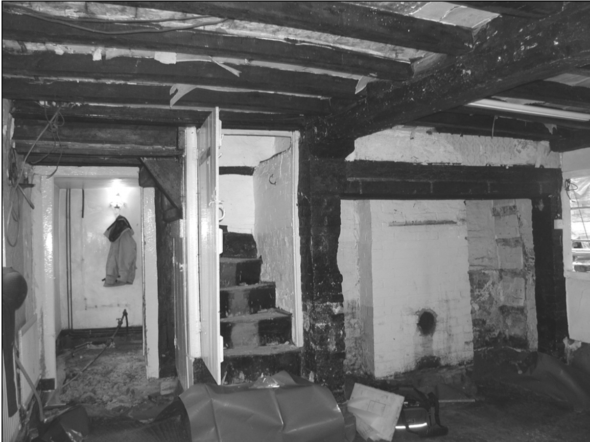
Fig 6: Room G1 showing exposed beams, stairs and fireplace
