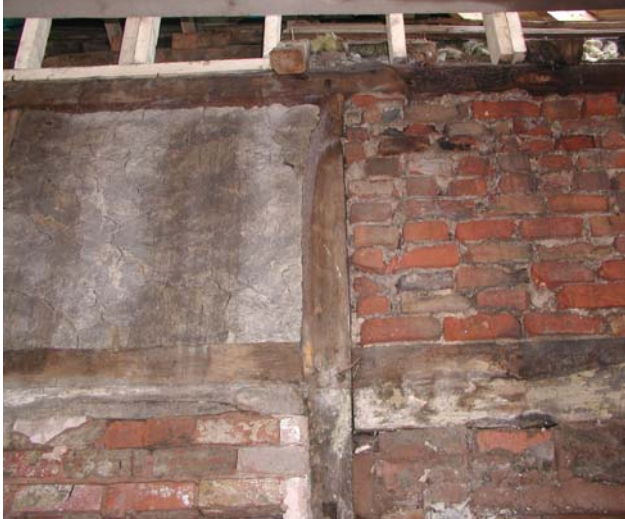
Fig 21: Detail of timber frame showing brick nogging infill
