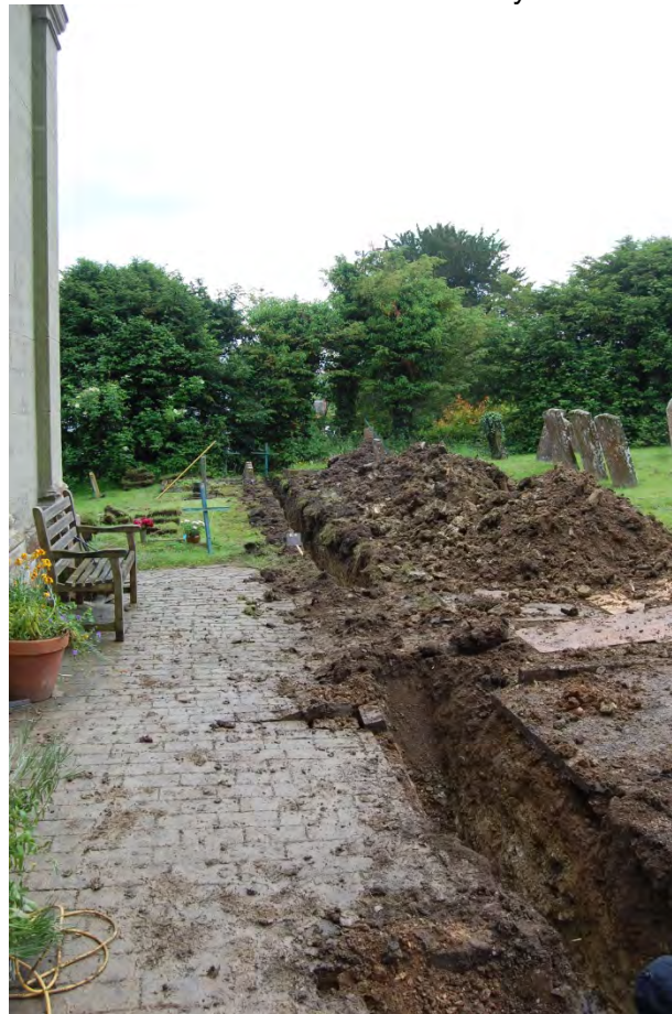
2. Excavated soakaway trench
