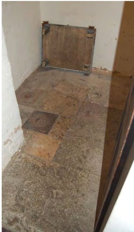
3. Vestry floor (4) with iron access covers (7)
