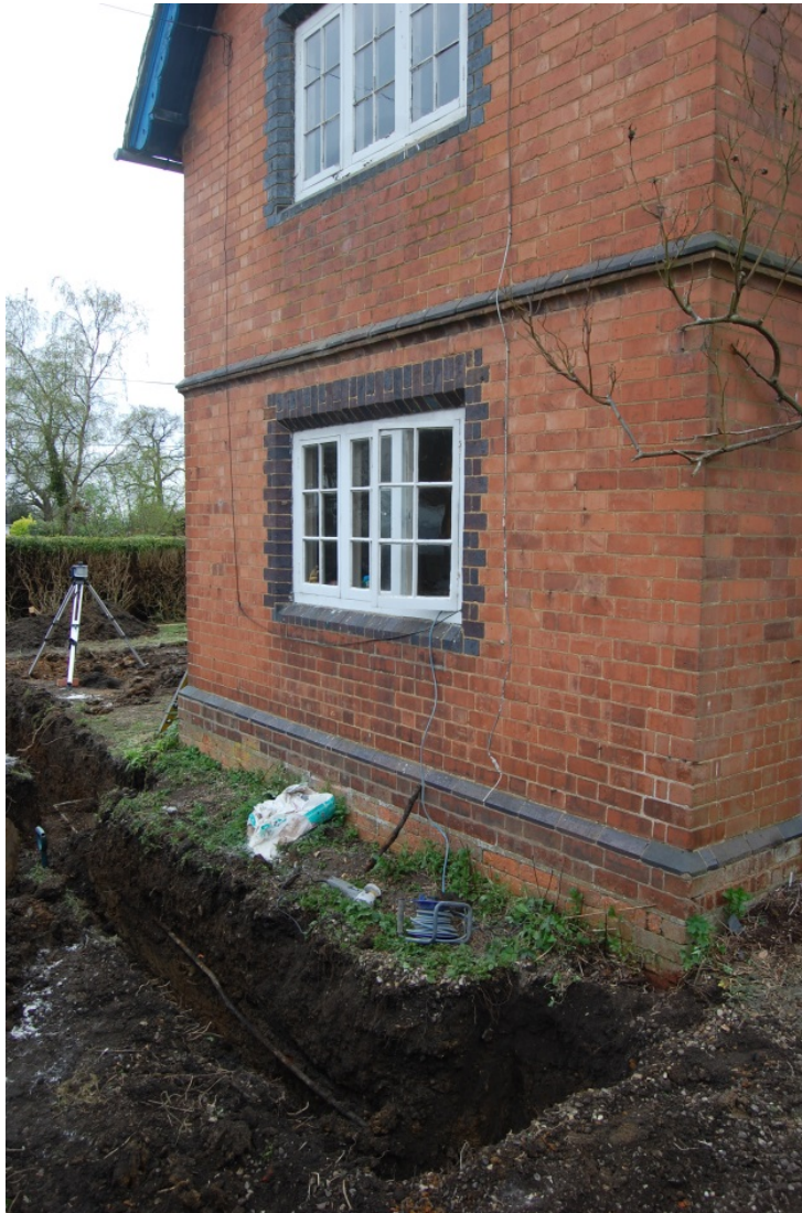
3. Foundation trenches to east of existing house
