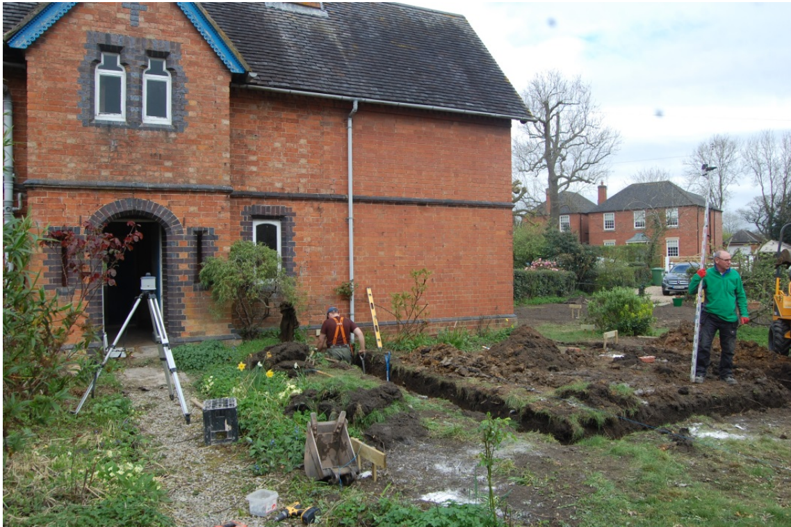
1 View northwards showing ground reduction
