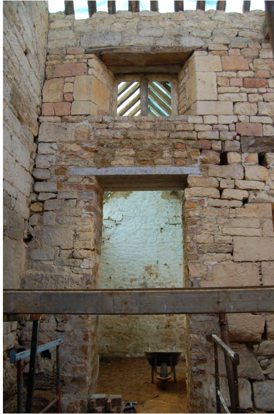
Fig 26: Looking from Room B into room C through newly cut door
