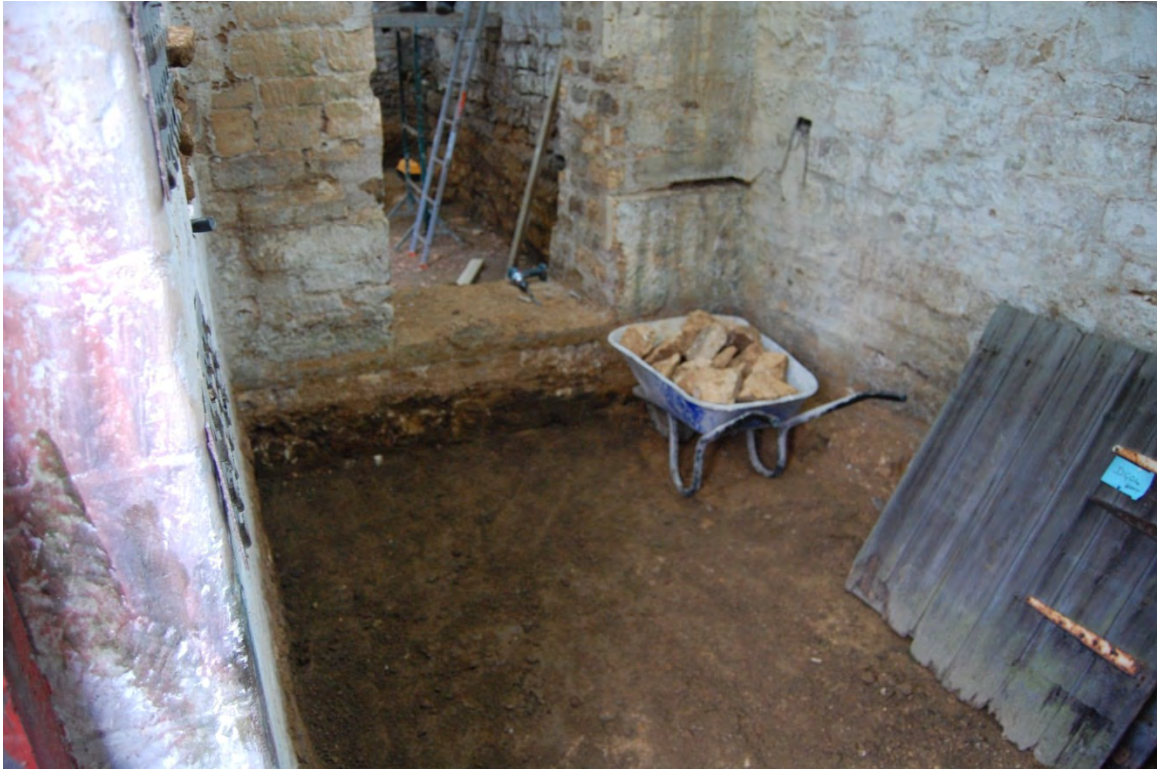
Fig 28: Reduced floor in room C
