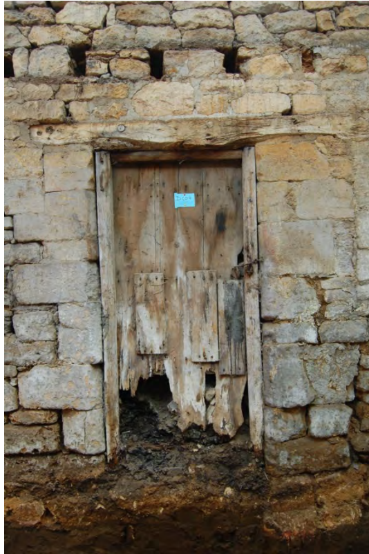
Fig 24: Interior of blocked doorway in east wall of Room B
