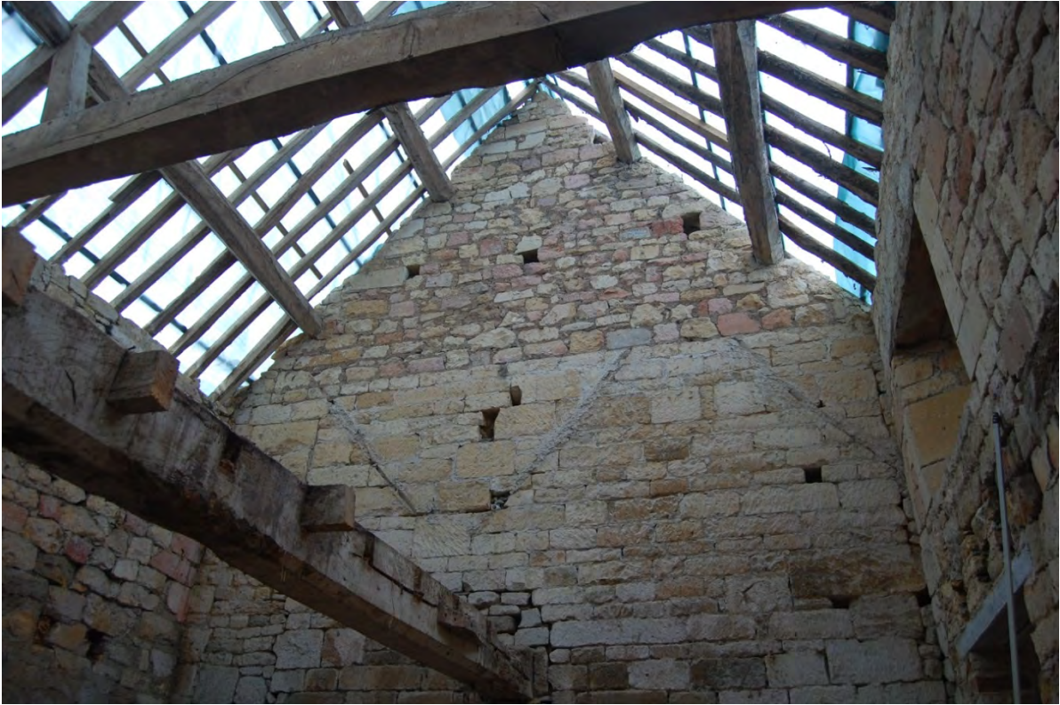
Fig 20: Close up of phase 4 pitched roof wall scars
