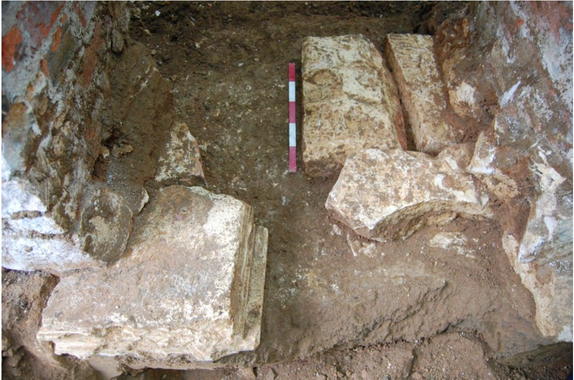
Fig 14: Re-used architectural fragments within the foundations of the dividing wall between Rooms A and B, showing in newly cut doorway
