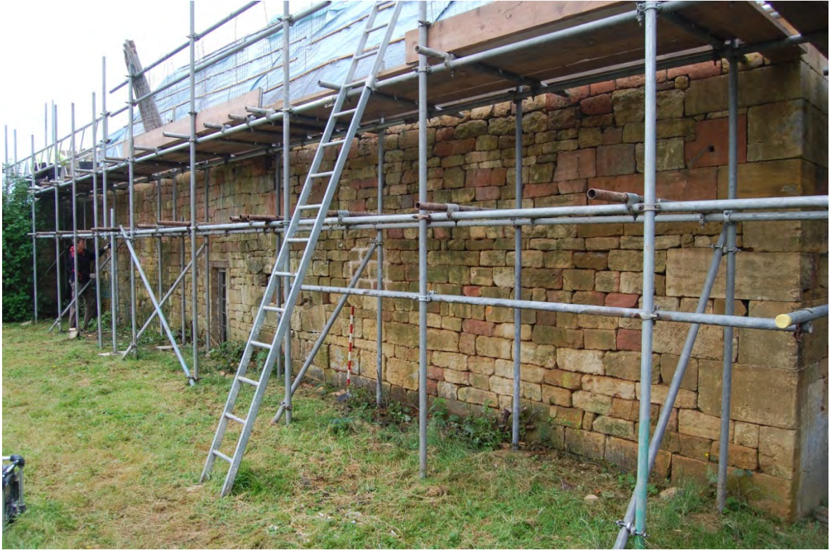
Fig 7: Close up view of the exterior of the east side of the building (looking south). All reddish stone has been burnt
