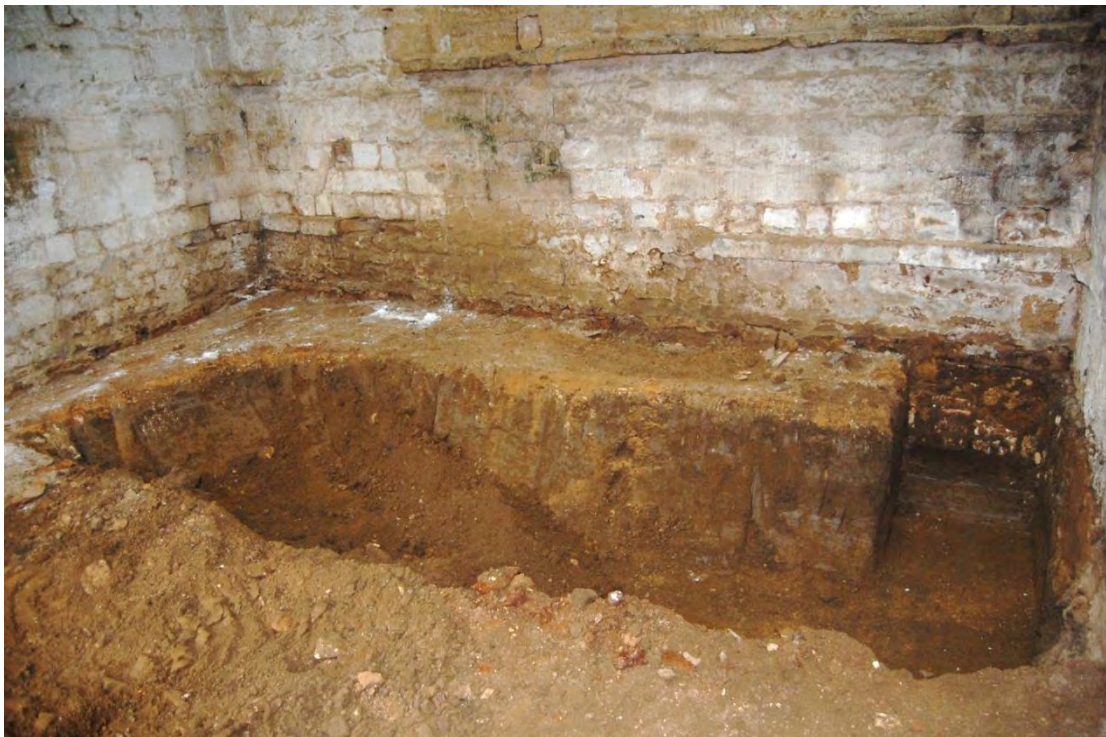
Fig 13: Ground reduction within Room A
