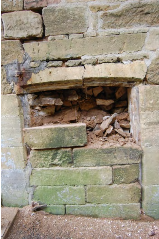
Fig 10: Exterior of blocked doorway in the northern end of room A
