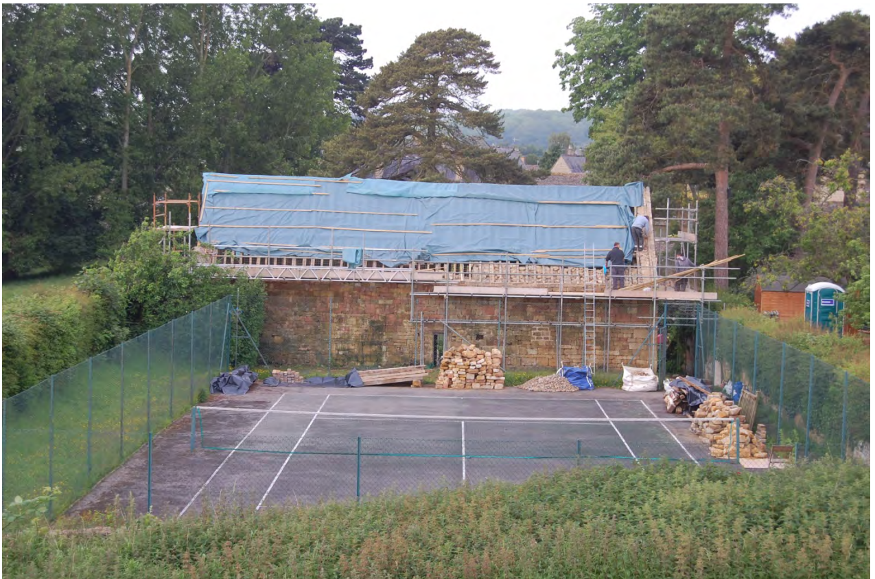
Fig 6: View of the east side of the building from the garden earthworks
