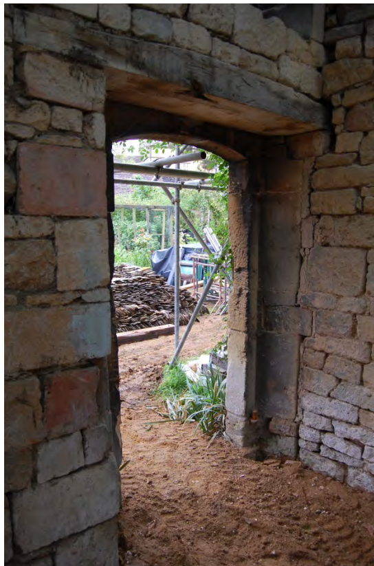
Fig 25: Interior of doorway in north-west corner of room B. Fire-blackening on its inside shows it to have been re-used from a burnt building, probably the main Campden House
