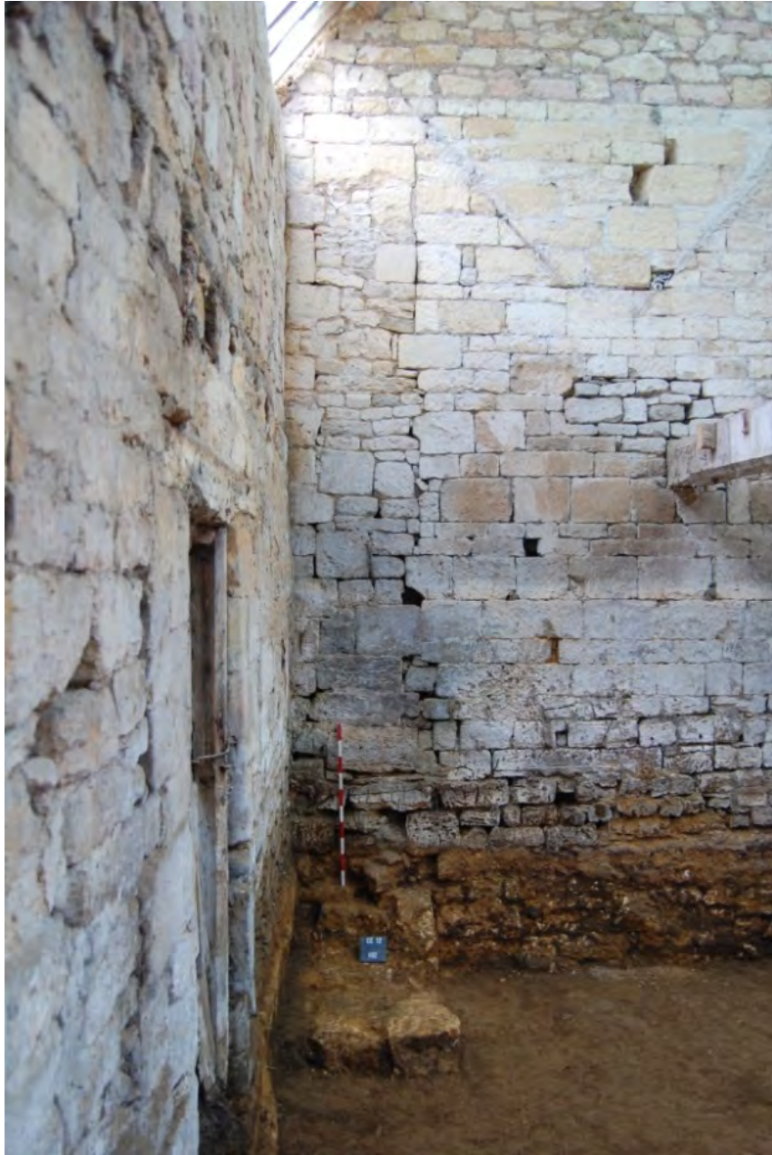
Fig 17: Phase 3 Buttress 102 and vertical wall scar
