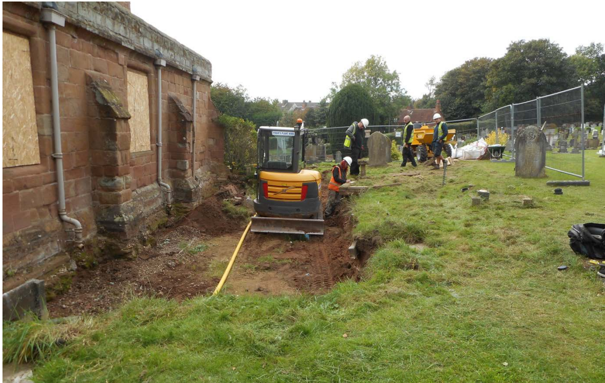
1. Start of groundworks in March 2016, gas pipe exposed
