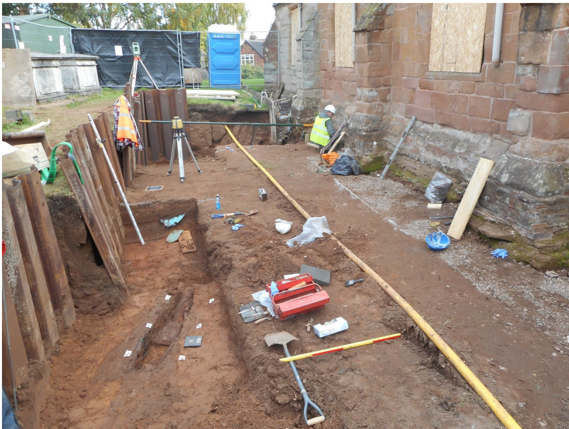
2. Groundworks October 2016 with shored sections
