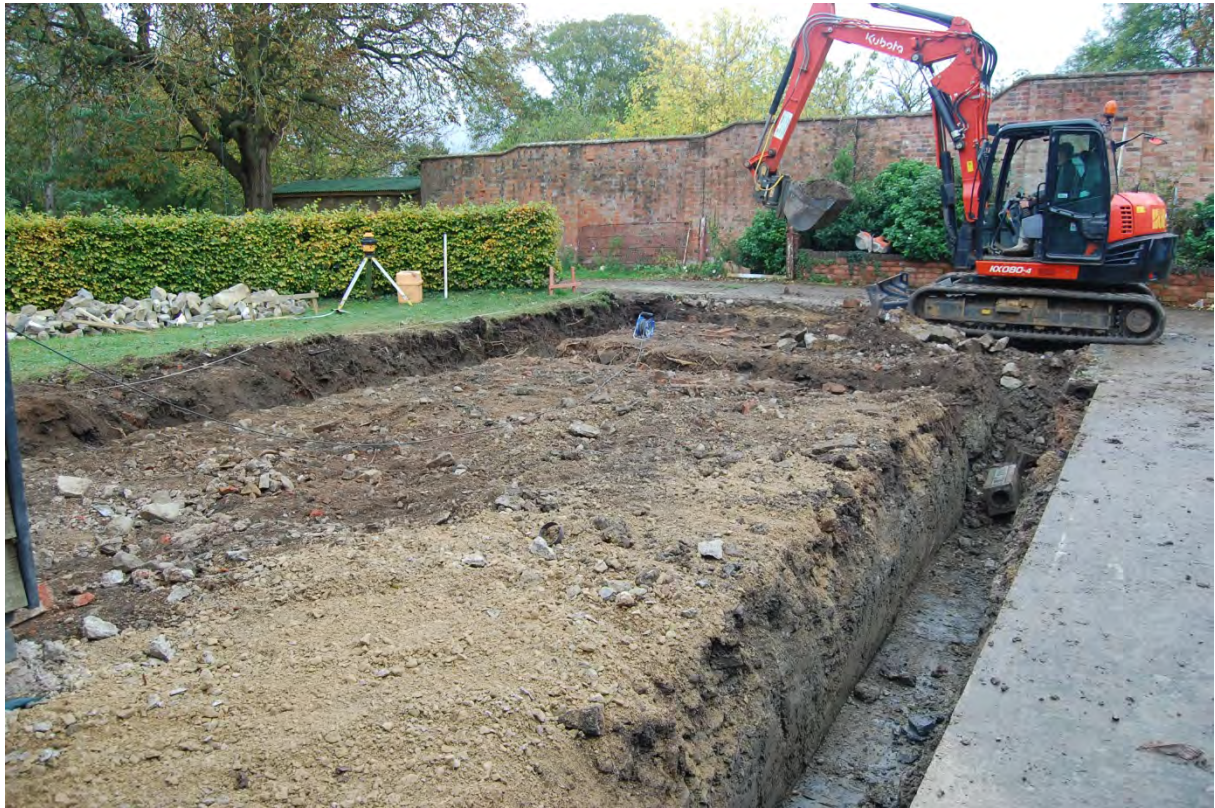
3: Trenches under excavation
