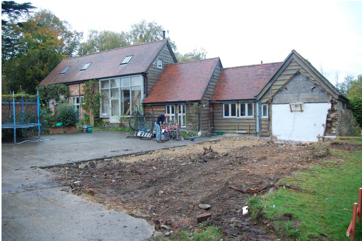
1: Site prior to foundation trenches being excavated
