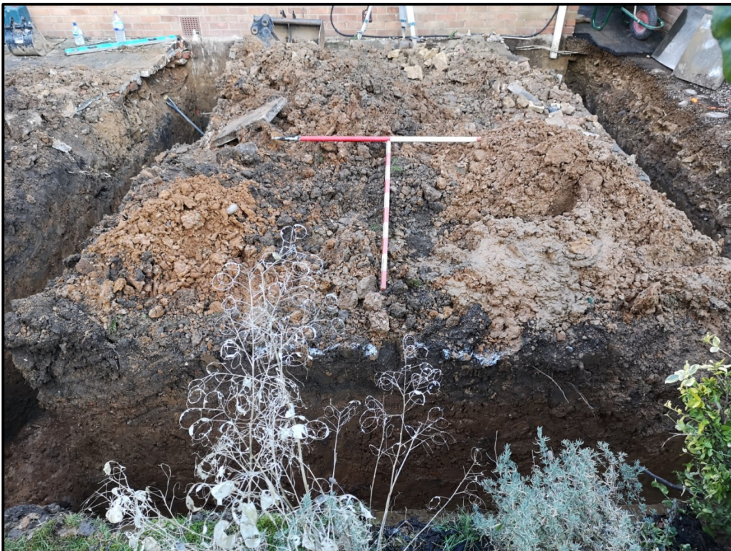
2: North facing view of foundation trenches
