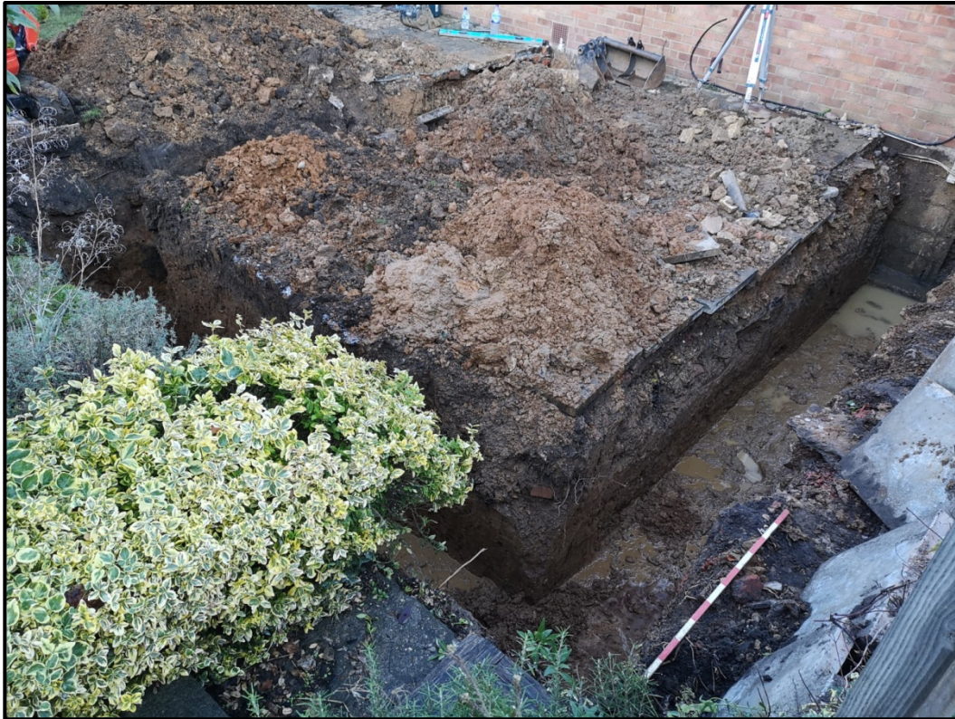
1: Northwest facing view of foundation trenches
