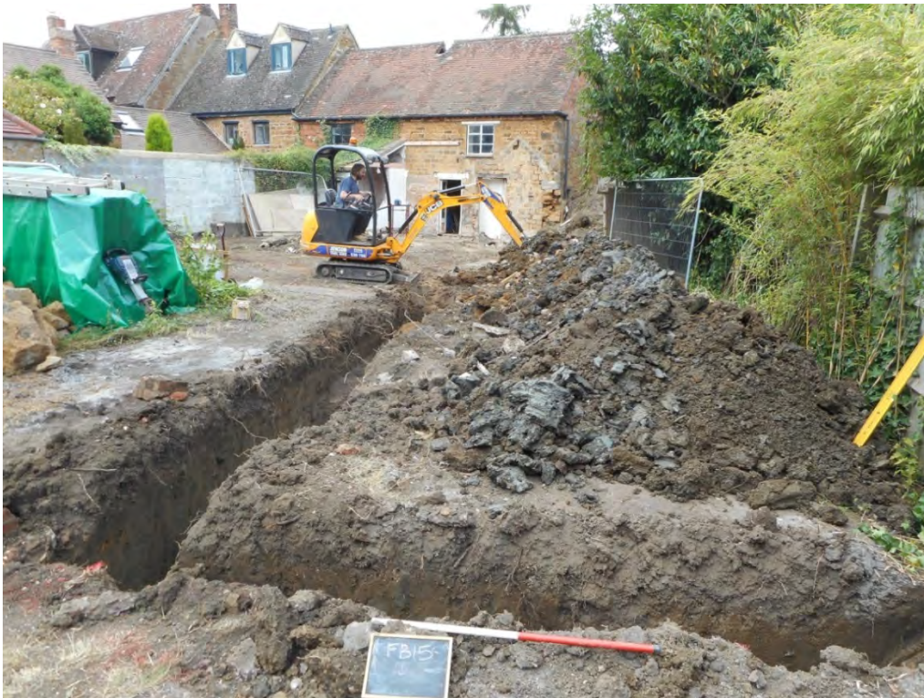
1. Foundation trenches for proposed garage
