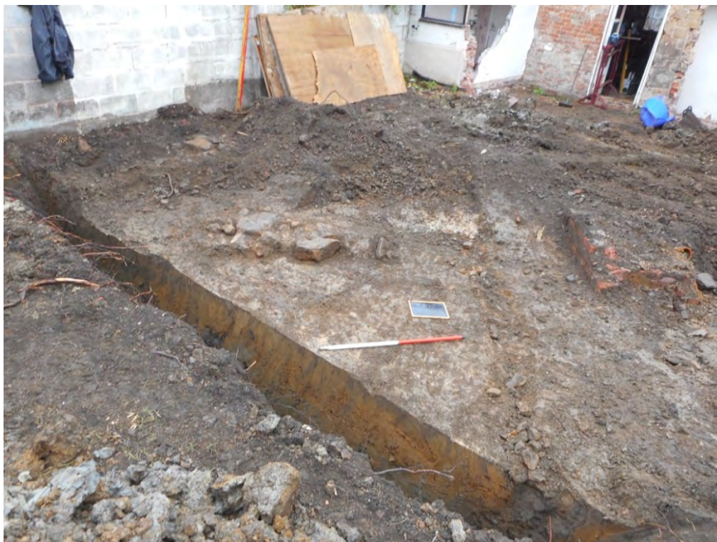
2. Foundation trenches and reduction for proposed extension
