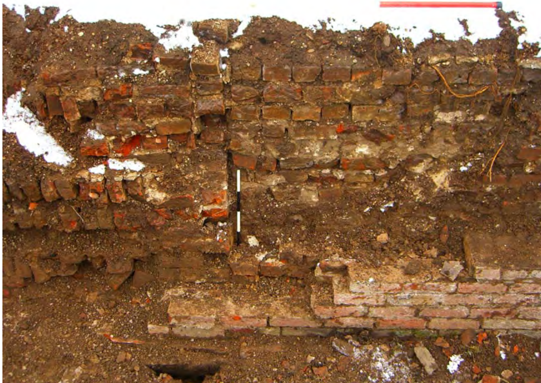
Fig. 5: Detail of construction joint between 102 and 103
