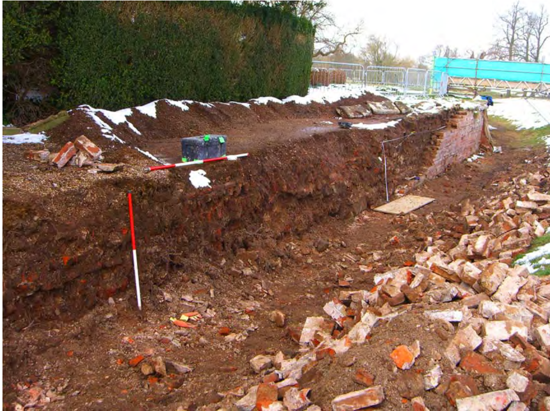
Fig. 4: View of east-facing elevation of ha-ha walls 100, 102-104
