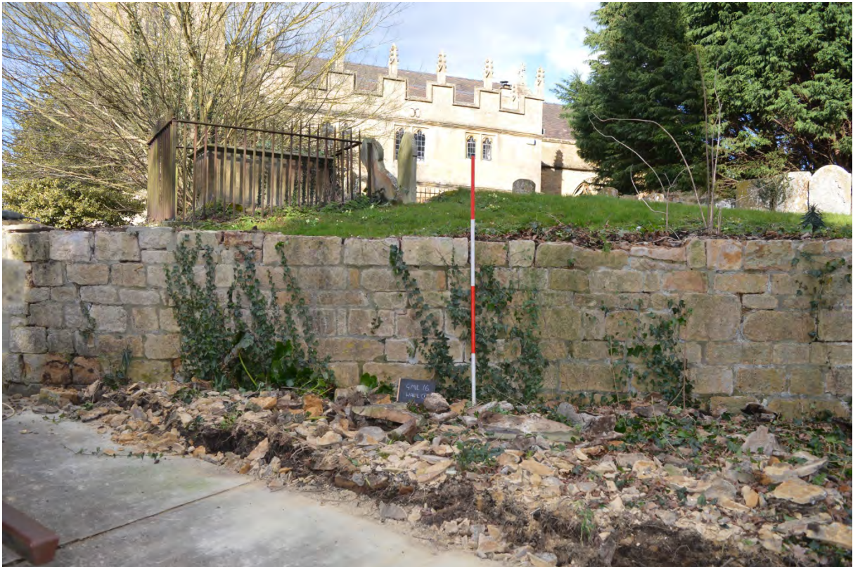
1 Graveyard wall before dismantling
