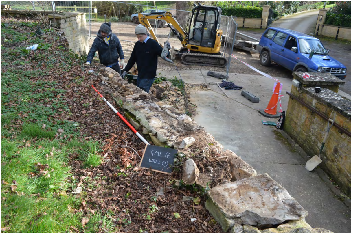
2 Dismantling in progress
