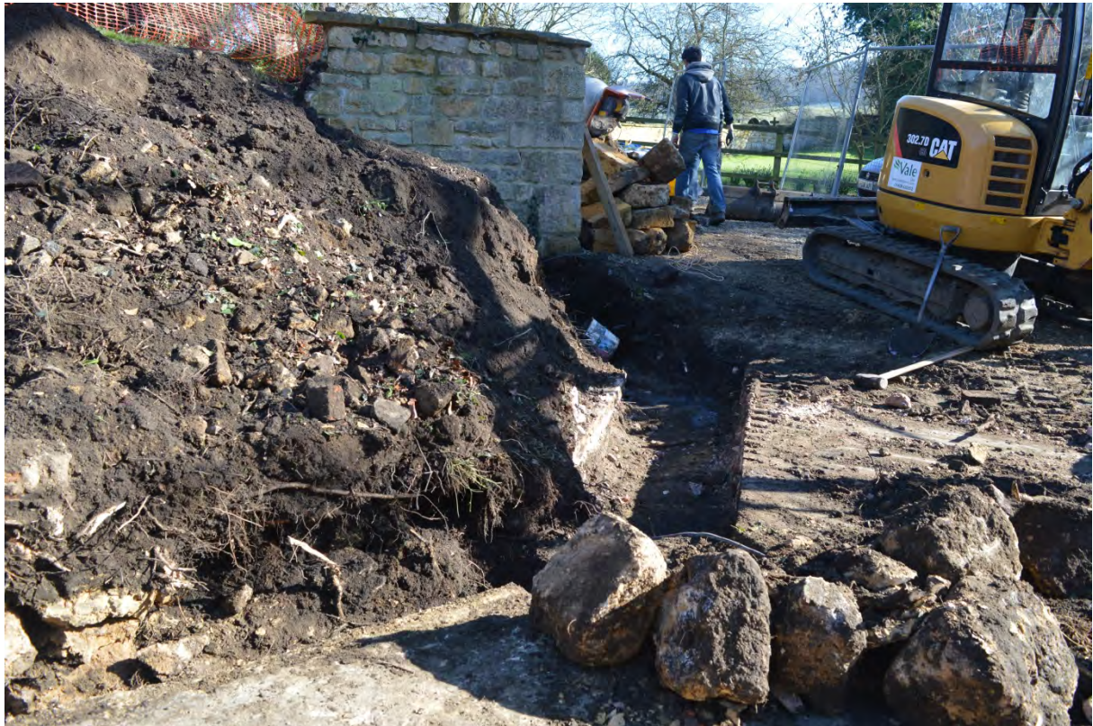
5 Excavation of footings for new wall
