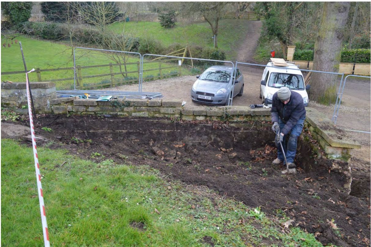
4 Grading of soil to rear of walls 4 and 5
