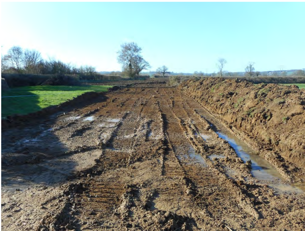
4. Western strip area, northern end, looking south
