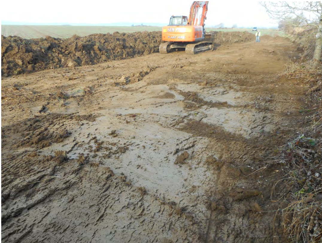
1. Stripping in area by railway embankment, looking north
