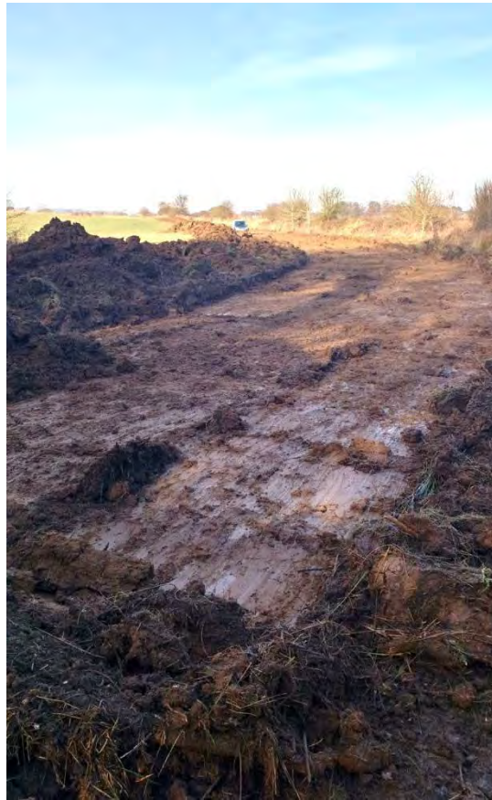
3. Stripped area at south end of embankment, looking north
