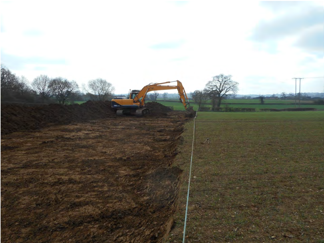
7. Southern end of western strip, looking south
