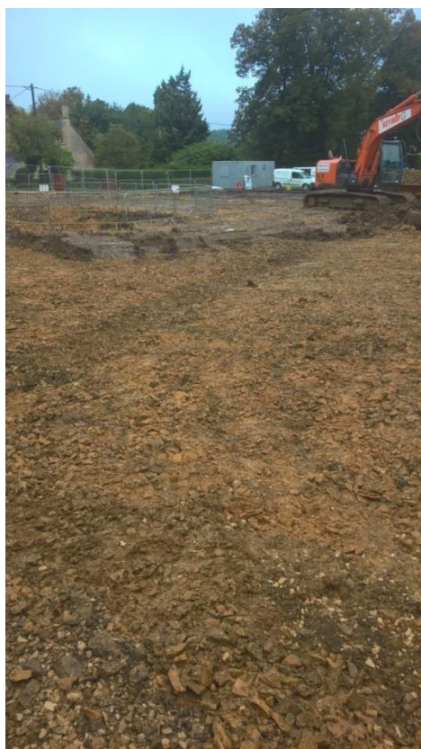
8. Enclosure ditch 20 with return in foreground
