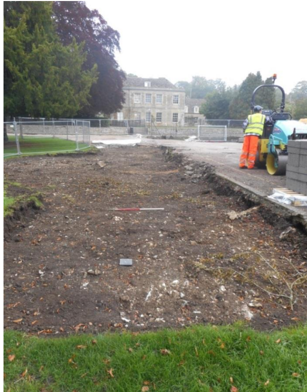
1. Area 1 topsoil stripping
