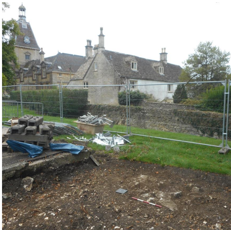
2. Area 1 - Wall foundation 3
