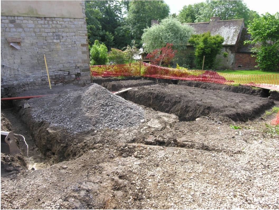
Fig 4: Foundation trenches, looking east
