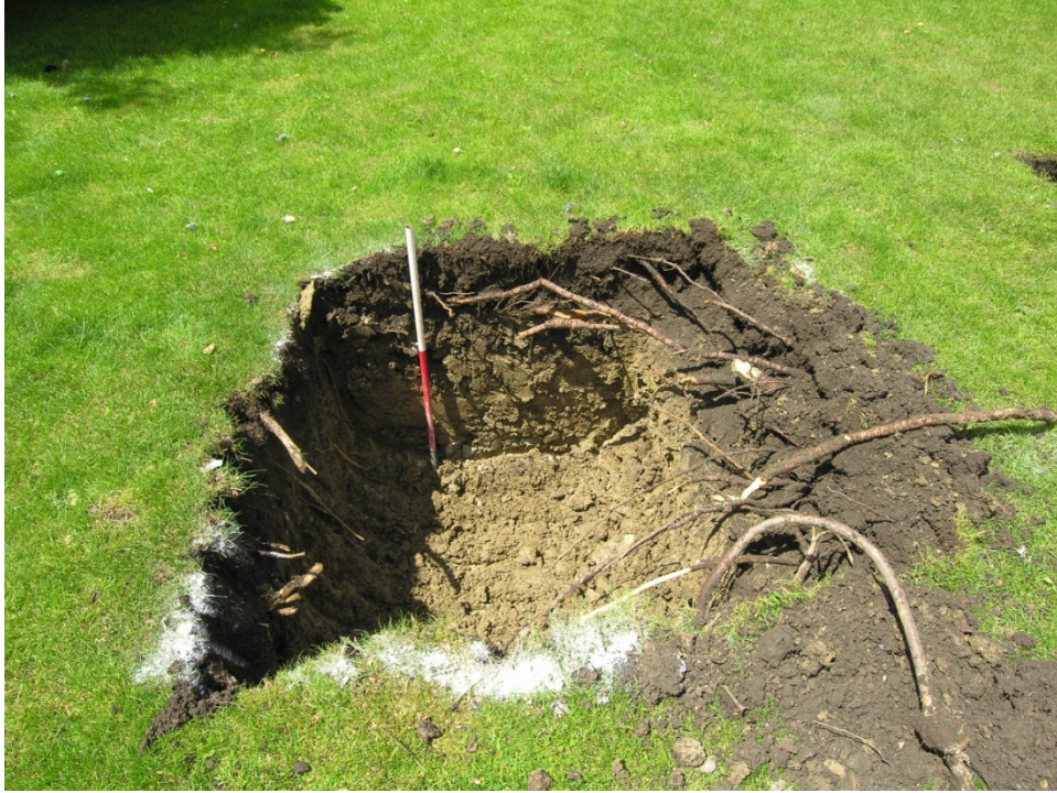
Fig 6: Soakaway, looking west
