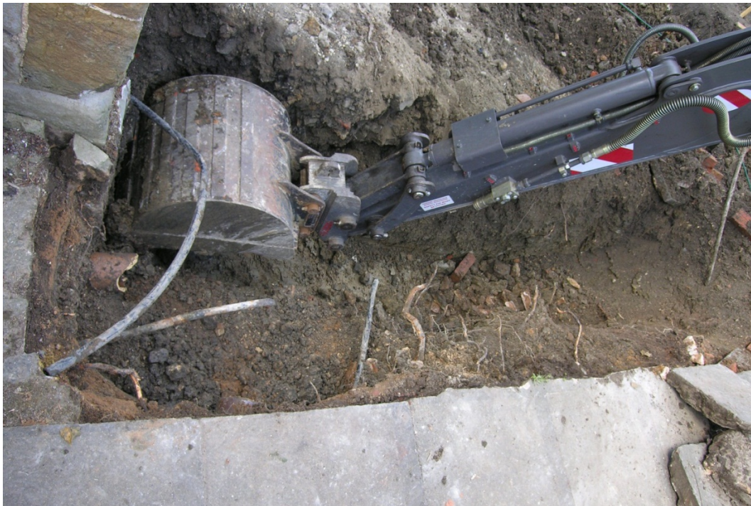
Fig 5: Manhole excavations
