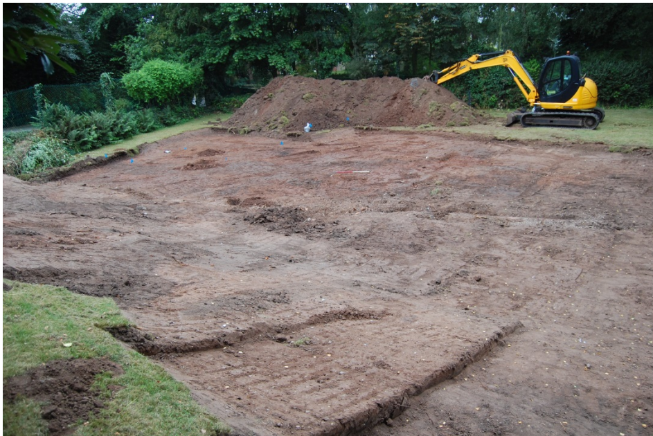
1. Excavation area, (1001) and (1003)
