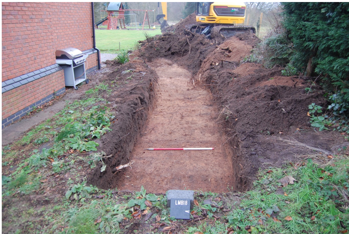
1: Trench 1, looking east
