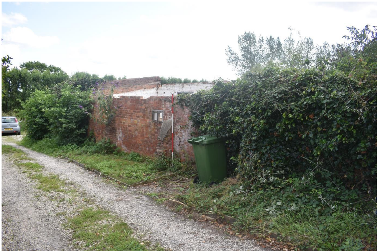
2: The north-east elevation of Building 1
