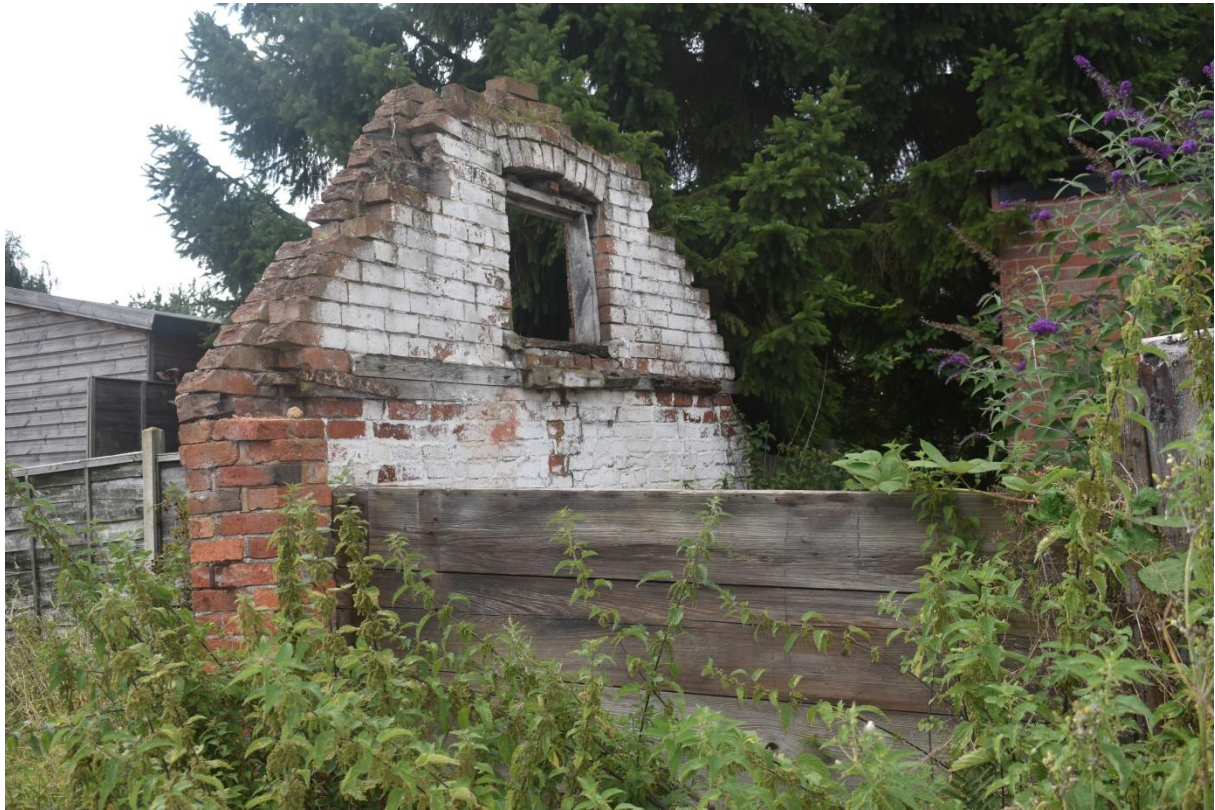
13: Wooden boards used to infill SW bay of Building 2
