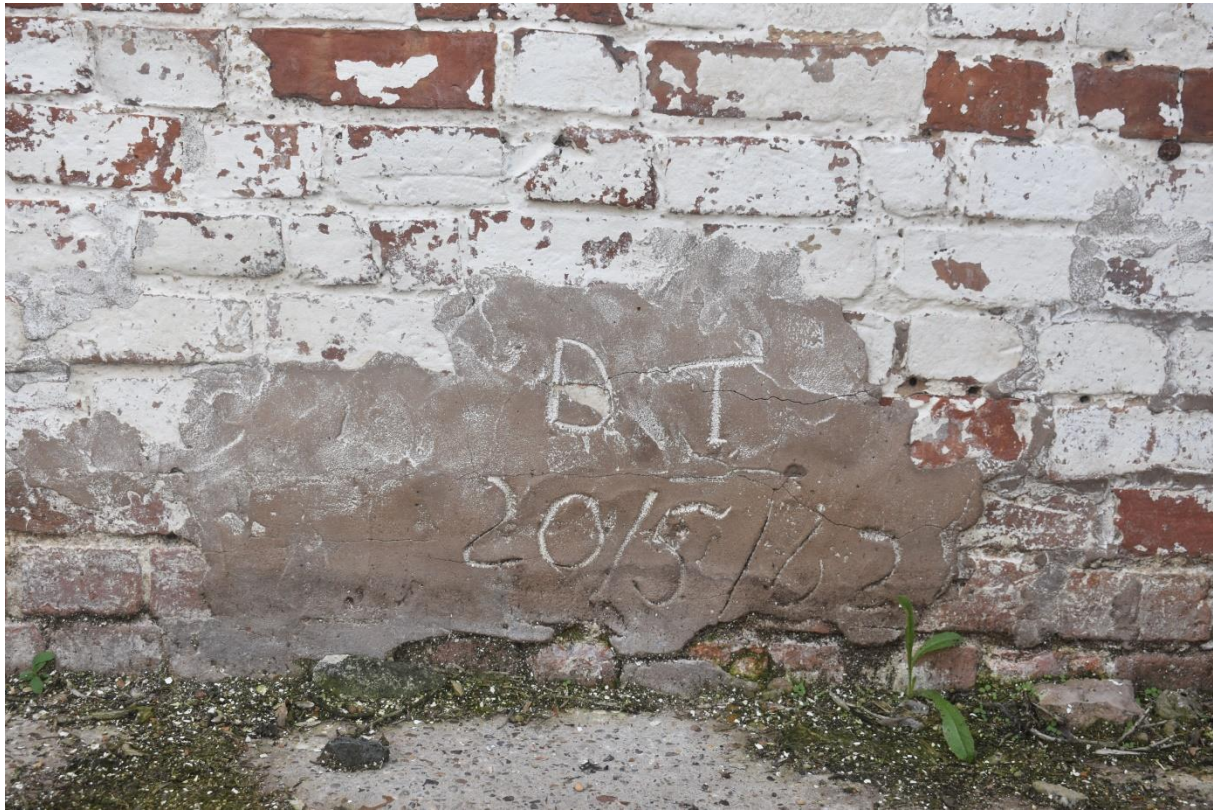
9: DT 20/5/62 on mortar
