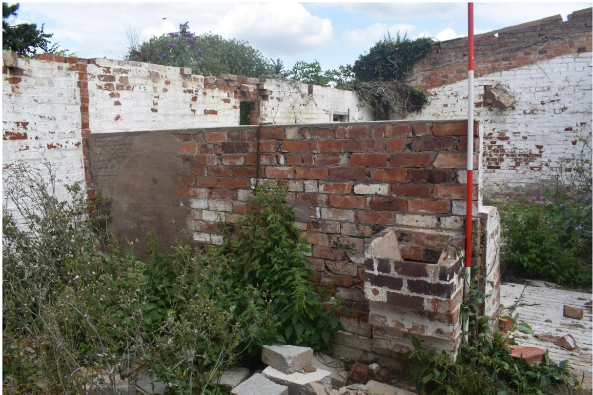
8: Rear of wall with brick feed chute
