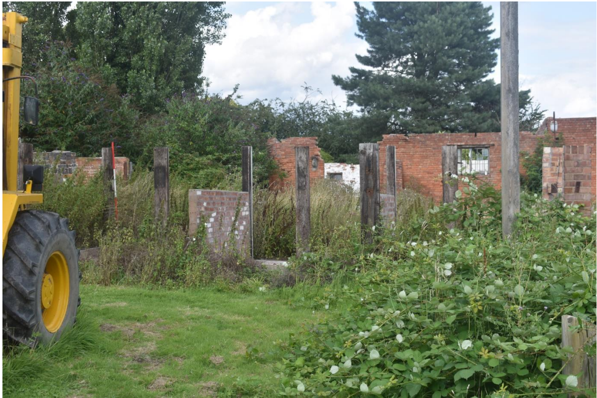
15: Railway sleeper posts of Building 3
