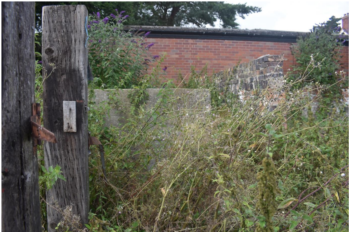
14: Concrete infill and blue brick cross-wall within Building 2
