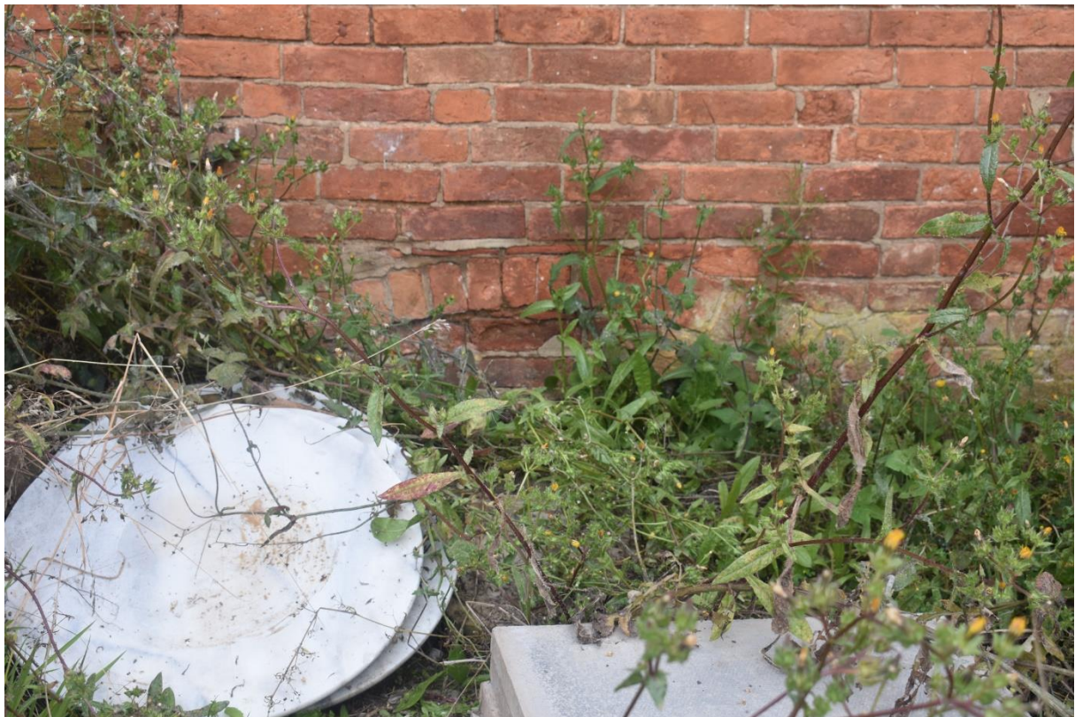
6: Relieving arch on SW wall
