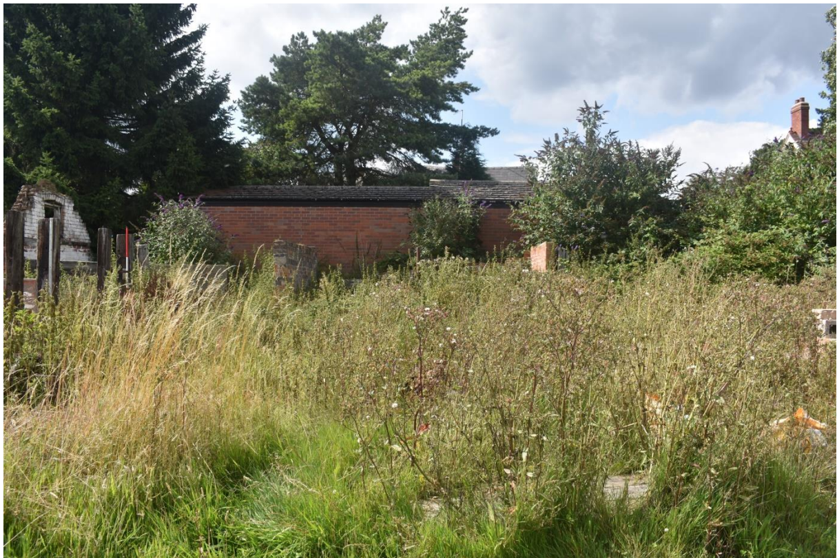
12: Front of Building 2, obscured by vegetation
