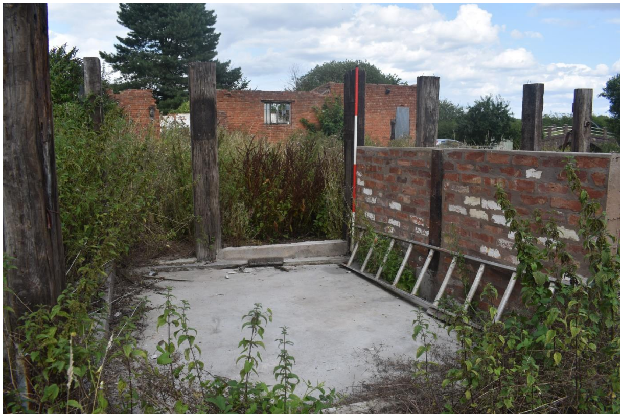
16: Concrete floor and brick cross-wall in Building 3
