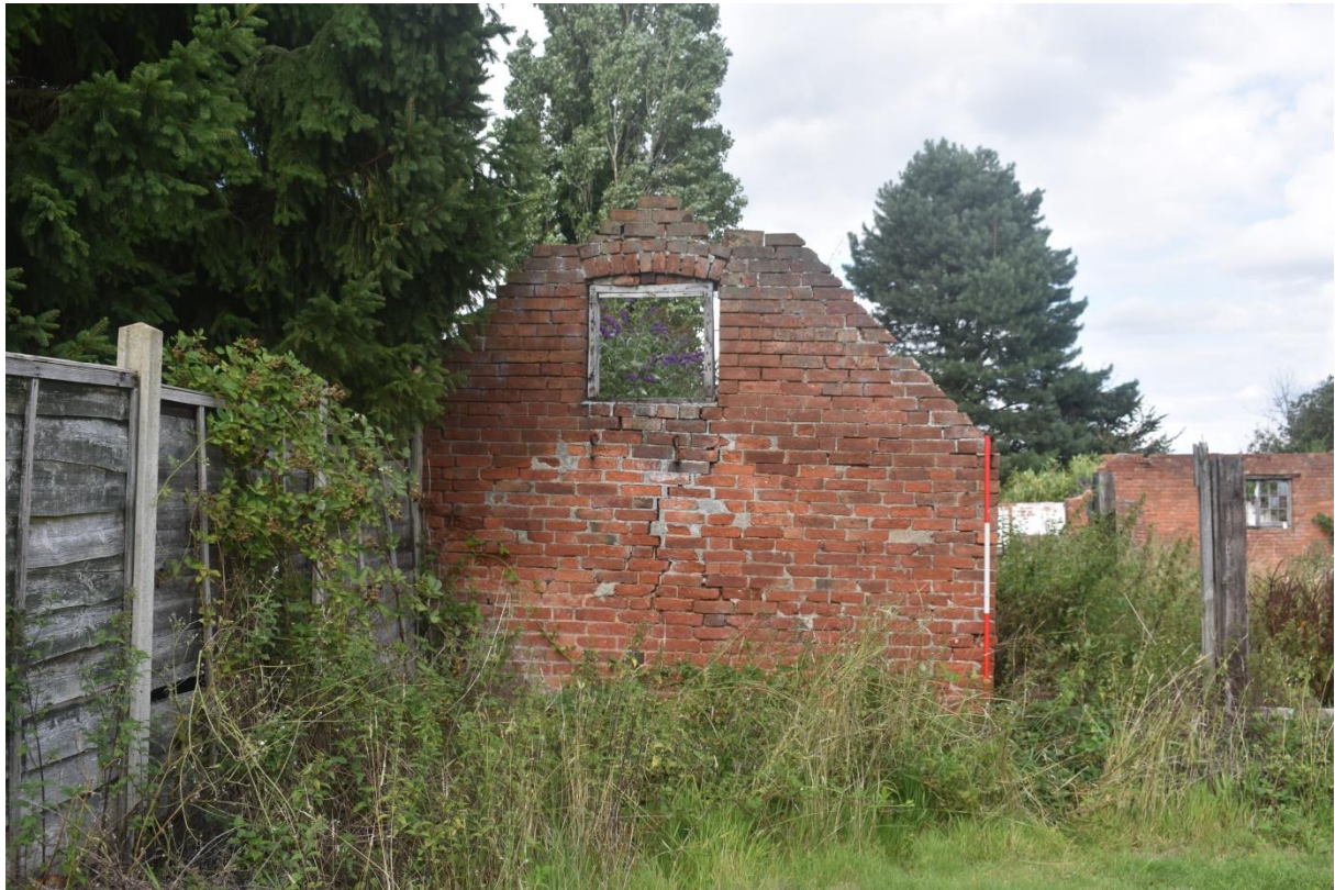
11: Gable of building 2
