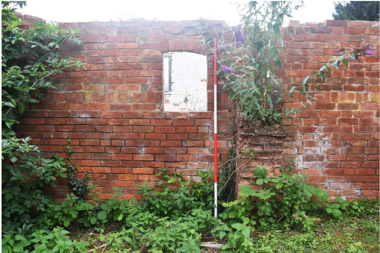
3: Original window and later buttress on NW side of Building 1
