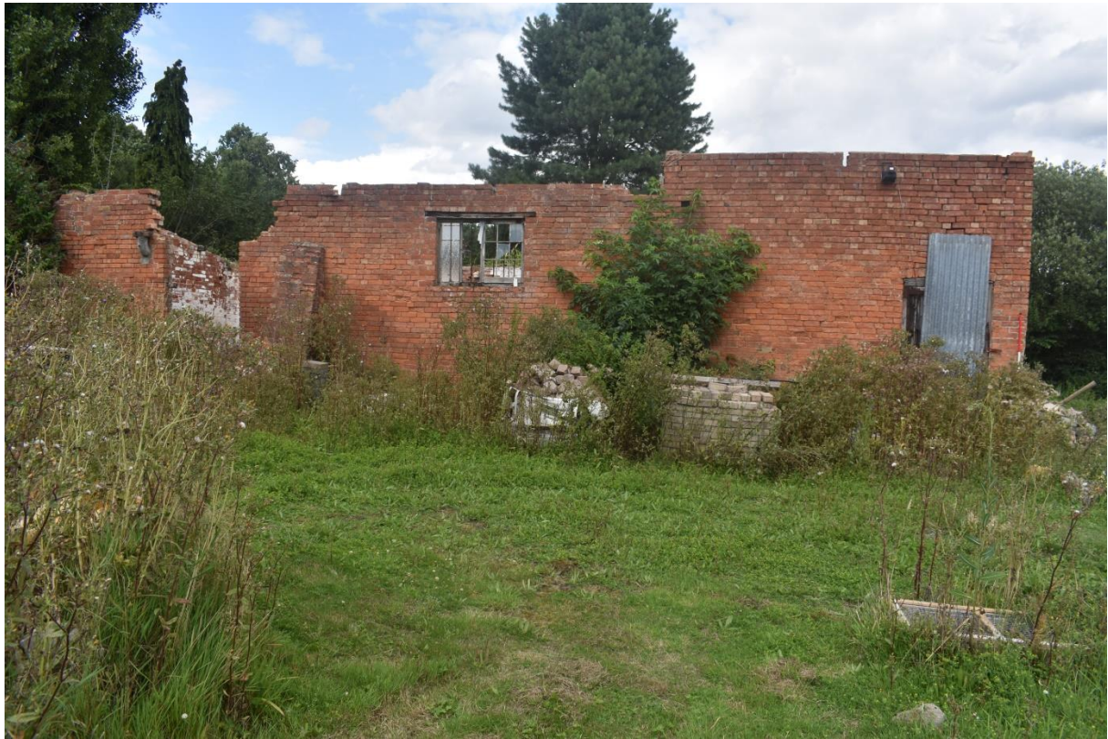
5: Building 1, SW elevation
