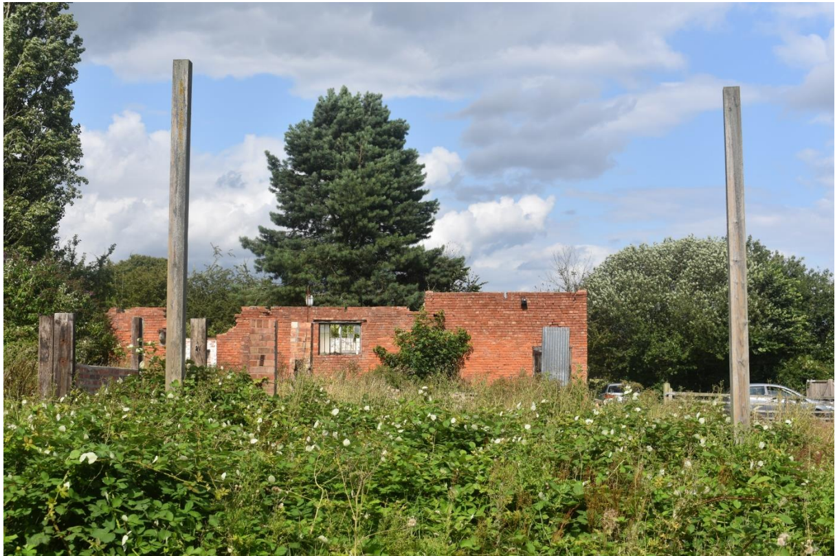
17: Two poles of the pole barn, with Building 1 beyond
