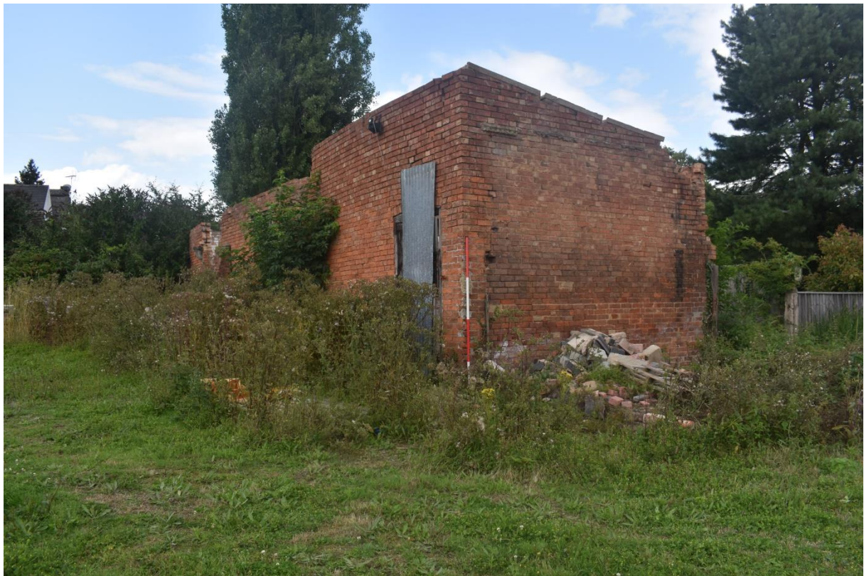
4: Building 1, looking north
