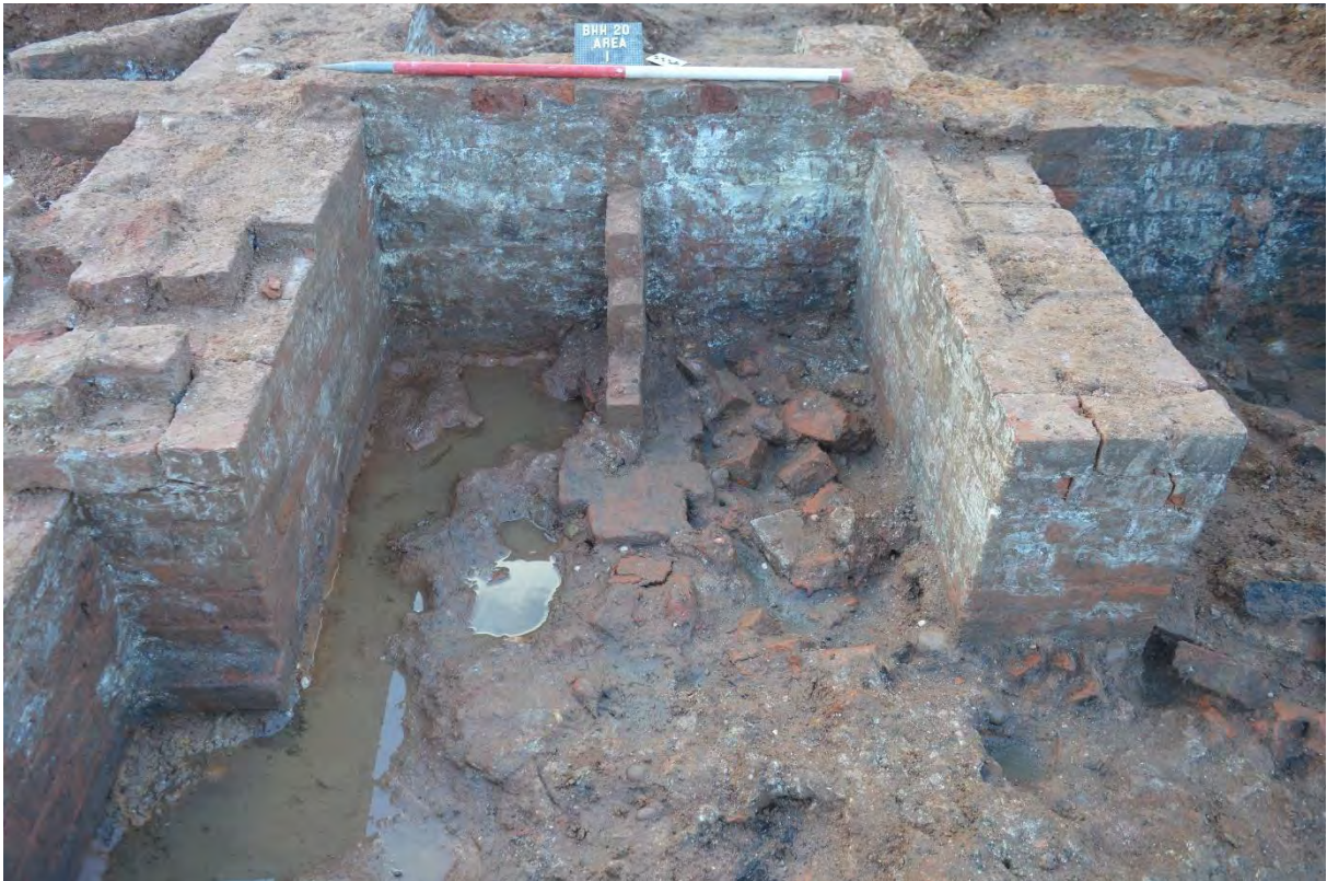
5: Support wall standing on extant remnant of brick floor between walls 36 and 74
