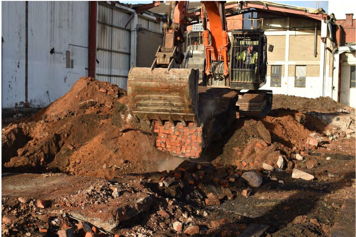
15: Modern brick footing being removed on western part of area
