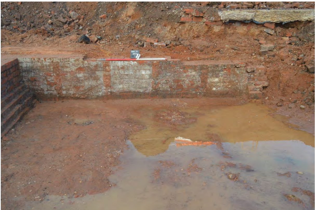
6: North wall of cellar with scars of brick support walls
