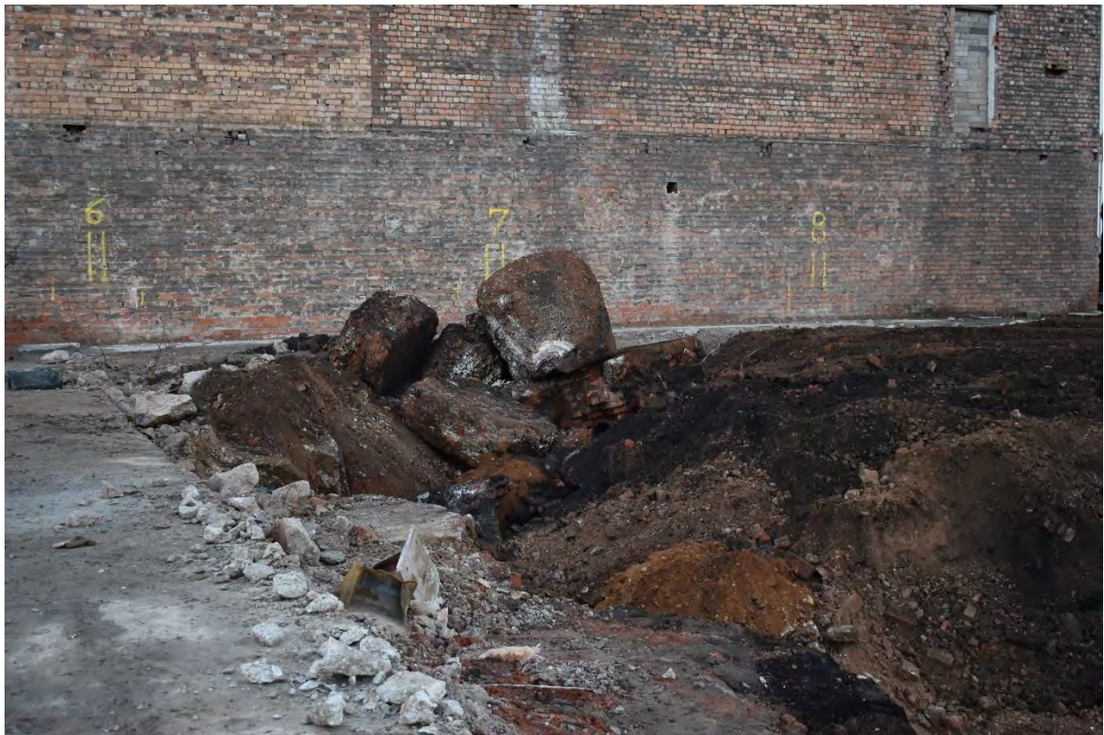
16: Massive concrete footings of modern factory
