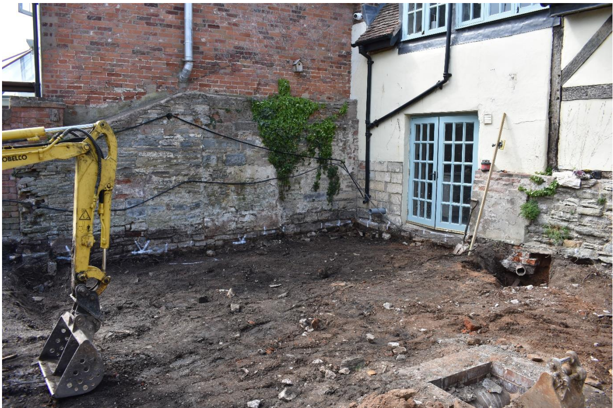
4: Wall 7 facing WNW
