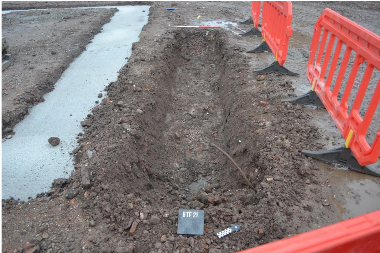
4: Foundation trench for Plot 17 looking north-west
