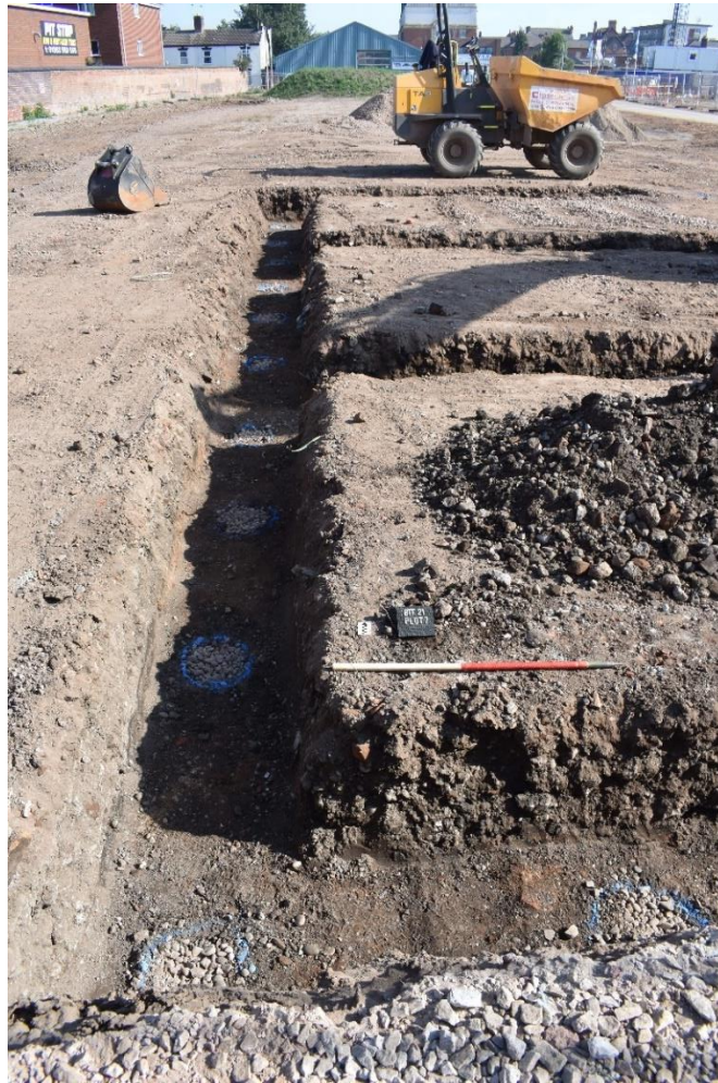
3: Groundworks in Plot 7 looking north
