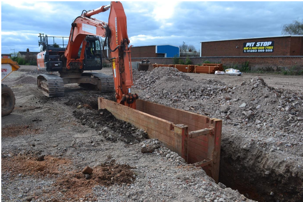
1: Excavation of drainage trench using steel trench box
