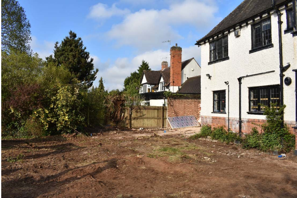
1: The site prior to digging
