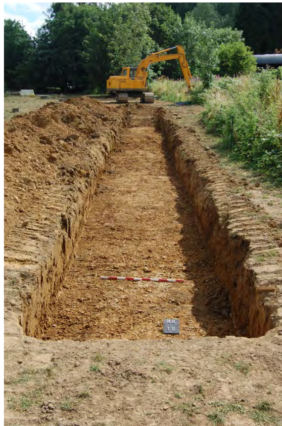
Fig 12: Re-examination and cleaning of Trench 12
