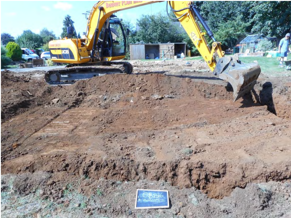
1 Ground reduction of internal footprint
