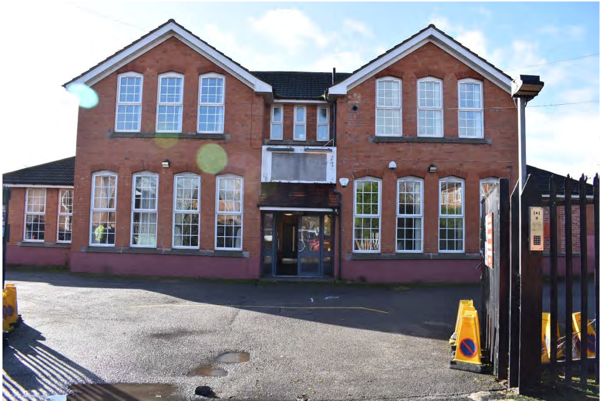
5: Main TA building looking south-west
