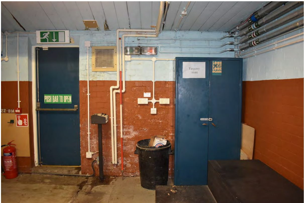
16: Control panel, exit and storage in shooting range, looking north-west
