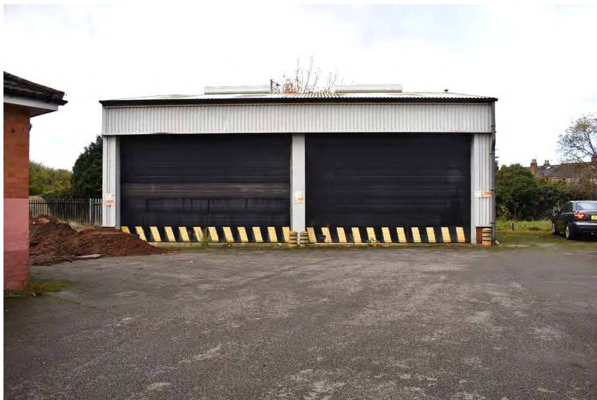
24: Building C garage looking west
