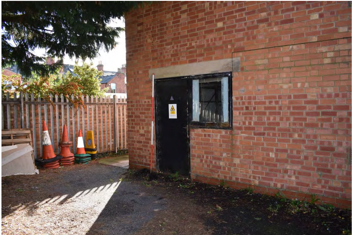
23: Building B, ground-floor offices, restricted area, looking south
