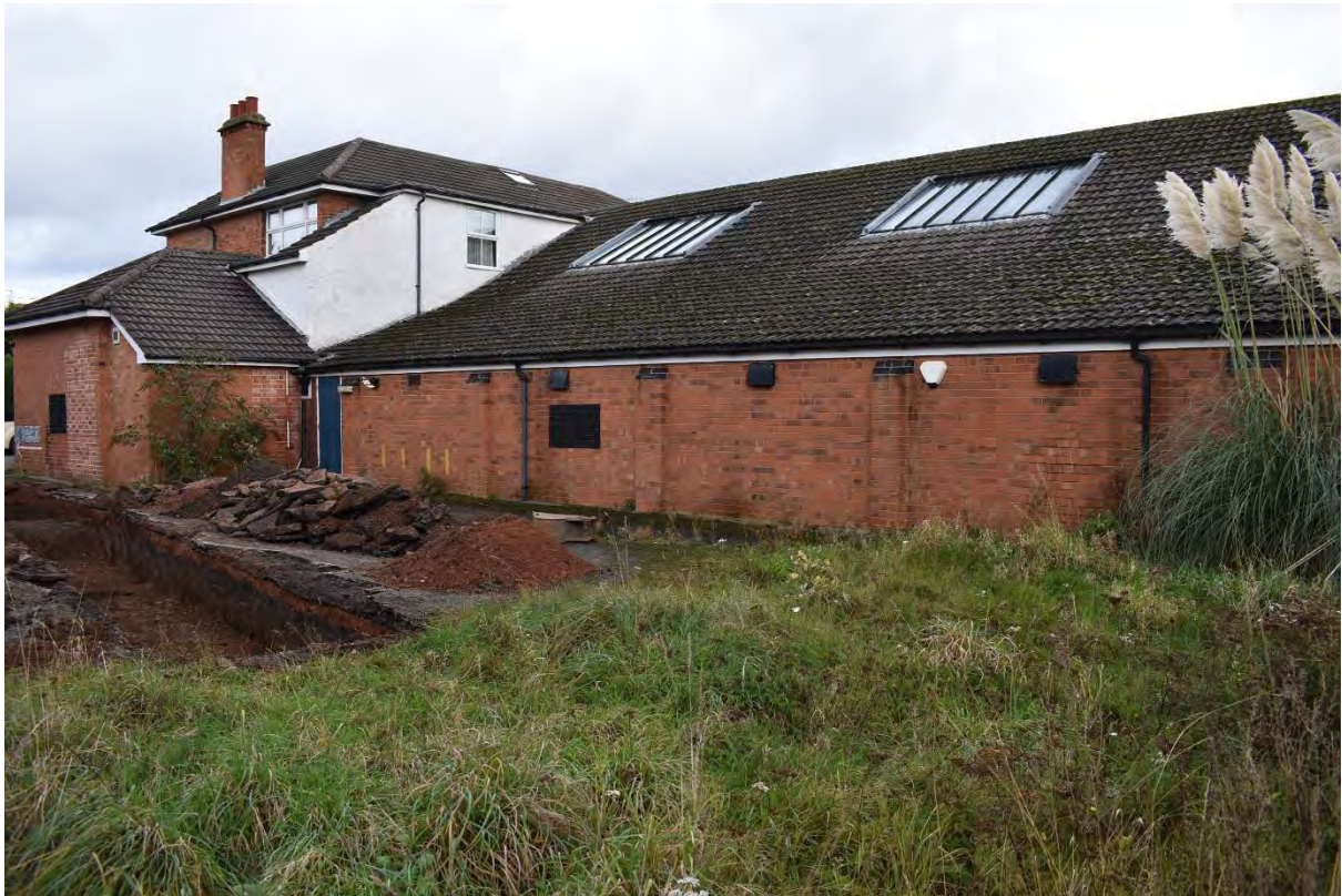
7: Drill hall, shooting range side of building, looking east
