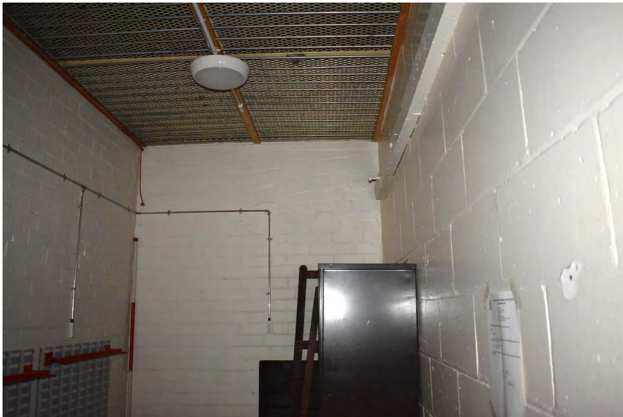
12: Rear of the armoury looking south-west, note high-level segmental brick arch in rear wall
