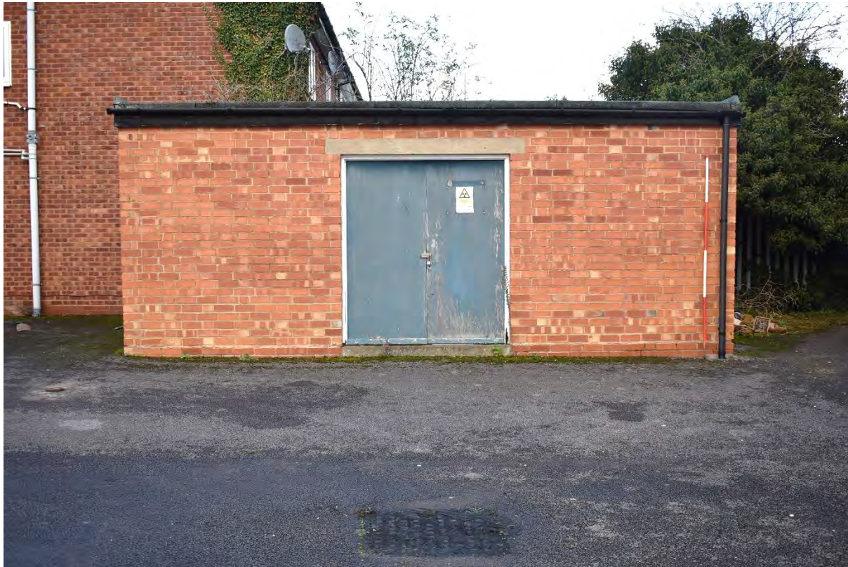
27: Building E, stores outbuilding, looking north-east
