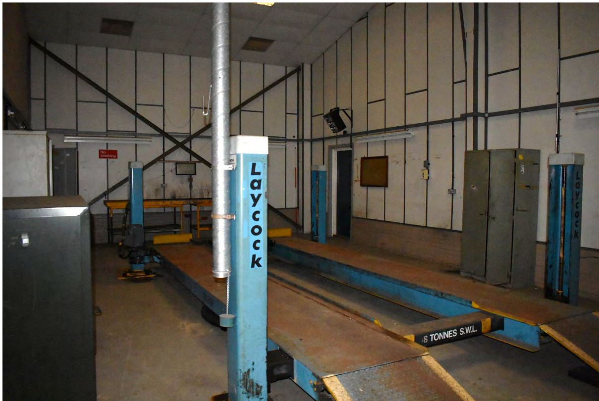
25: Room 2 of the garage with maintenance ramp, looking north-west
