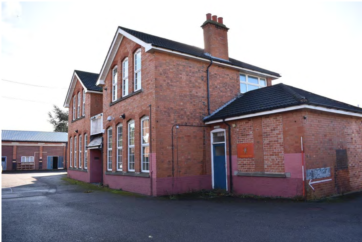
6: Oblique view of TA building looking south
