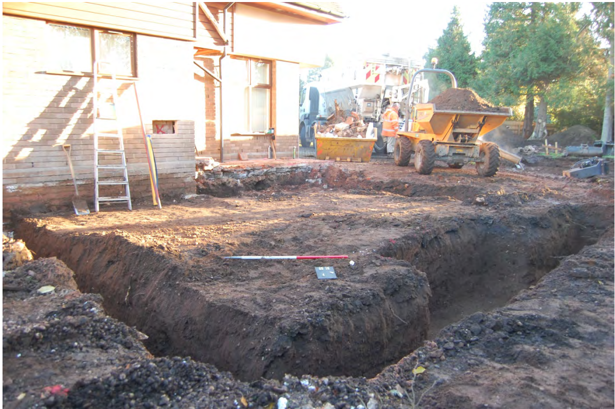
4. General view of extension trenches
