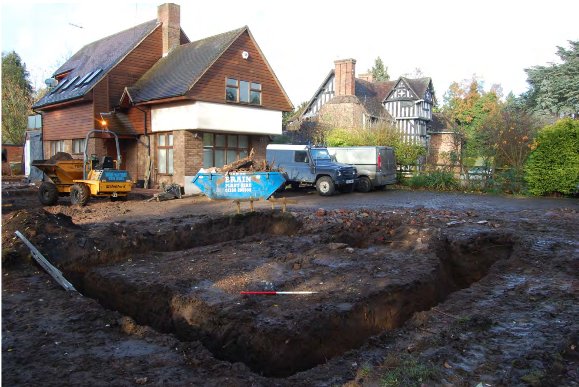
3. General view of house and garage foundation trenches
