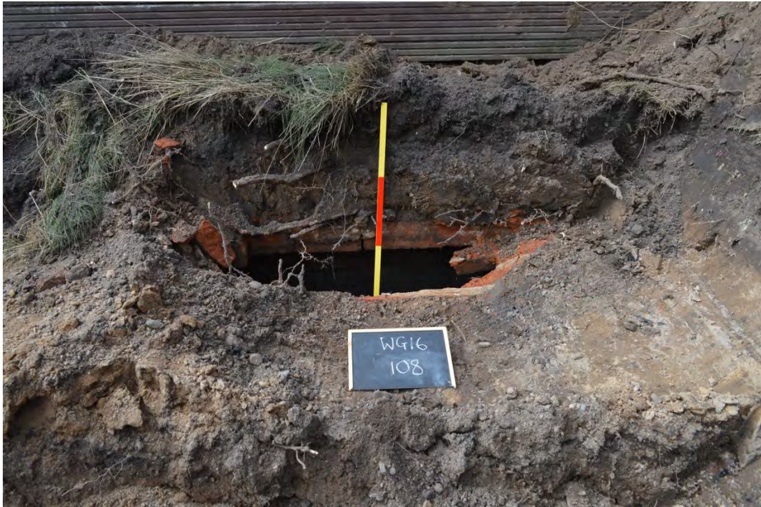
3. Culvert when found
