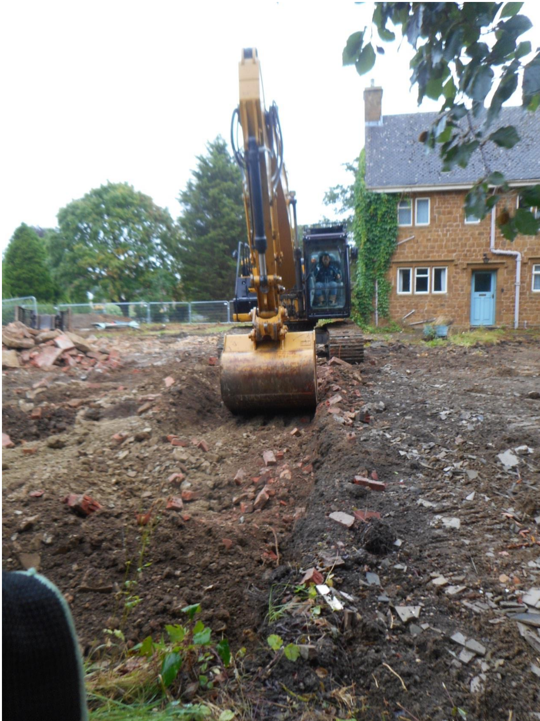
1. Removal of footings of garage and outbuilding
