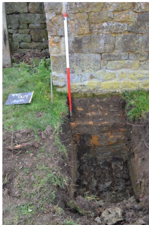
4: Geotechnical pit 1 looking south, showing wall foundation 11
