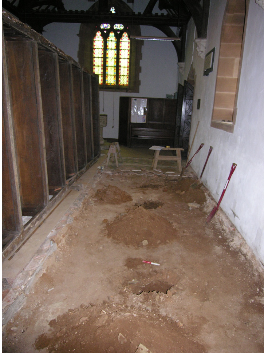
Fig 2: View of area of investigation with excavation of pits
