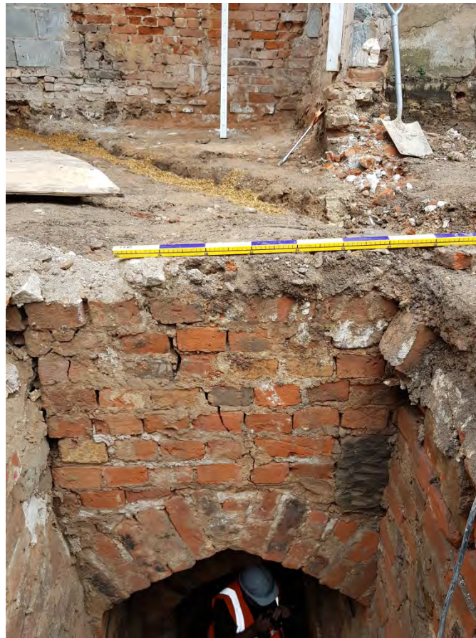
7: Brickwork of access shaft 29
