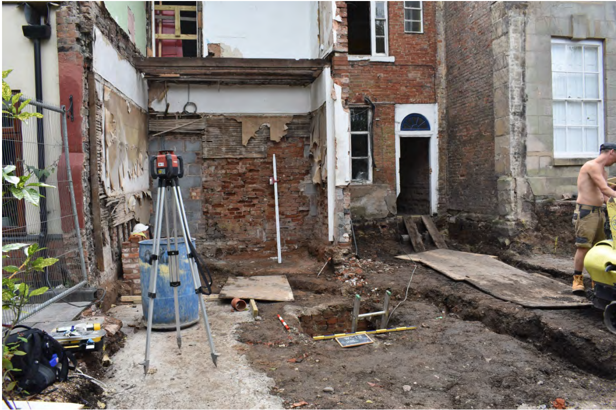
3: Rear of the property and demolished wall 4, looking south-west
