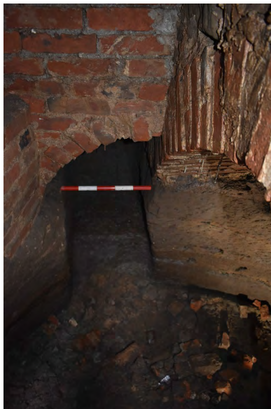
10: Fill inside structure 32 with brick arches
