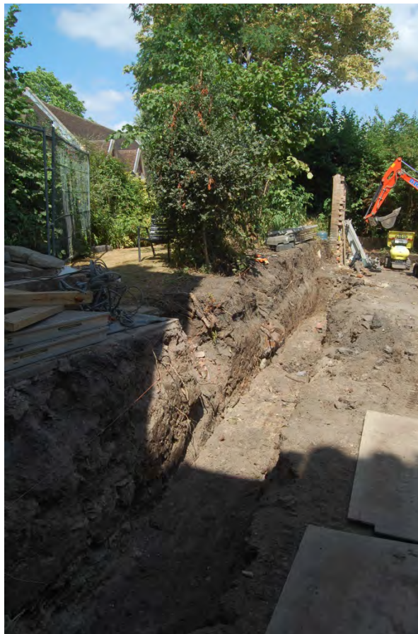
4: East footing, looking north-east
