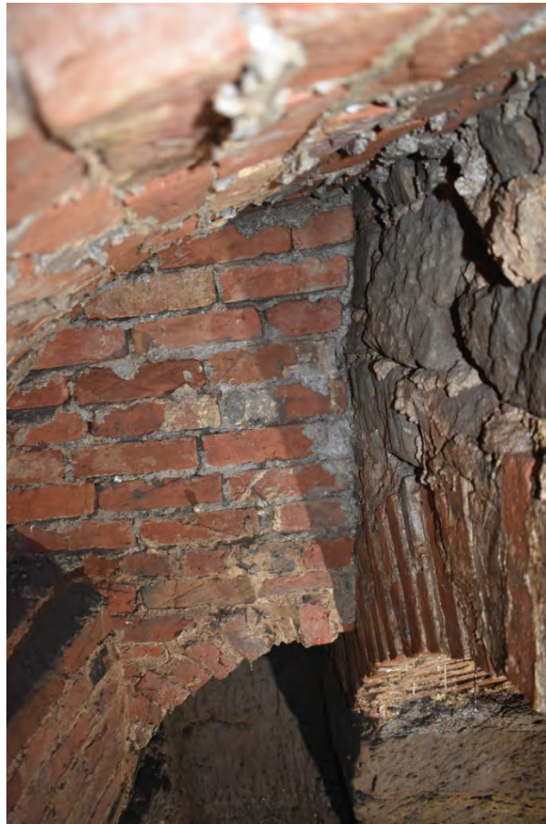
9: Brickwork inside structure 32
