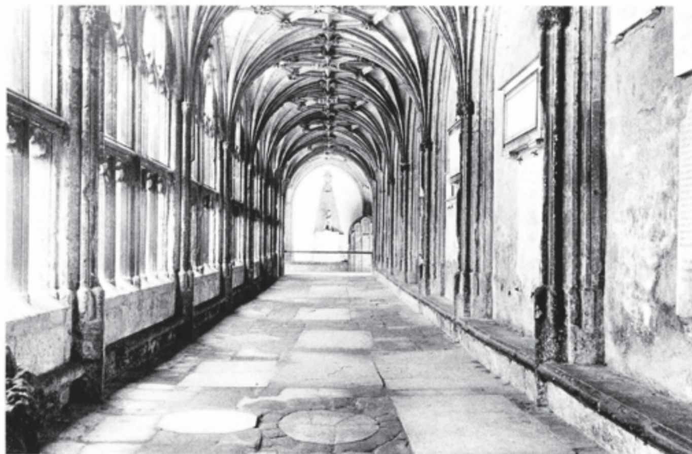
Fig. 273 South cloister walk, looking east, showing the medieval paving and later grave slabs. Note how the late medieval screen wall (left) is built on top of the earlier bench, which has a projecting roll-moulding. Taken by Thomas Phillips, around the turn of the twentieth century (Dean and Chapter of Wells)
