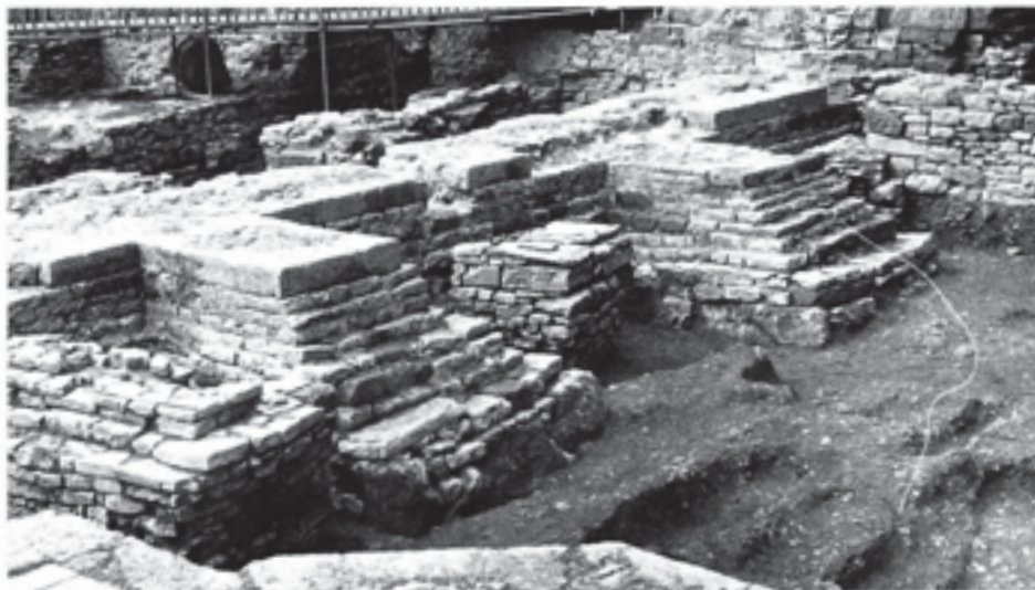
Fig. 208 Stillington's chapel. North wall of the nave, showing the stepped foundations of buttresses F337a and F337b. In between, are the remains of two buttresses belonging to the earlier Lady Chapel. Scale of 75 cm
