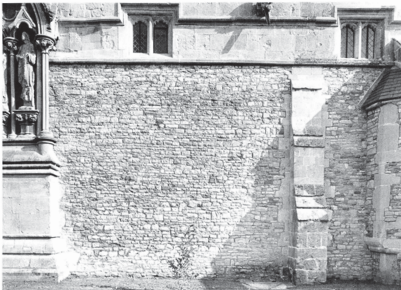
Fig. 342 The northernmost bay ( W 1 ) of the west cloister and the first buttress, showing the relationship to the west front of the cathedral. Note that the cloister plinths are now below ground level. The porch stair-turret (Structure 25A) is seen on the far right
