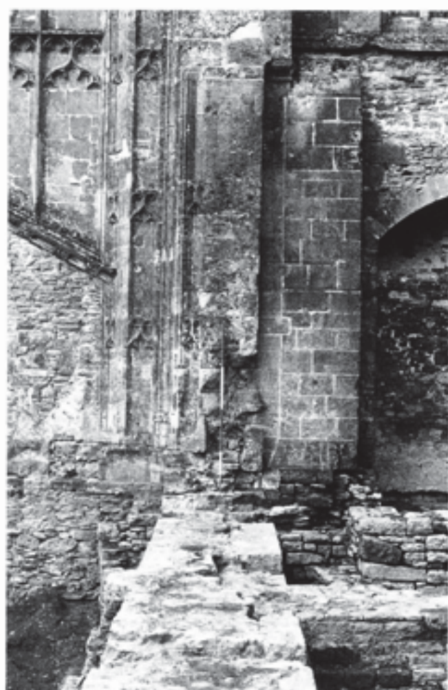
Fig. 234 View west along the north wall of Stillington's chapel where it abuts the cloister. Above the 2 m ranging-pole is the splay of the westernmost window of the chapel. Between the wall and the arched entrance to the Holy Cross chapel (right) is one of the early Gothic cloister buttresses (E67)
