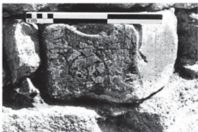
Fig. 151 Section of an octagonal column, perhaps from the north arcade of the Lady Chapel, reused in the foundations of Stillington's chapel. Note the limewashing and graffiti (cf. Fig. 141E)
