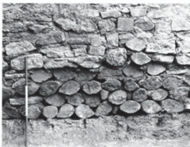
Fig. 373 Sections of discarded medieval screen mullions used in the foundations of the Victorian masons' yard wall. Scale of 75 cm
