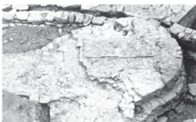
Fig. 218 Stillington's chapel. Stepped circular foundation for the south-west stair-turret. View south, with the pipe-duct and conduit beyond. Scale of 2 m
