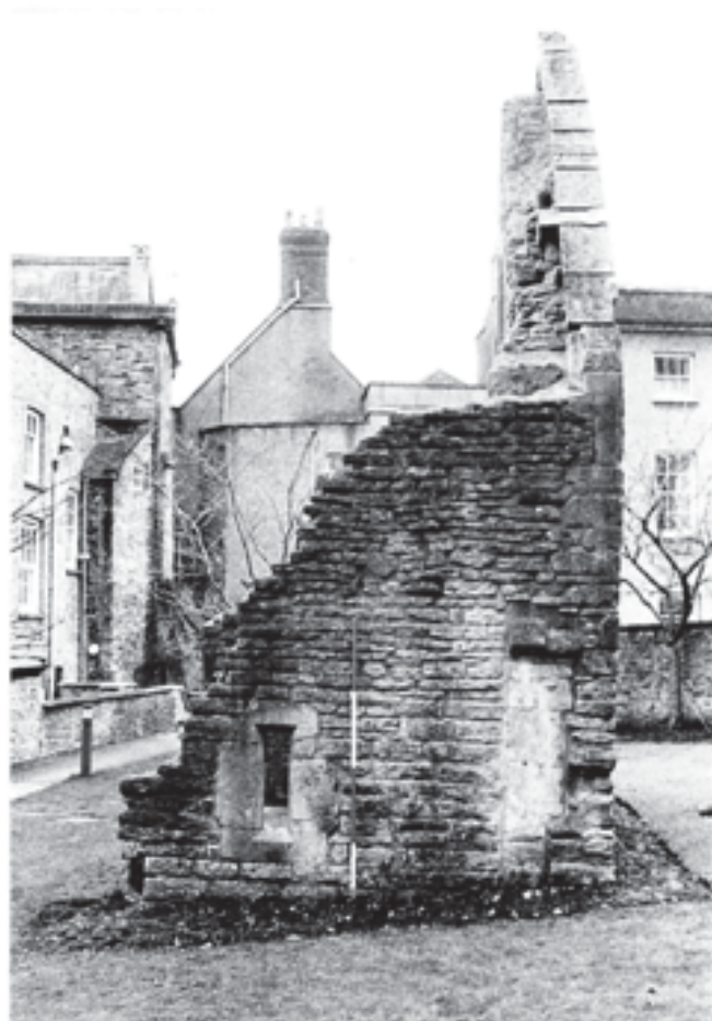
Fig. 351 Fragment of the east wall of the choristers' house
