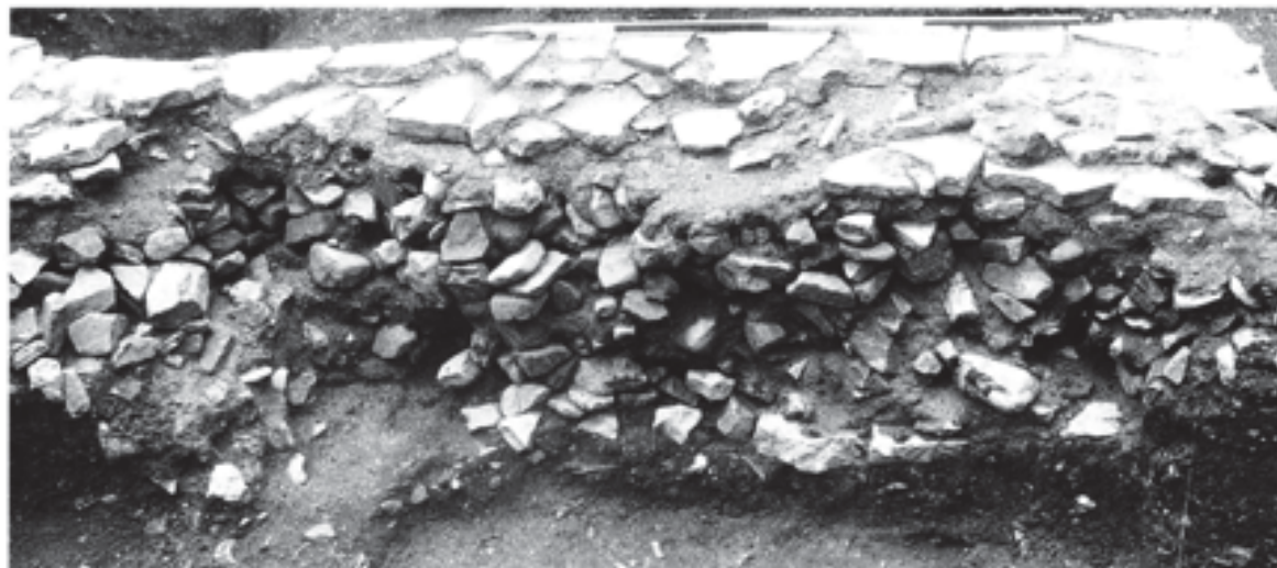
Fig. 77 Part of the north wall of St Mary's chapel, showing the pebble-rubble core exposed by a later grave-cut. On top of the foundation is the lias walling of the second phase of the chapel. Scale of 2 m
