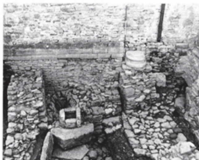
Fig. 139 Lady Chapel. General view of the abutment of the foundations of the south-west chapel to the cloister. The masonry in the centre foreground is the top of the great conduit. Scale of 2 m
