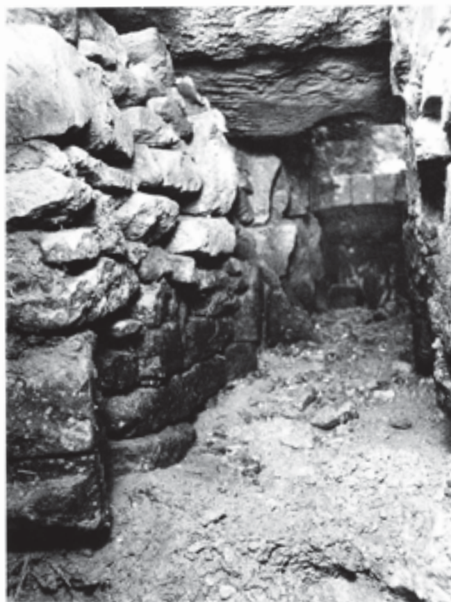
Fig. 405 View east inside the post-medieval conduit running between the Camery wall and St Andrew's Well (plan, Fig. 395, 'D' to 'B'). The furthest part of the channel is open topped, and the voussoirs of the bridge beside the well can be glimpsed in the distance
