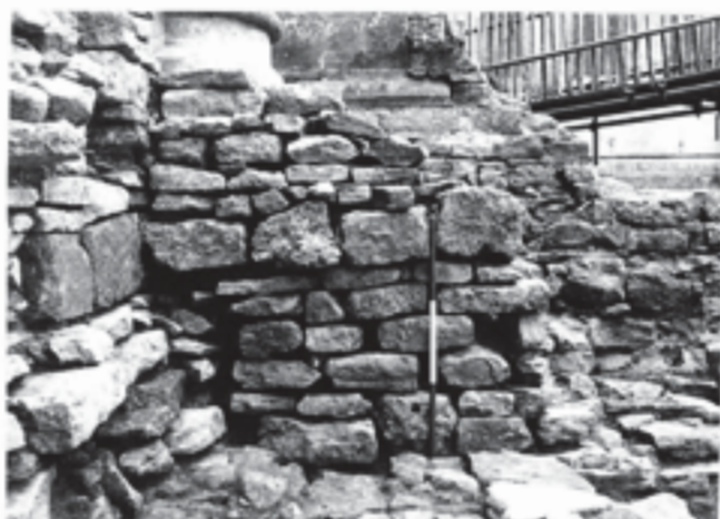
Fig. 84 South link-wall of St Mary's chapel, showing the superimposition of the two phases of masonry (F182 and F332), with a slight overhang between them. Scale of 75 cm
