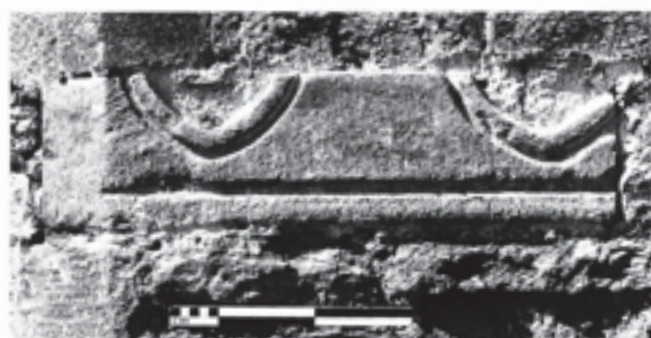
Fig. 316 Lintel embodying the heads of two pointed and moulded arches, thirteenth century. Reused, inverted, in the north-east face of the library stair-turret (Structure 13)
