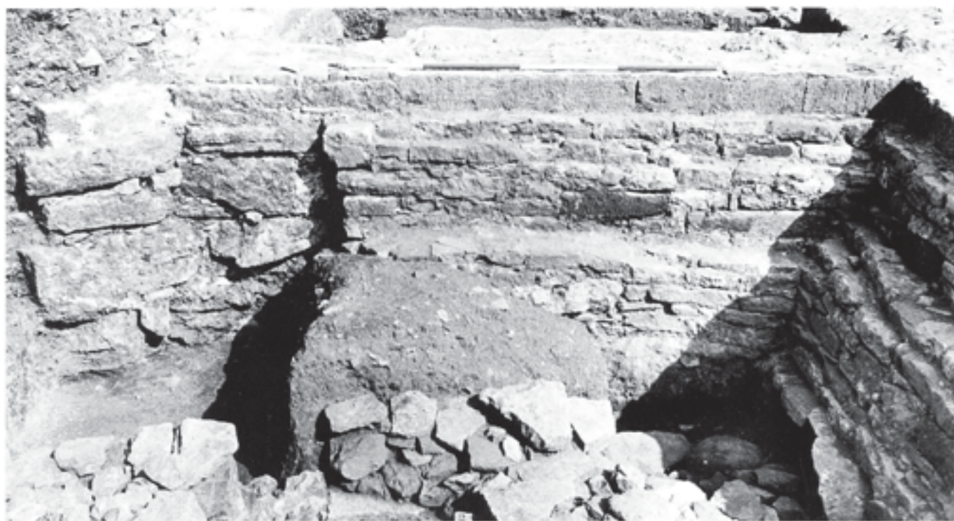
Fig. 227 Foundation of the west wall and diagonal buttress of the sacristy of Stillington's chapel, showing the incorporation of an original chancel buttress. The shadow (left of centre) marks the junction between the two periods of construction. Scale of 2 m
