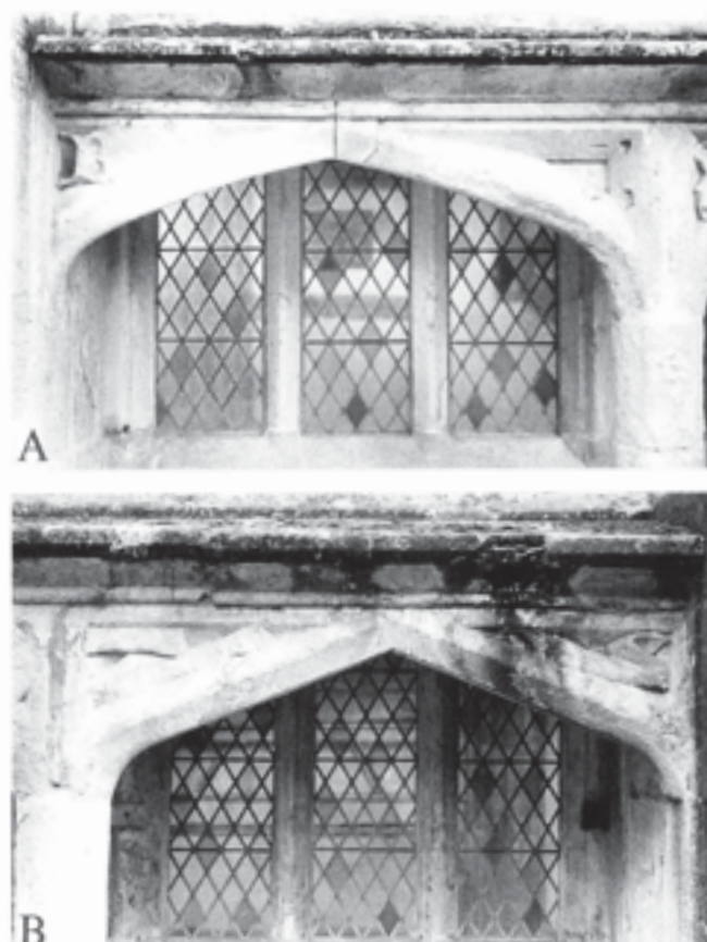
Fig. 332 Details of the arched heads of the pentices. A Left-hand head of the southern pentice (Structure 19A), showing the initial 'B', and the empty socket of a second letter (lost), in the spandrels; B Right-hand head of the northern pentice (Structure 19B), showing ribbon decoration in the spandrels
