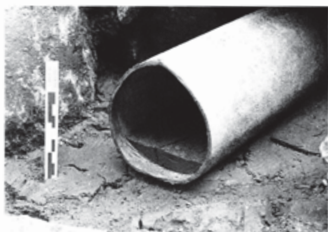
Fig. 421 Section through the pipe-duct (F132) and the lead water-pipe (F133, length 3). A (upper) The realigned duct of 1477; in the centre foreground is one of the pad-stones that supported the pipe before the duct was filled with liquid clay (removed in this view). B (lower) Close-up of the sectioned pipe, showing the final internal silting. The clay packing (F134) can be seen here beneath the pipe. Scales: (A) 25 cm; (B) centimetres and inches
