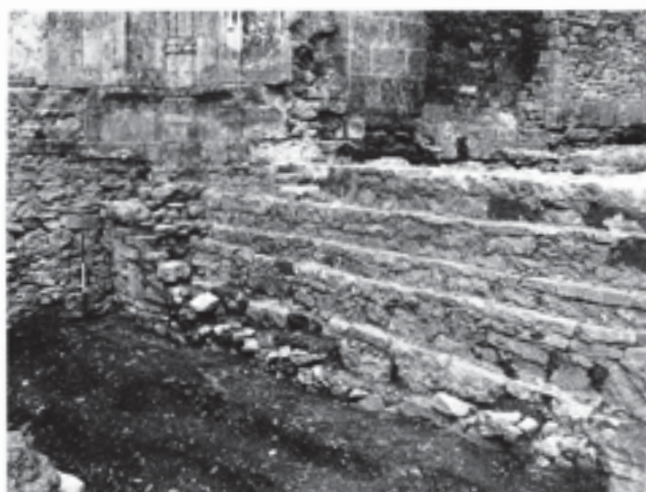
Fig. 209 Interior of the north wall of Stillington's nave, contrasting its neatly stepped foundation (right) and the rough rubble foundation added against the cloister (left) for the support of the wall-bench and screenwork at the west end. Scale of 75 cm
