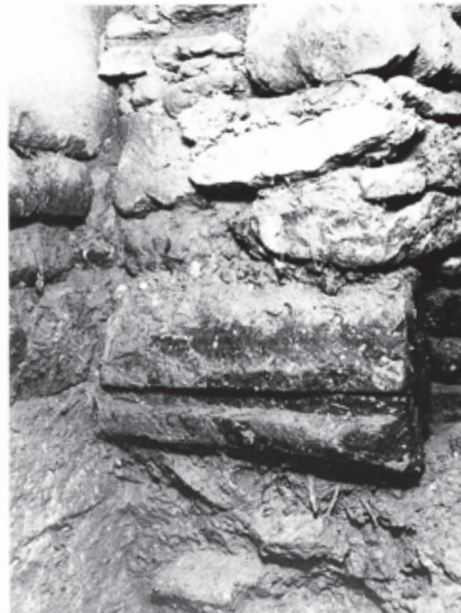
Fig. 406 Rubble construction of the post-medieval conduit east of the Camery wall ('D'), showing the base-course made from a block of channelled masonry salvaged from an earlier sluice (cf. Fig. 405). The conduit here is built on a bed of mud and rubble
