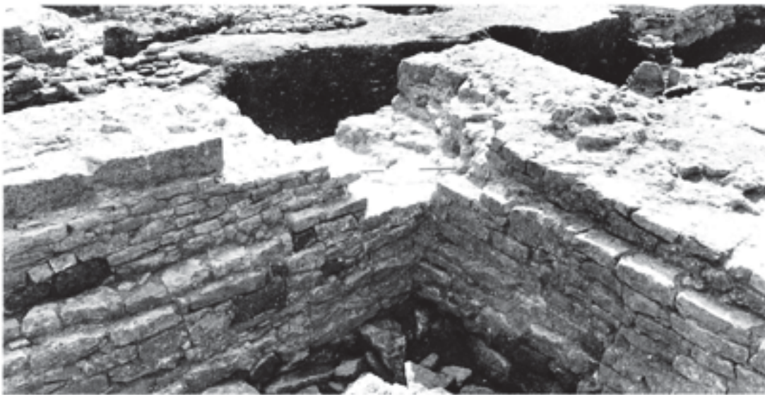
Fig. 259 Crater in the foundation of the north-east crossing pier of Stillington's chapel, caused by the use of an explosive charge during the demolition. Scale of 75 cm
