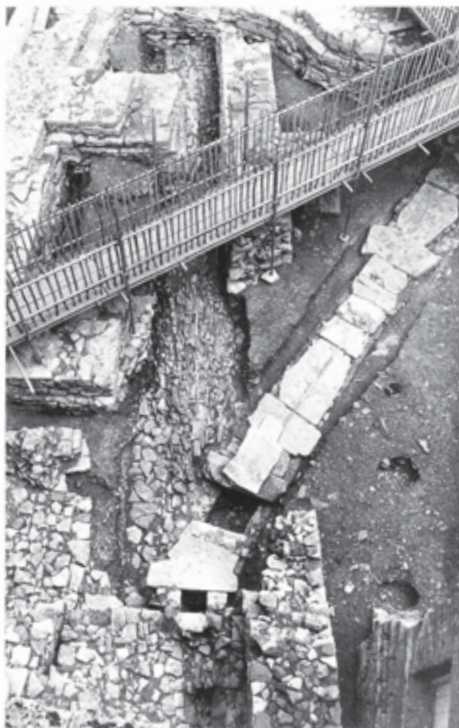
Fig. 390 The converging routes of medieval conduits in Areas 4 and 5, approaching the cloister from the east (top). The vaulted conduit of c. 1190–1200 runs through the centre of the picture, with the south aisle wall of the early Lady Chapel alongside (right); the diversion of 1477, with its slabbed top, enters from the upper right. Part of the transept turret of Stillington's chapel is visible at the top. Scales of 2 m
