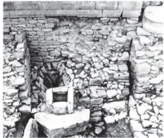
Fig. 281 Robbed foundation for the unbuilt buttress at the junction of bays E 4 and E 5 on the east cloister. Note how the chamfered plinth at the base of the main wall was carried across the intended site of the buttress, and returned along the south wall of the Lady Chapel (right). The 75 cm scale rests on the front edge of the buttress foundation
