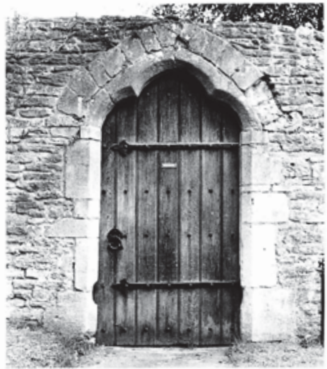
Fig. 295 Possible recycled thirteenth-century doorway from the south cloister porch, now used as a gateway in the late medieval wall separating Palace Green from the bishop's garden
