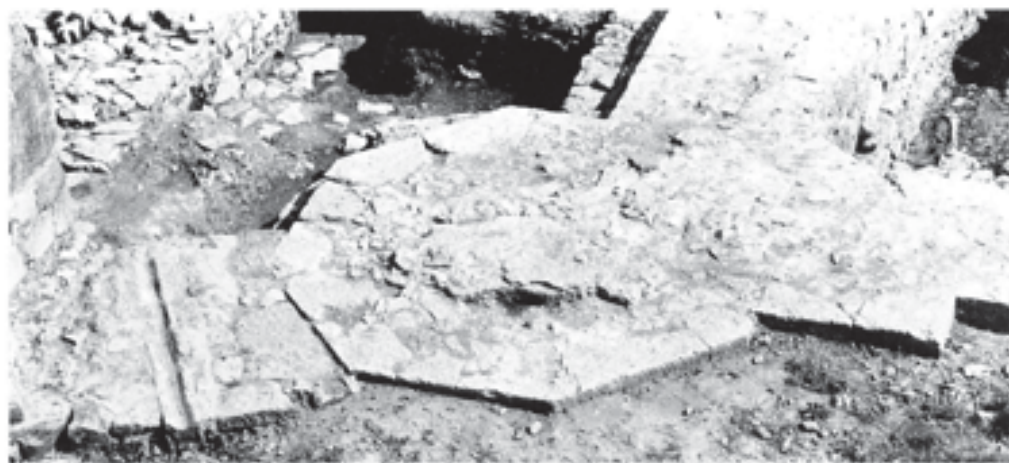
Fig. 229 The base of the north-west stair-turret of Stillington's chapel and foundation for the later bridge linking it to the cathedral. View north-east
