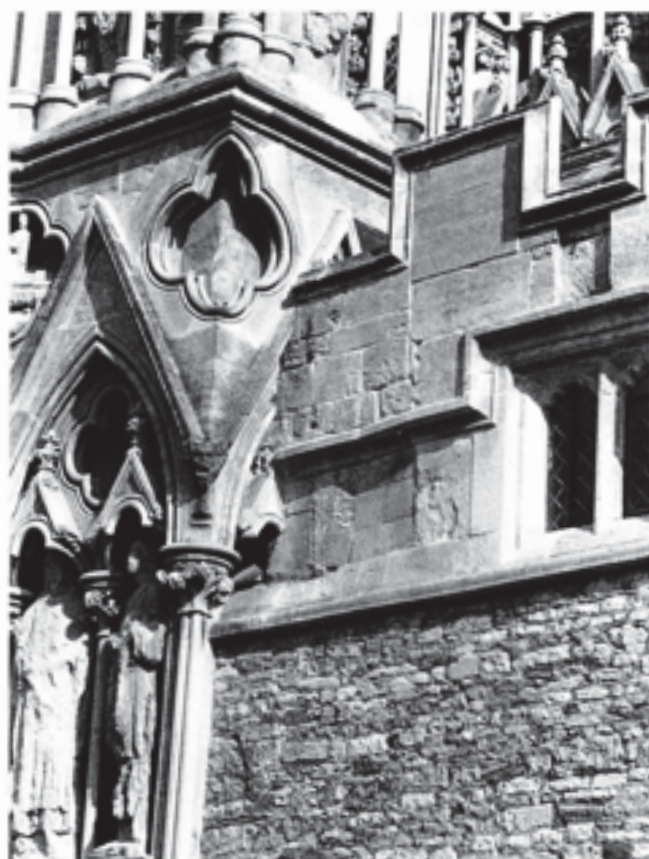
Fig. 282 Union of the outer wall of the west cloister with the buttress of the south-west tower. The remains of the thirteenth-century cloister coping can be seen disappearing under a gablet intended as a statue canopy. The vertical joint and misalignment in the fifteenth-century upper storey of the cloister suggests that it initially stopped just short of the tower
