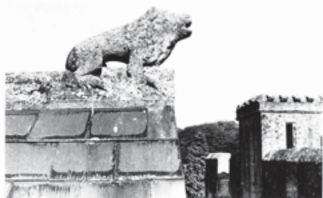
Fig. 317 Mid-fifteenth-century ridge finial, representing a crouching lion, on the south gable of Bubwith's library extension. To the right is the crenellated chimney stack serving the muniment room fireplace
