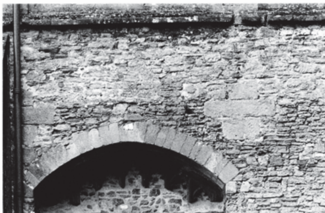
Fig. 303 Two groups of large ashlars in the east wall of the cloister, bay E 7 , apparently counterpoise blocks associated with an inserted stone vault of mid-thirteenth-century date. Below is the late fifteenth-century arched entrance to the Holy Cross chapel (English Heritage)
