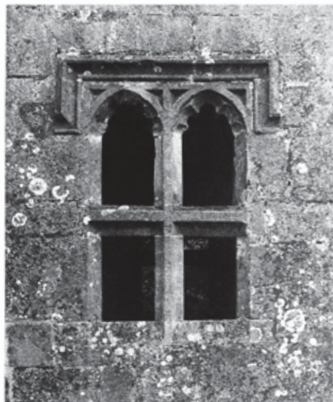
Fig. 414 West window of the well-house
