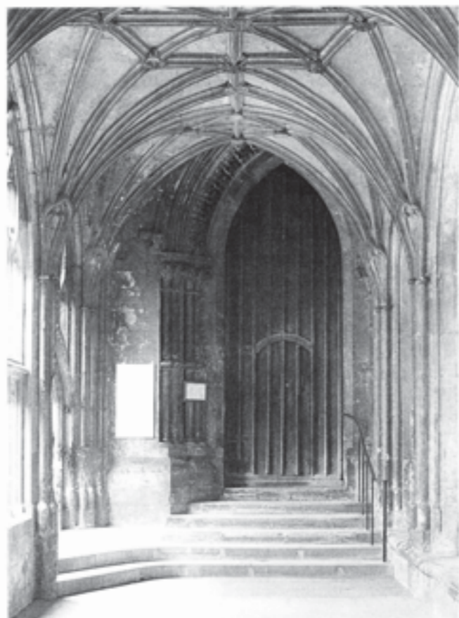
Fig. 119 The south transept portal of the late 1180s, asymmetrically abutted by the east cloister and partly obscured by the vaulting of c. 1420 (Jerry Sampson)
