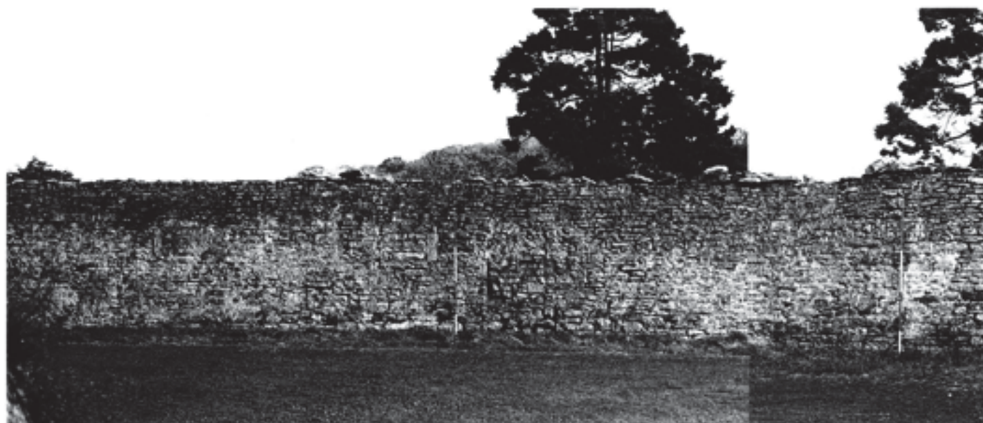
Fig. 357 General view of the east Camery wall, from the west in 1979, after being stripped of vegetation. The right-hand ranging-pole stands at the bend in the wall, from which point northwards (left) it was realigned in the early fourteenth century. Scales of 2 m
