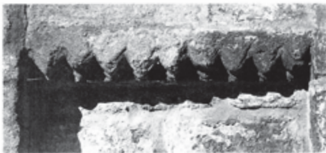
Fig. 438 Romanesque chevron-moulded string-course (no. 14), now used as a false-lintel in the south-west corner of the Vicars' Hall. Length 75 cm (Jerry Sampson)
