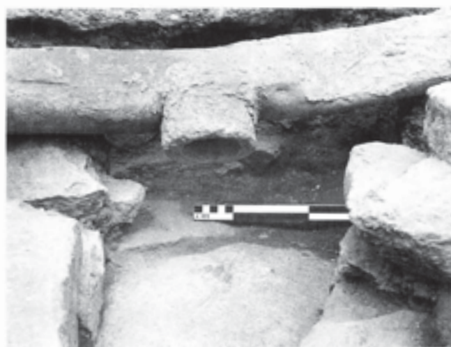
Fig. 426 Close-up view of the washout point on pipe length 5, as seen inside manhole F95. Scale of 25 cm
