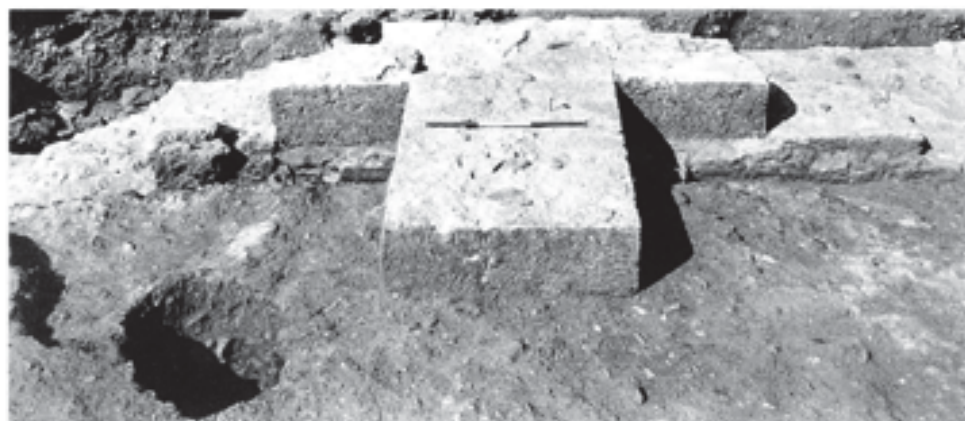
Fig. 202 Stillington's chapel. Footing-course of large Chilcote blocks of buttress F1208f, in relation to contemporary ground level on the south side of the chancel. View north. Scale of 75 cm
