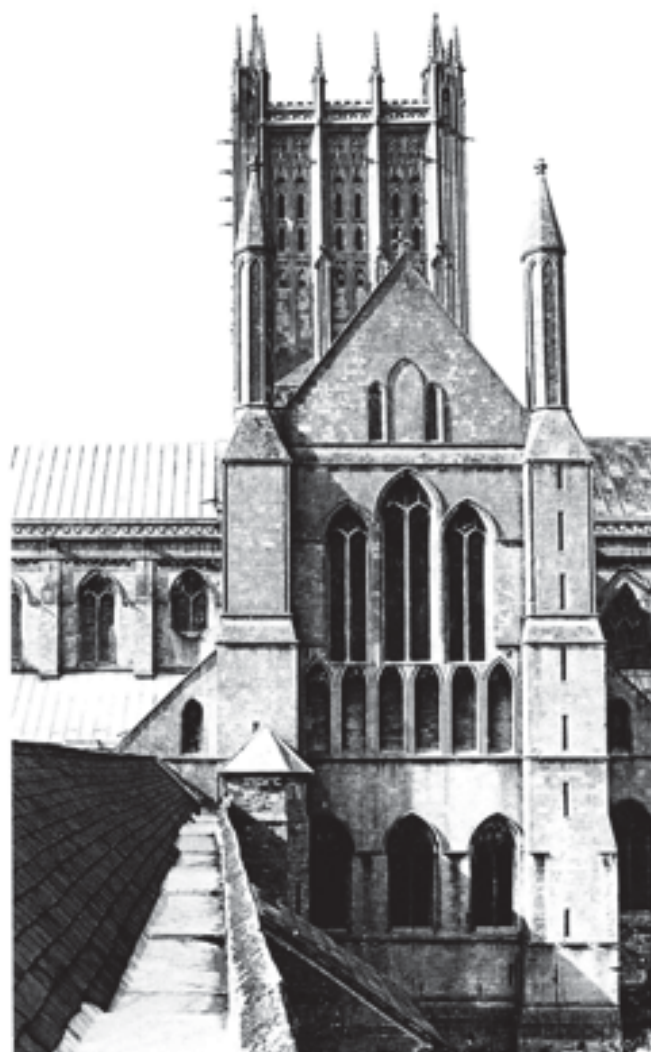
Fig. 296 The south front of the south transept, showing the abutment of the east cloister and stair-turret. The library roof and parapet enter from the bottom of the picture. Note the broad, shallow parapet gutter
