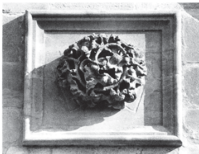
Fig. 245 Vault-boss (no. 19) from Stillington's chapel, reused as a decorative feature and set in a recessed panel over the doorway to the west cloister porch. It was possibly placed there in the sixteenth century. See also Fig. 462
