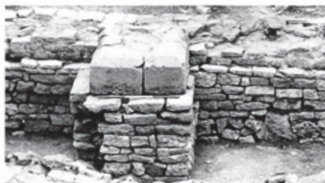
Fig. 142 Lady Chapel. South aisle foundation and mid-wall buttress (F186a), showing the surviving plain-chamfered plinth. Scale of 75 cm
