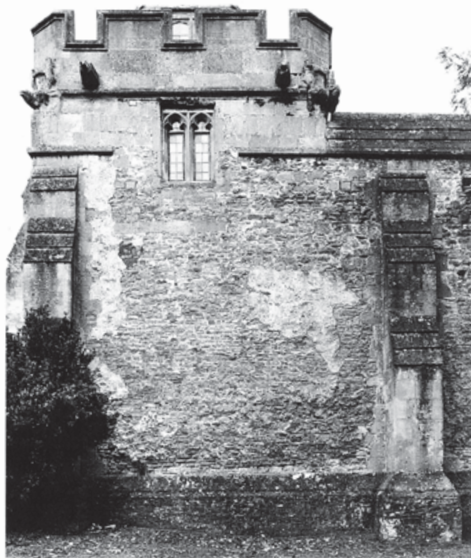
Fig. 292 Cloister bay S 1 , with the fifteenth-century crenellated parapet (1992). A glimpse of the recessed gable of the west range can be seen through the central embrasure of the parapet. For a key to structural features, see Fig. 291 (English Heritage)
