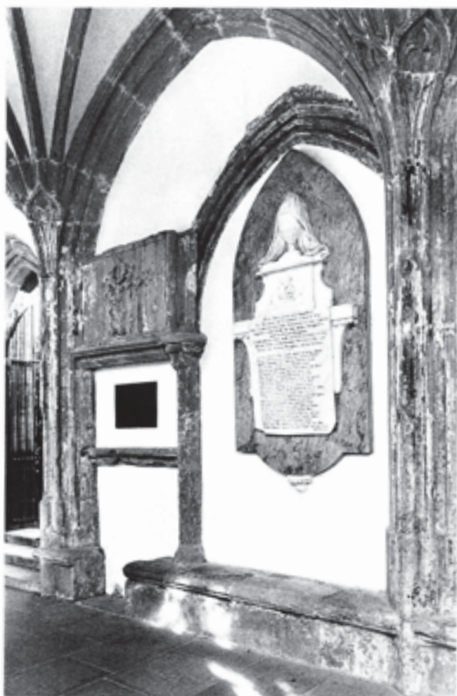
Fig. 326 Cloister bay 6, showing the outline of the original entrance arch to the Lady Chapel (centre right), Stillington's doorway to the new chapel (far left), and the probable setting of the pyx of St Saviour between the two
