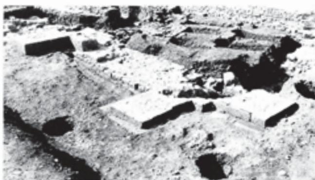
Fig. 222 South-east corner of Stillington's chancel, showing the survival of footing-courses to buttresses, and large postholes association with construction scaffolding. Scale of 75 cm
