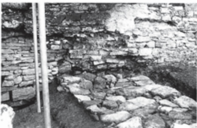
Fig. 85 North link-wall of St Mary's chapel (first phase, F703A), passing under the foundation of the east cloister. The attachment scar of the second phase (F703B) can be seen, together with the contemporary cloister foundation to the right. Left of the scar is the masonry of the squared-off apse (F1517) of St Andrew's church. Scale of 75 cm
