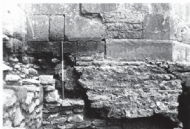
Fig. 315 Detail of the junction between the late twelfth-century east cloister (left) and the base of the library stair-turret (Structure 13). The turret and its foundation can be seen to override, respectively, the earlier buttress (E7a) and its foundation. Scale of 75 cm. For the elevation, see Fig. 312
