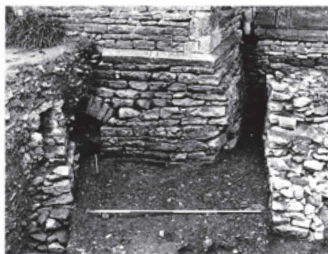
Fig. 319 Plinth and foundation of the north-east corner of the latrine tower revealed by excavation. The segmental arch enabled the contents of the cess pit to seep into the adjacent ground. Scale of 2 m
