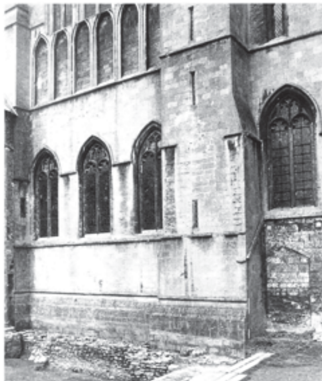
Fig. 228 The south transept of the cathedral, showing the projecting stair-turret to which the bridge from Stillington's chapel connected. For a detail, see Fig. 231. Scale of 2 m
