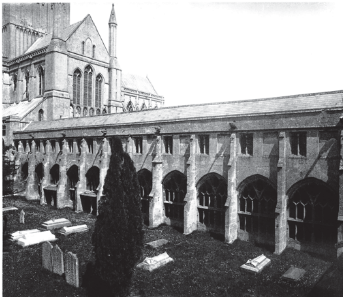
Fig. 266 Bubwith's library over the east cloister, taken from the roof of the south cloister by Thomas Phillips between 1895 and 1900. Note the fresh, recumbent grave-slabs (left of the yew tree), encroaching on the site of the dipping-well (then infilled). The stone-roofed penteries (Structures 19A–B) can be seen between the buttresses of bays 4 and 6 (Wells Cathedral Library)
