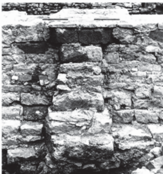
Fig. 210 Stepped projection in the foundation of the north wall of Stillington's nave, intended to receive the base of the wall-shaft between the first and second bays. Note the canted ashlar blocks at the top. Scale of 75 cm
