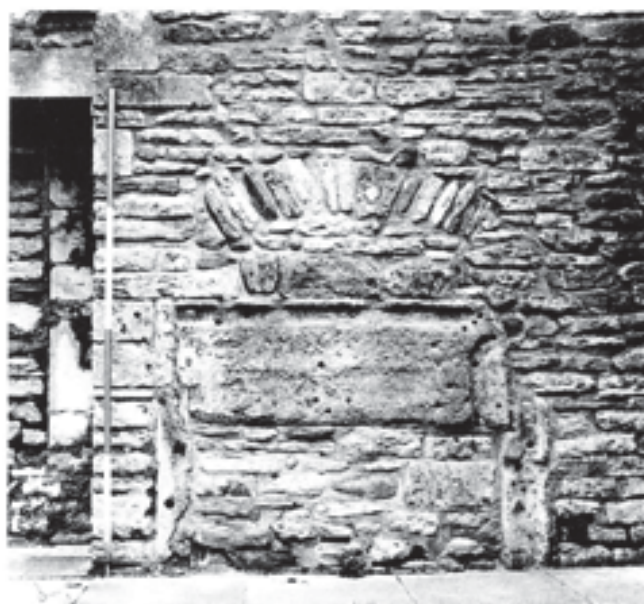
Fig. 353 Detail of the two infilled fireplaces(?) in the north wall of the choristers' house. Scale of 2 m
