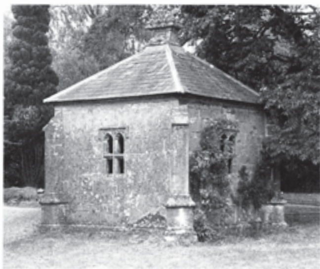
Fig. 410 Views of Bekynton's well-house of 1451 in the grounds of the Bishop's Palace from the south-west. A (upper) From a drawing (reversed) by Orlando Jewitt, c. 1860. B (lower) As existing in 1979
