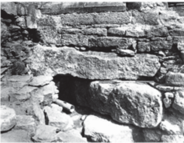
Fig. 200 The lead water-pipe of c. 1451–53 emerging from beneath the junction between the east cloister (left) and the south wall of Stillington's chapel. The large sandstone blocks provided a protective casing. Scale of 75 cm
