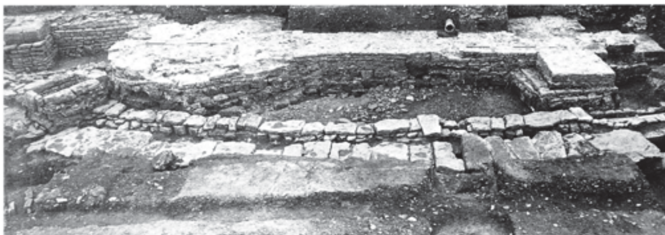
Fig. 217 View of the south transept of Stillington's chapel, from the south, showing robbing to a level below the footing-course of the octagonal stair-turret. The cover-stones of the conduit and pipe-duct can be seen in the foreground. Scales of 2 m
