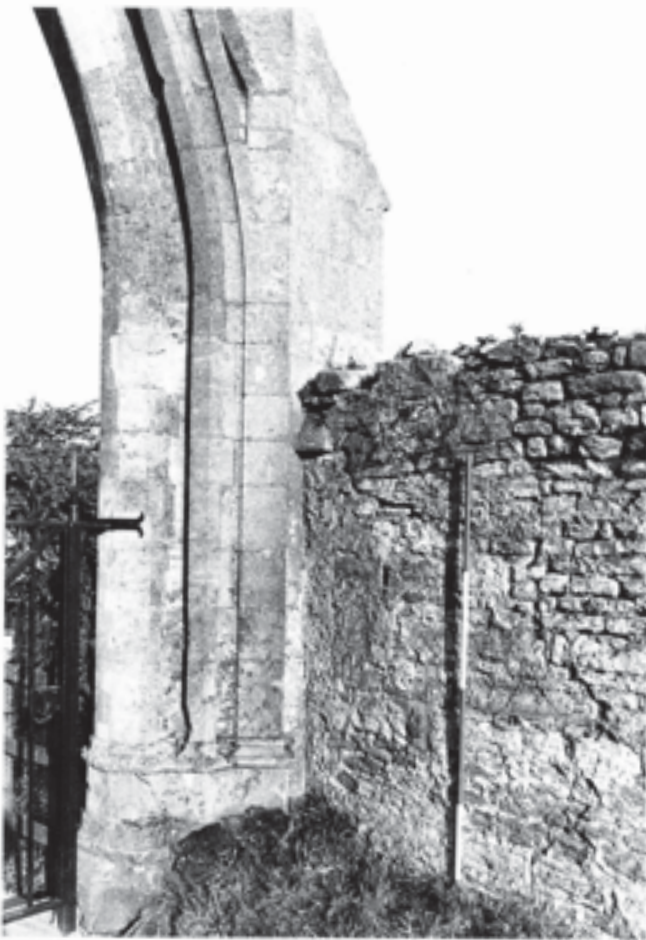
Fig. 363 Detail of the mouldings of the buttress-arch and abutment of the Camery wall on the south. Note the beginning of a steeply profiled ashlar coping embedded in the wall-top. Scale of 2 m
