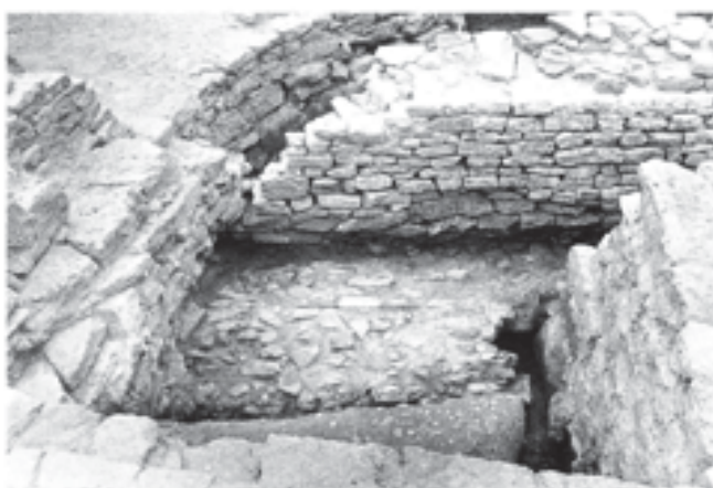
Fig. 219 The junction between Stillington's south transept and the early medieval conduit, looking south. The vaulted roof of the conduit has the 2 m scale lying on it. It is severed by the transept foundation (left) and one of the nave buttresses (right). Note the offset and other changes in the masonry of the transept where its construction was interrupted when the conduit was encountered. Beyond the conduit, and partly overlying it, is the south aisle wall of the earlier Lady Chapel
