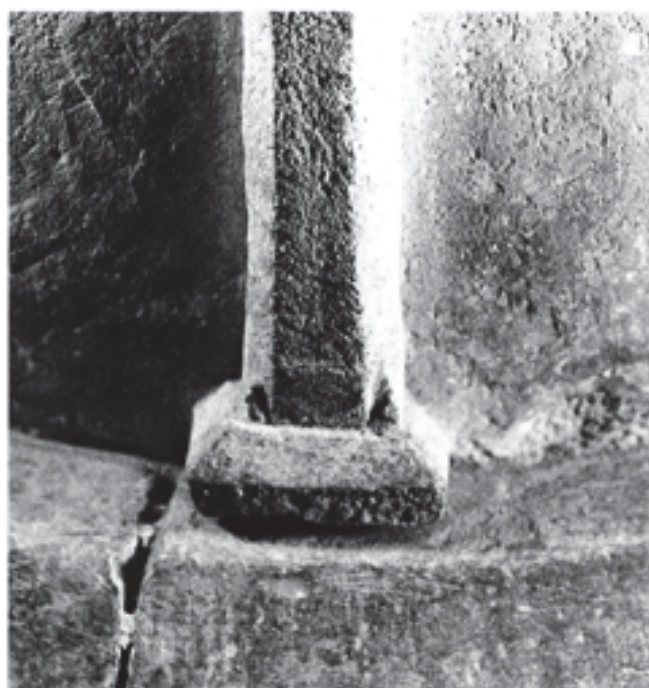
Fig. 131 Font: detail of pilaster-base no. 2/3. The chamfers and broach-stops are secondary (Jerry Sampson)
