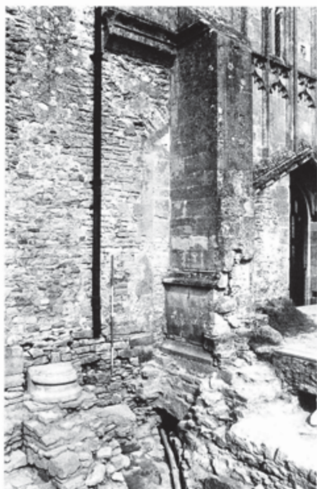
Fig. 233 The remaining stub of the south wall of Stillington's nave abutting the cloister. This fragment includes the west splay of one window, and it blocks the original entrance to the Early English Lady Chapel. The lead water-pipe of c. 1451–53 is seen below, set into a protective duct. Scale of 2 m
