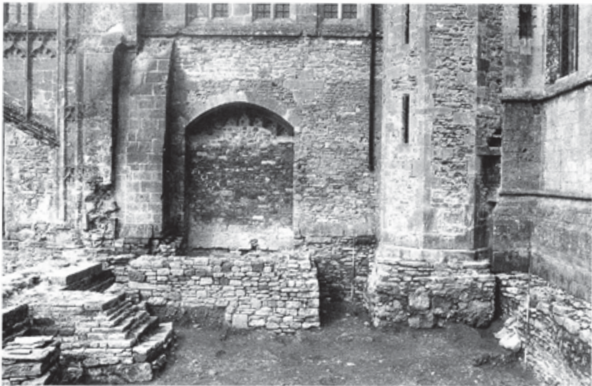
Fig. 320 General view of the excavated foundations of the chapel of the Holy Cross-by-the-Cloister (Structure 18), with the segmental entrance arch and remains of the traceried screen embedded in the east cloister wall. Scales of 2 m
