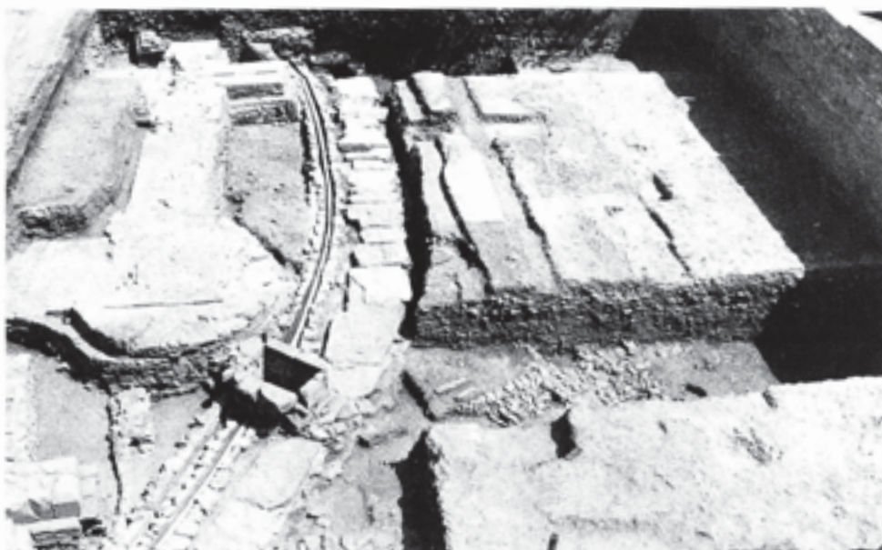
Fig. 418 General view looking east, showing the conduit and lead water-pipe of 1477, curving around the south transept of Stillington's chapel. An inspection chamber can also be seen, adjacent to the turret base. The capstones have been removed from the pipe-duct, but are still in place over the conduit. The surface of the late medieval masons' yard is seen on the right. Scales of 2 m
