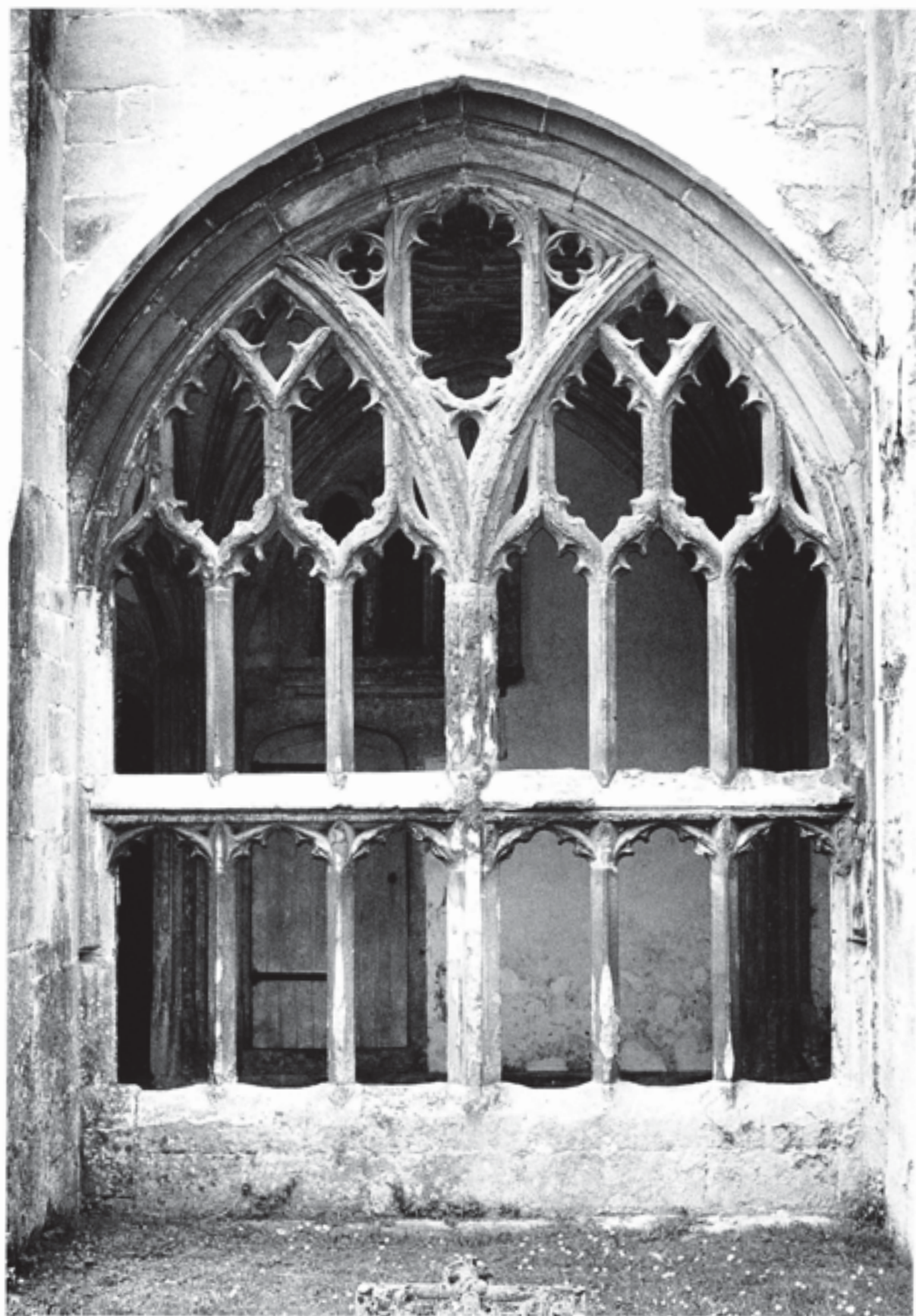
Fig. 271 A typical traceried cloister bay, seen here in 1980 before reglazing. The design dates from c. 1420, but this example, in the west cloister (bay 36), is later in the series (c. 1460–70). Within the walk can be glimpsed the doorway and window of the stair-turret adjoining the cloister porch (Structure 25A). (Jerry Sampson)
