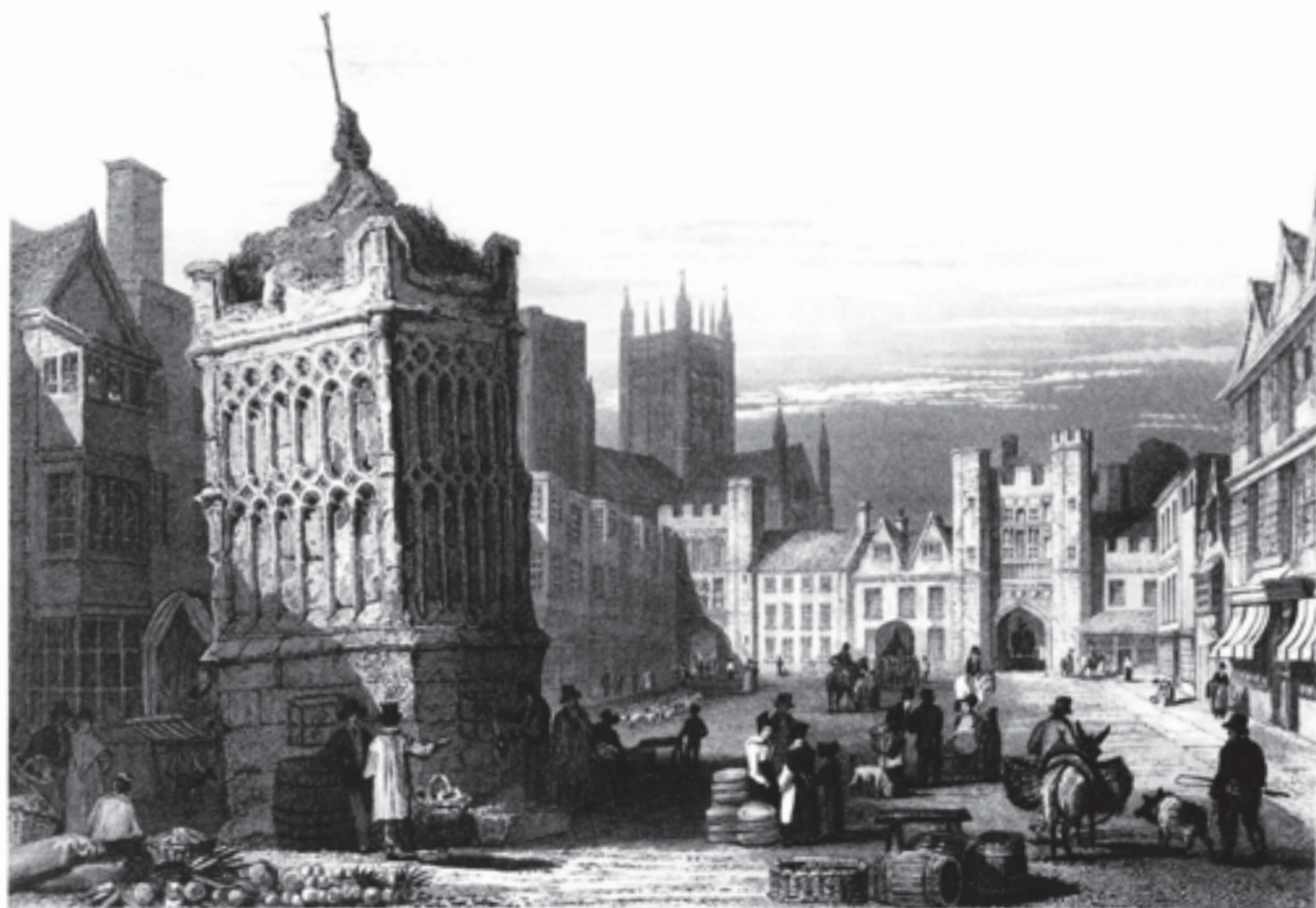
Fig. 415 Bekynton's conduit-head of 1451 in the market place, from the south-west in c. 1800. The architectural detail is meticulously represented. After Britton 1830
