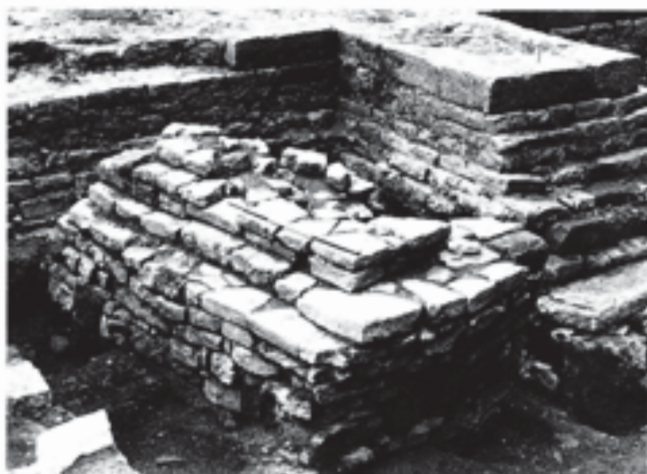
Fig. 138 Stepped foundation of the north-east buttress of the north aisle of the Lady Chapel (F1007c). Behind it is the buttressed north nave foundation of Stillington's chapel. View south-west. Scale of 75 cm
