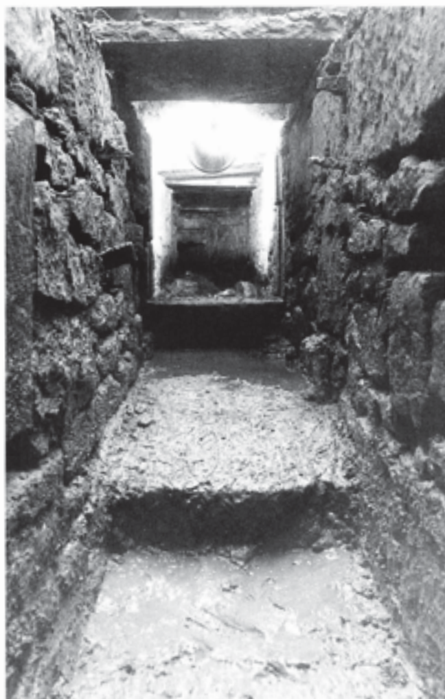
Fig. 400 View west inside Bekynton's conduit, after draining and removal of post-medieval fills. The two steps in the floor are original
