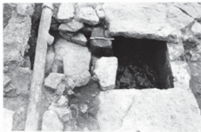
Fig. 427 Lead water-pipe and the channel leading from the washout point to the conduit, after dismantling the sides of the manhole (F95). View east. Scale of 25 cm
