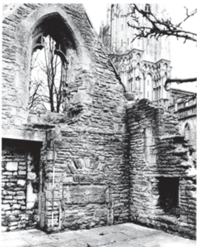
Fig. 352 Interior of the choristers' house, looking north-east
