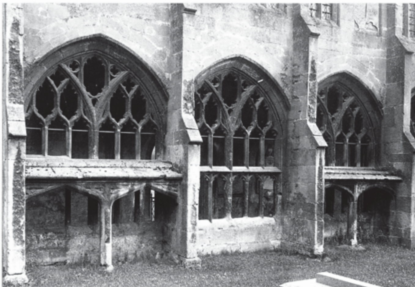
Fig. 330 The two pentices (Structures 19A, right; 19B, left) constructed between the buttresses of bays 4 and 6 of the east cloister. Photographed by T.W. Phillips between 1895 and 1901 (Dean and Chapter of Wells)
