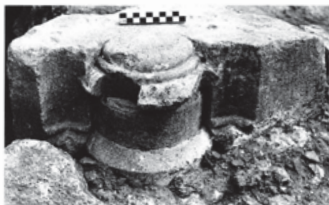
Fig. 143 Mid-thirteenth-century moulded base of a door jamb(?), reused in the foundation of Stillington's chapel. For the moulding profile, see Fig. 141F. Scale of centimetres
