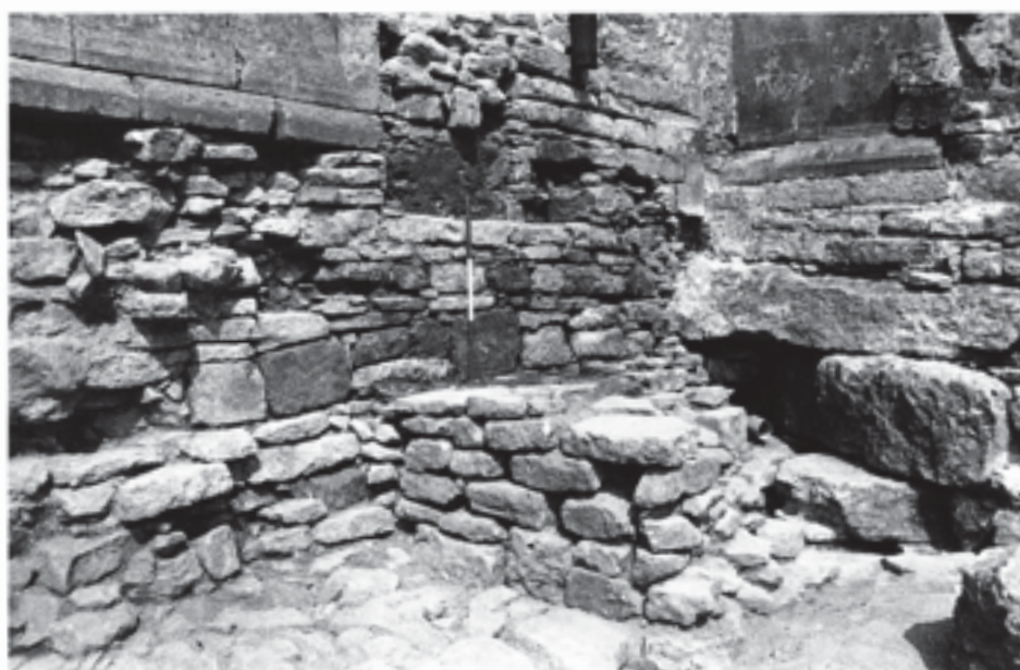
Fig. 82 The east cloister foundation (left), clasp and over-riding the lowest five courses of the south link-wall (F332) of St Mary's chapel, upon which the scale (75 cm) stands
