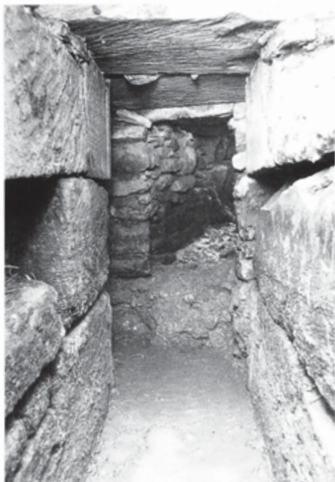
Fig. 407 View east inside Bekynton's conduit, beneath the Camery wall at sluice 'E'. In the middle distance is the junction ('D') with the post-medieval extension beyond. Its clay and rubble floor is at a higher level, and relates to the raising of the lake in the early nineteenth century
