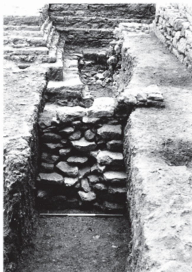
Fig. 307 Structure 12: section through the foundation of the east wall, showing also the shallow setting (right) for a presumed internal bench. Scale of 75 cm
