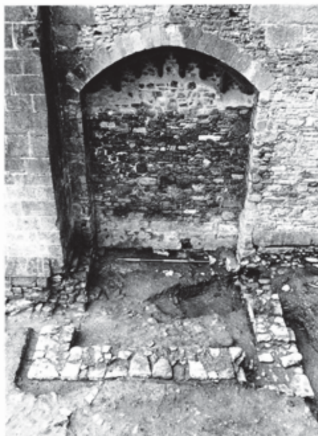
Fig. 15 Re-excavation of foundations exposed by trenching in 1894 of a small building (Structure 18) adjoining the east cloister; this was identified at the time as an 'office', but is probably the chapel of the Holy Cross-by-the-Cloister. Scale of 2 m
