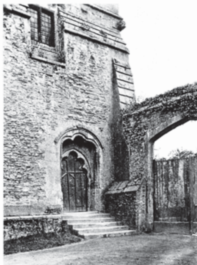
Fig. 278 Early thirteenth-century south doorway (with original door) to the cloister, and the arched entrance of 1433 leading into the masons' yard beyond. Taken c. 1865. After Parker 1866b
