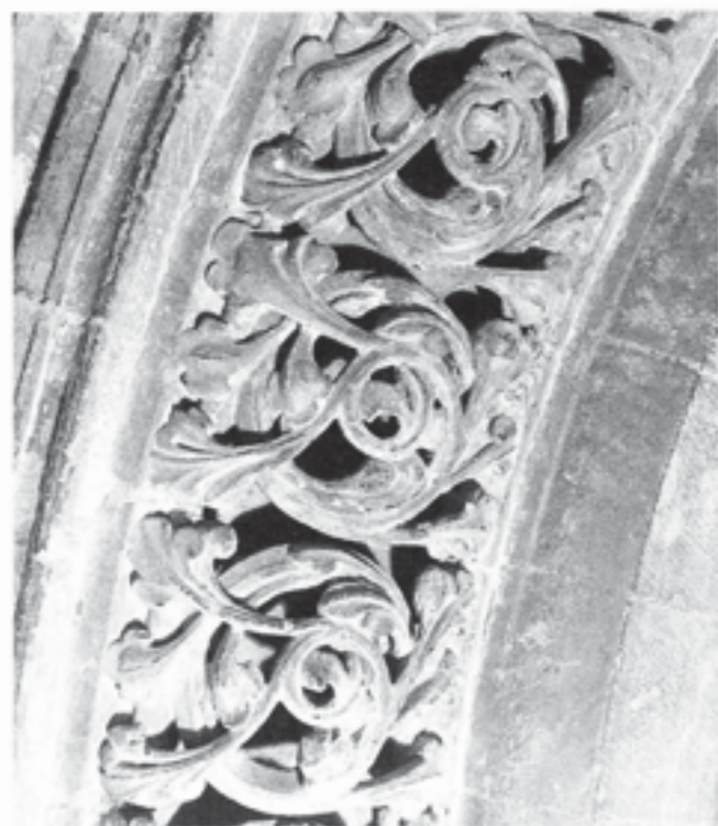
Fig. 120 Detail of fretted, stiff-leaf carving in Chilcote stone on the head of the south transept doorway. Late 1180s. For the moulding profile of the arch, see Fig. 121 (George H. Hall)
