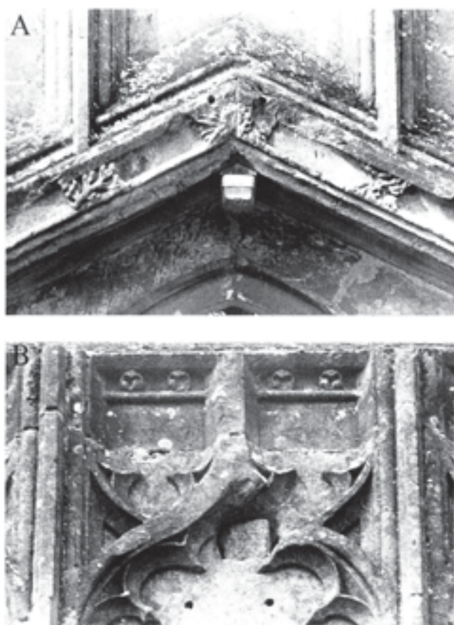
Fig. 235 Stillington's chapel. A Detail of the enriched string-course over the entrance; B One of the sections of ball-flower string-course, inserted between the super-mullions of the truncated arcading in the west wall
