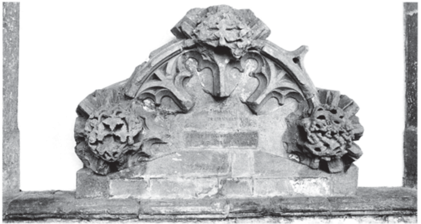
Fig. 242 Reconstructed central vault-ring representing the north transept bay in Stillington's chapel; chain-holes are arrowed. Display constructed in the east cloister in 1894 (boss and segment nos. 8–12)
