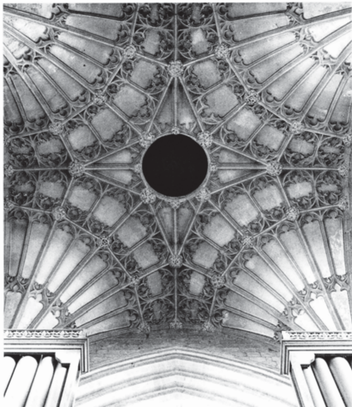
Fig. 250 Fan vault, probably erected by William Smyth in the 1480s, over the crossing in Wells Cathedral. East is at the bottom (Jerry Sampson)
