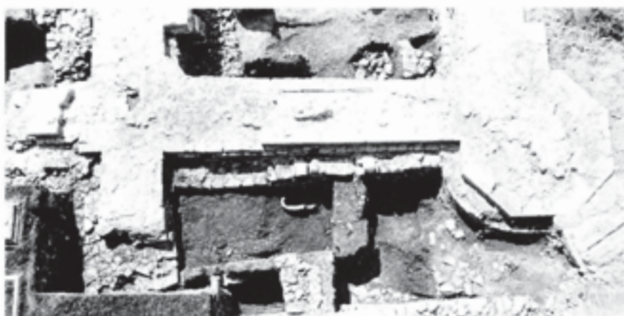
Fig. 214 The north wall, buttresses and stair-turret of Stillington's north transept, showing the close proximity to the cathedral transept and its foundation (which just appear at the bottom of the frame). Scale of 2 m
