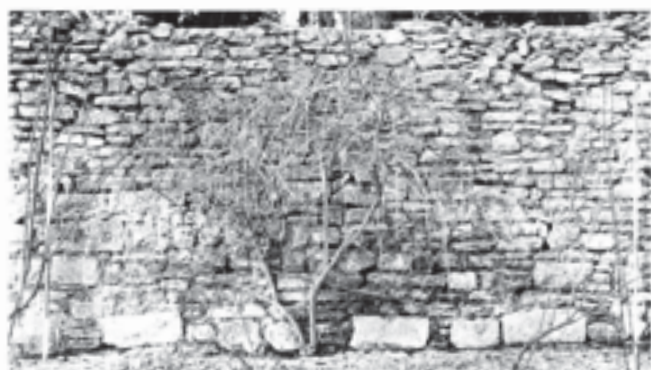
Fig. 361 Detail of the construction of the early thirteenth-century Camery wall, showing reused ashlar blocks in the lowest visible courses. Scales of 2 m
