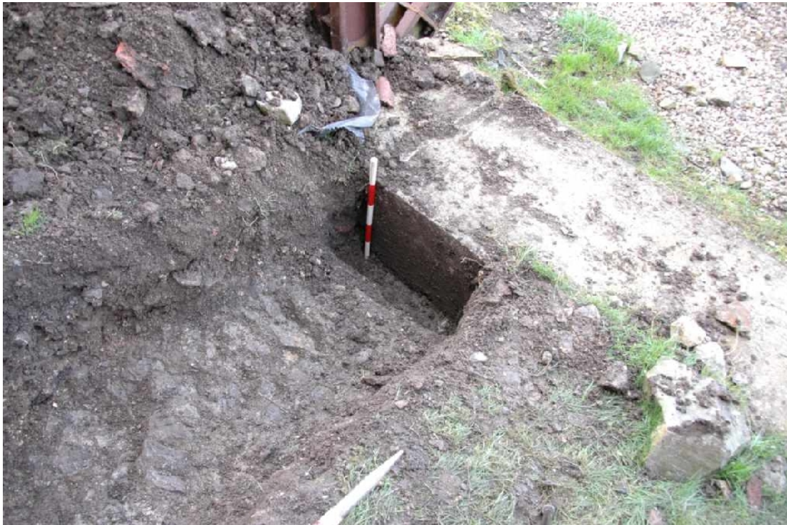
Illus 6 TP 1 detail of buttress base
