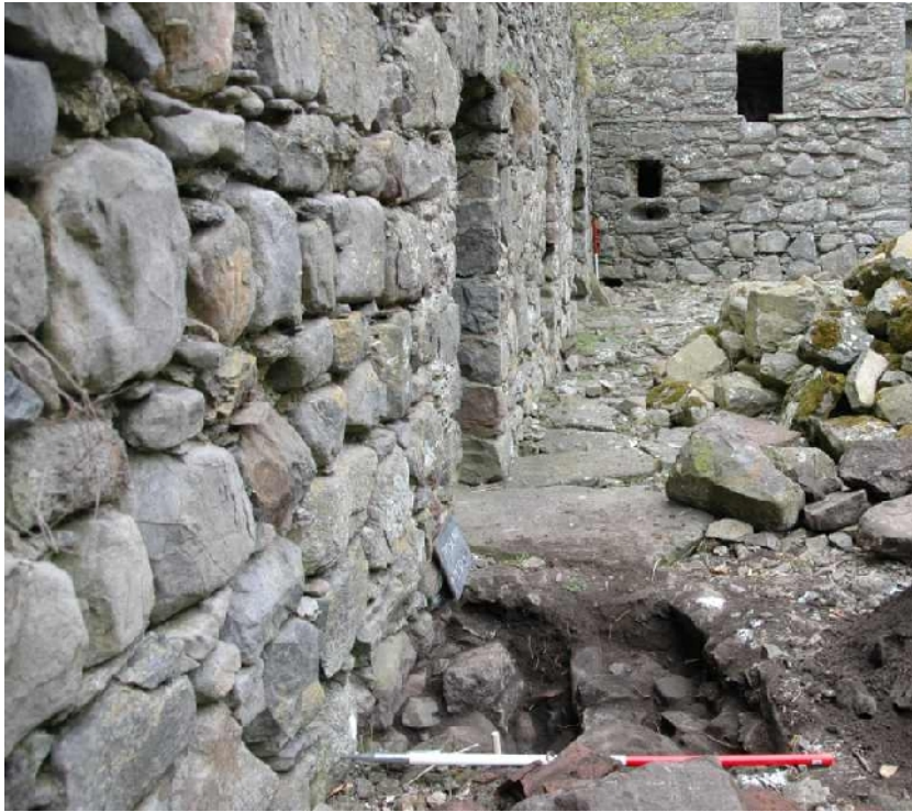
Illus 23 TP 5 stone drain looking E showing capstones extending to drain outlet from stair tower
