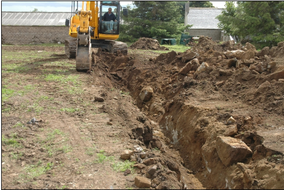
Illus. 5: Cable trench (3) running through natural rock, looking S
