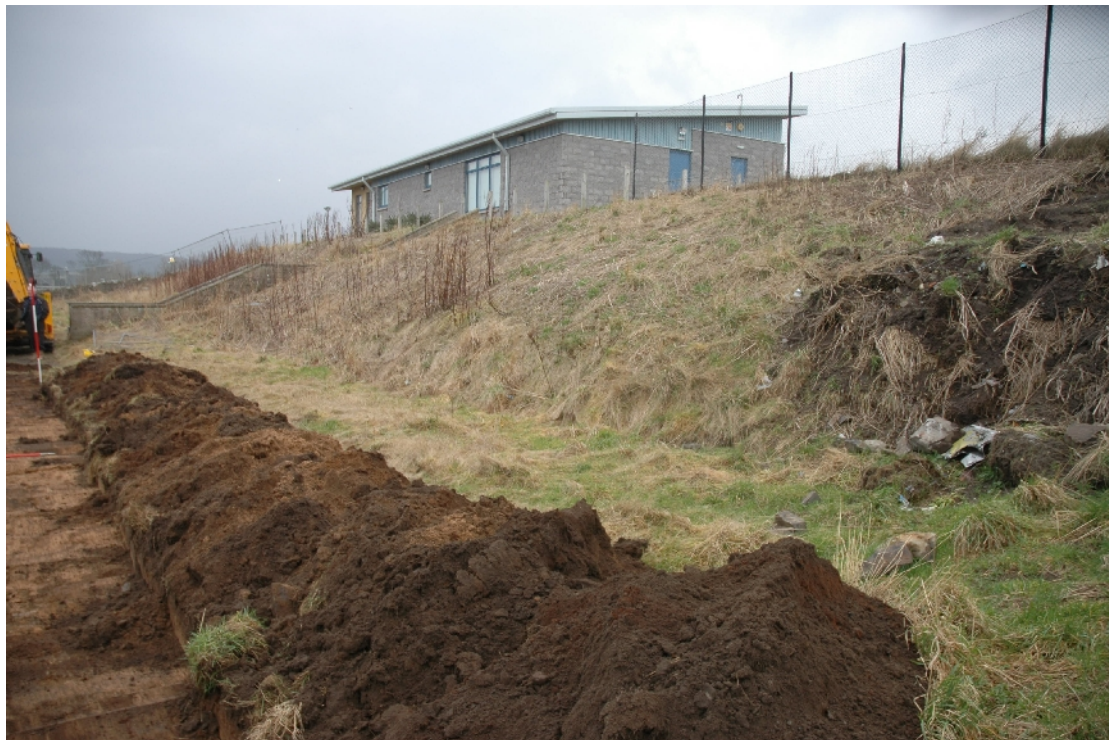
Illus 5 Showing difference in level between Areas D and E with nearly 4m of made- up ground at E end of Area E.
