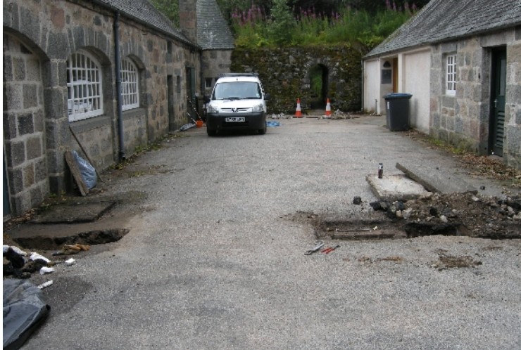
Illus 2 Location of site, looking S with the W exterior wall of the Stable Range of building to LHS and the freestanding W range to the RHS
