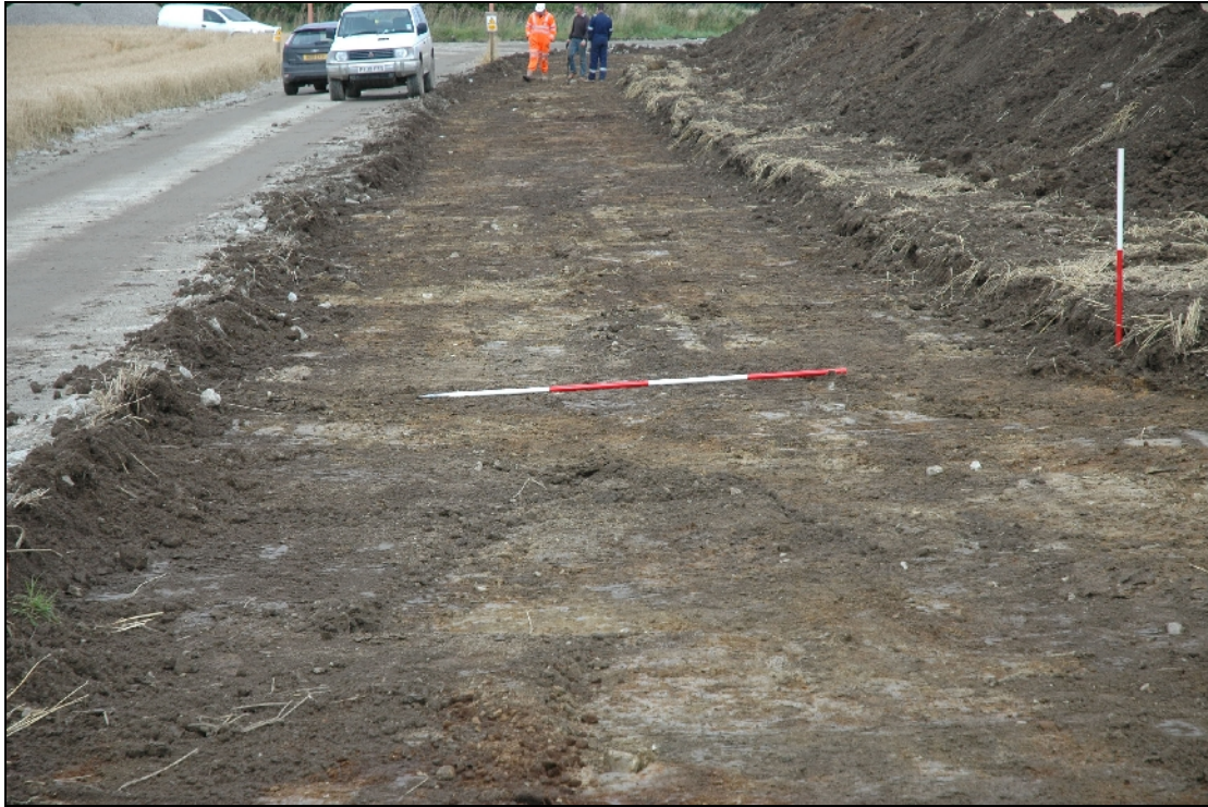
Illus. 4: Detail of cable trench corridor, looking N.
