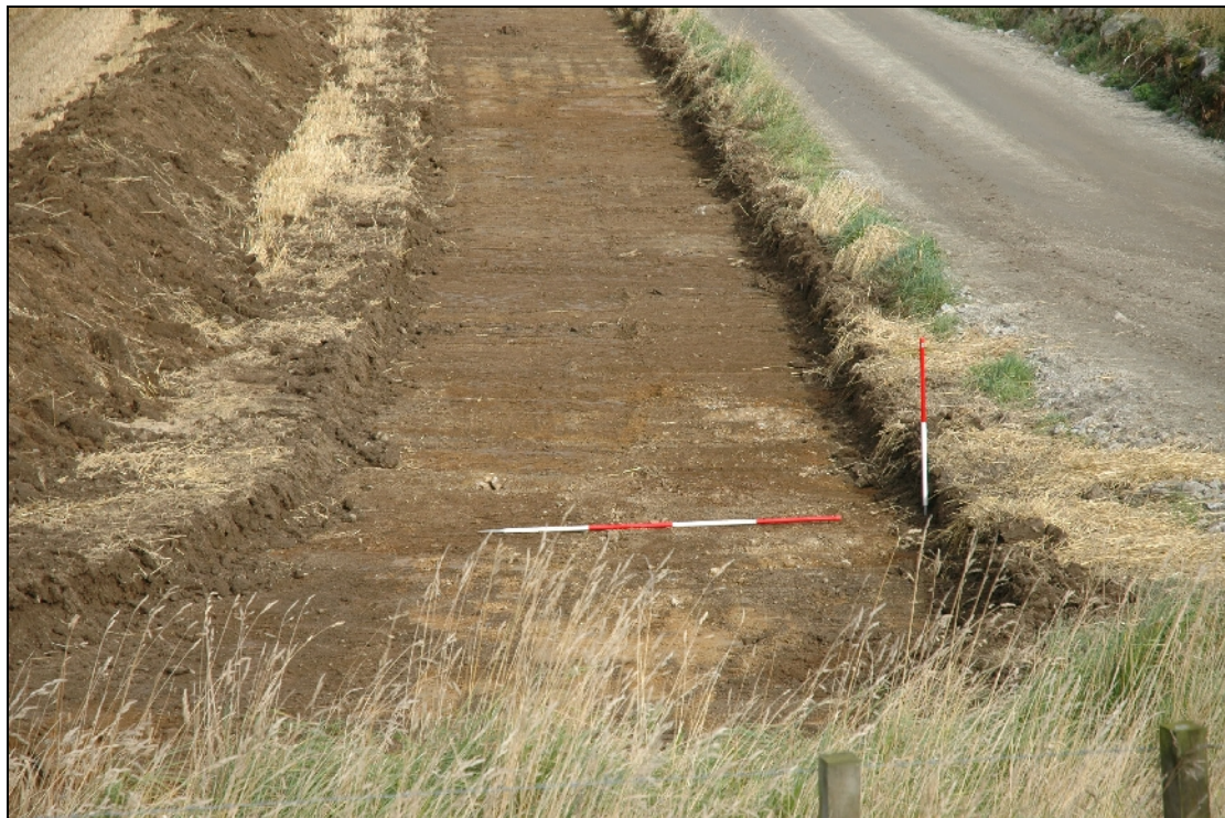
Illus. 7: Cable trench corridor, N of farm buildings towards Turbine 2.
