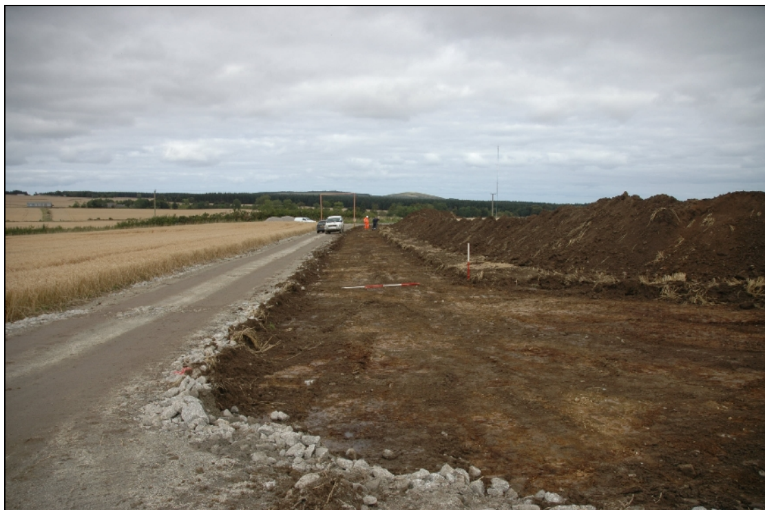
Illus. 3: Cable trench corridor running N from Turbine 1.
