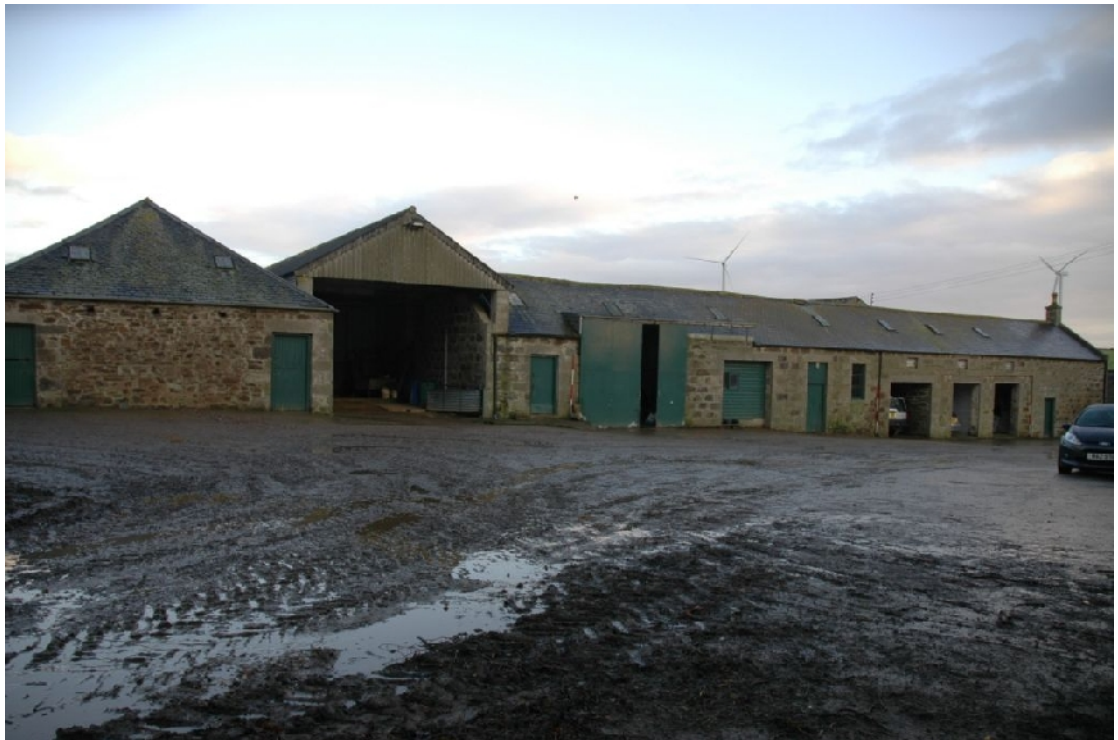
Illus 1 The site, general view looking N
