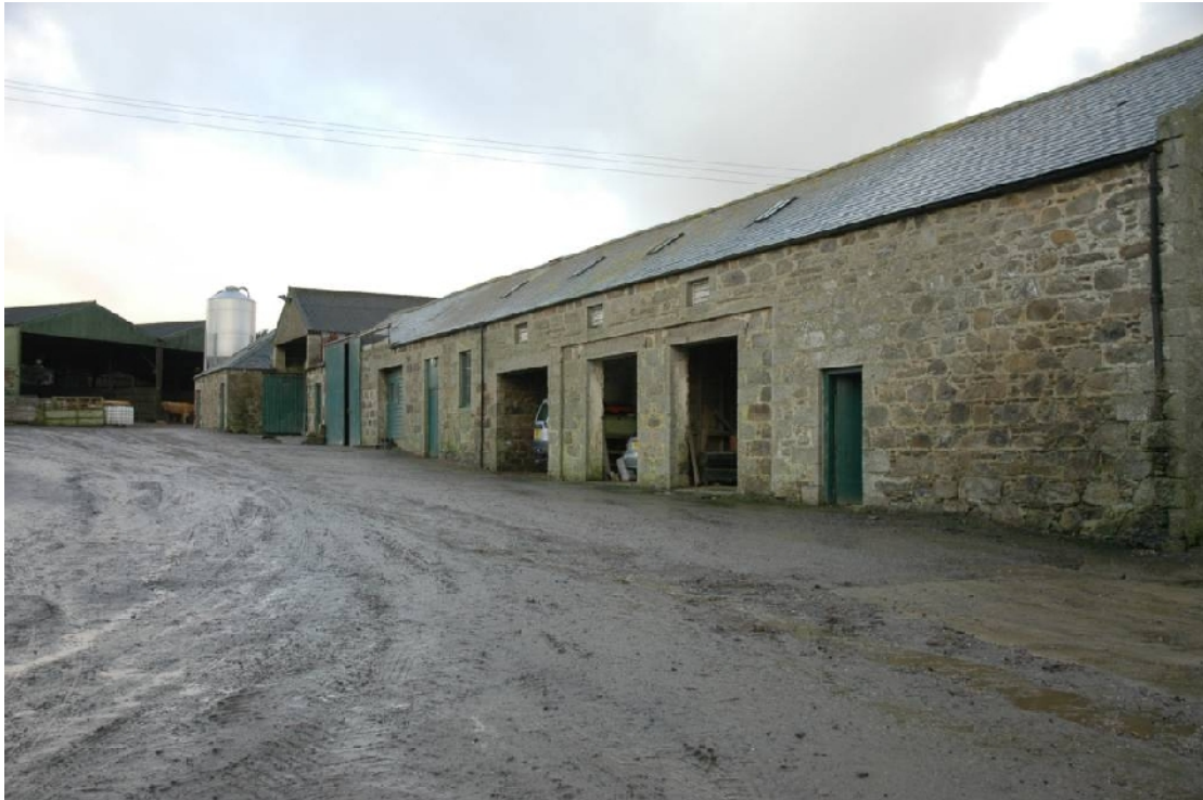
Illus 5 S wall of S range looking W
