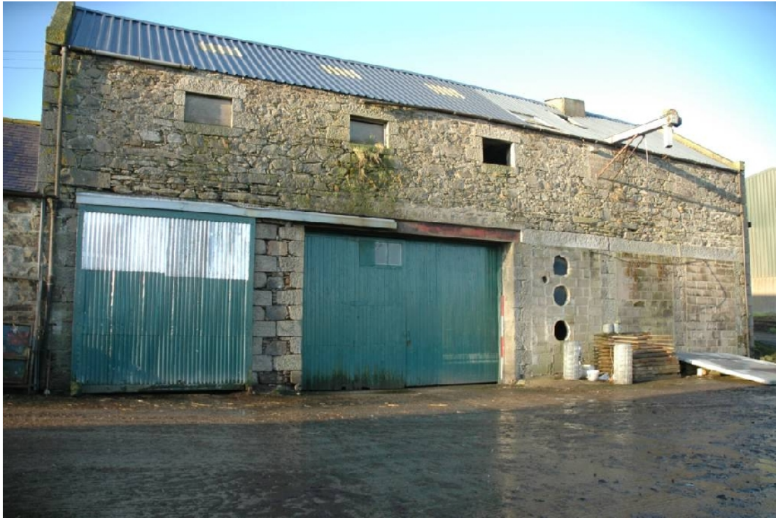
Illus 16 E wall of Building 5
