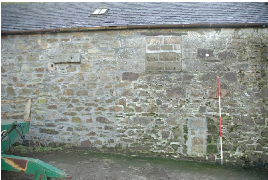
Illus 14 Detail of projecting stone, window to 1 st floor W10 and V2 below. Mill wheel is likely to have been in this area.
