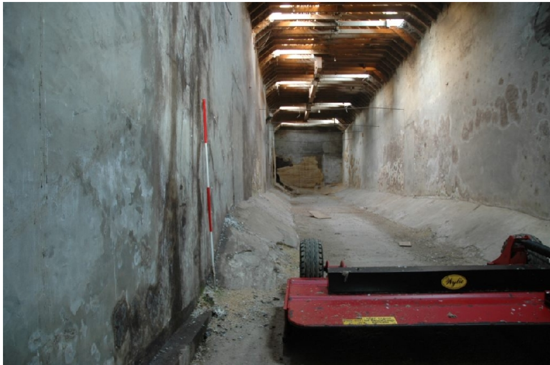
Illus 15 Interior Building 4
