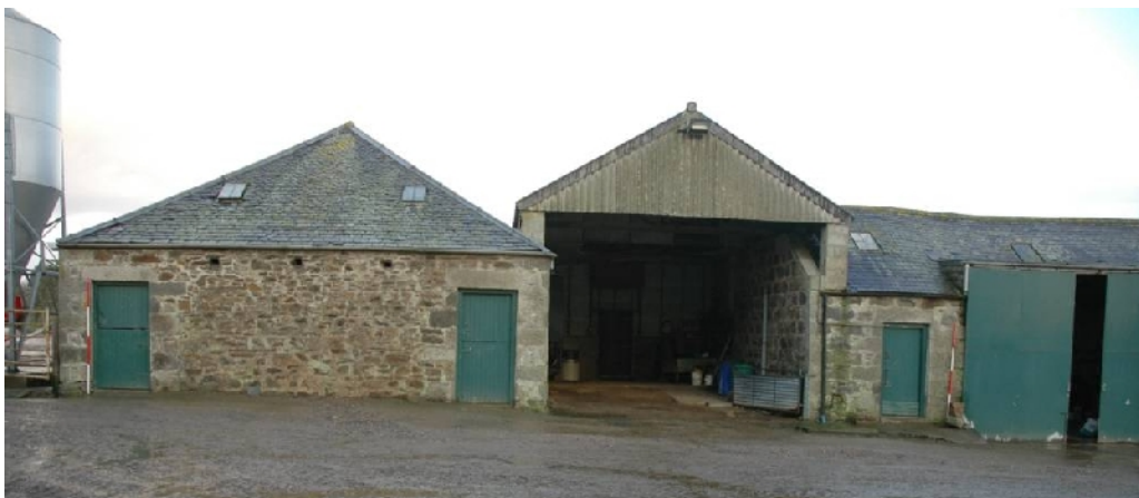
Illus 11 S end of Building 2/3 and the covered passageway between it and the main block Building 1
