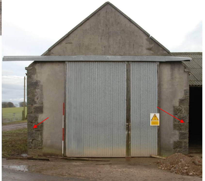
Illus 21 E gables of S range (top) showing pink granite rybats and of N range (below) showing use of grey granite rybats at corners
