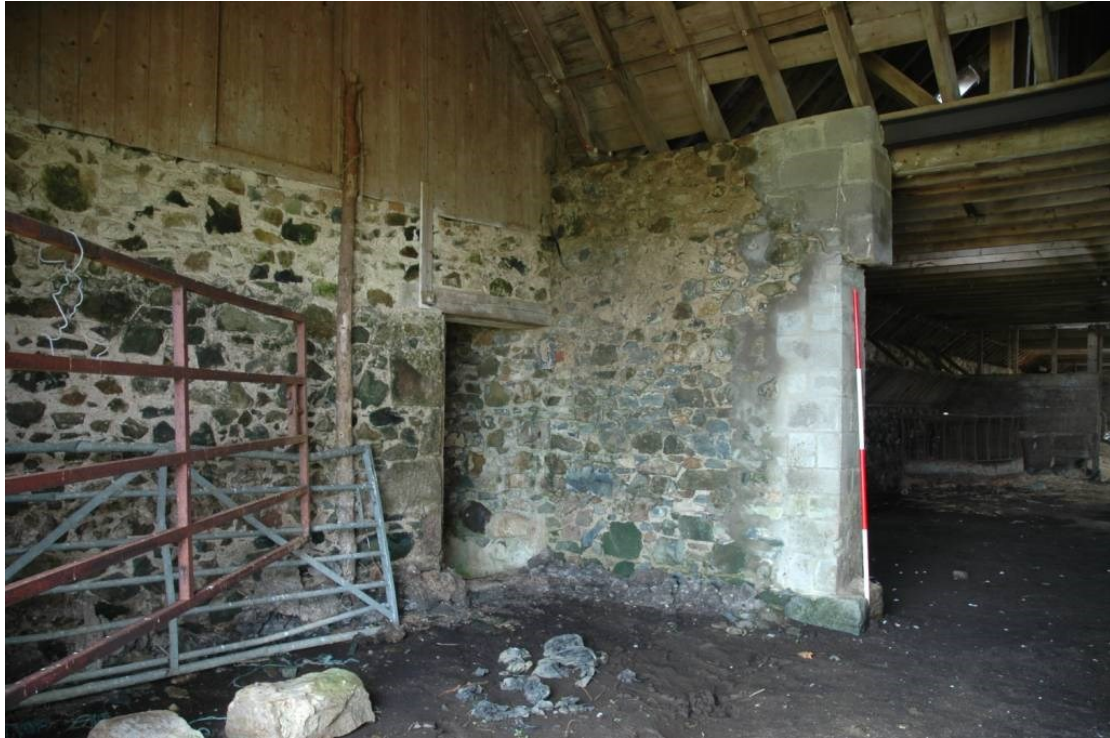
Illus 26 W end of N Range, looking SE showing door to byre and door to hayloft above in wooden upper partition (just L of vertical timber)
