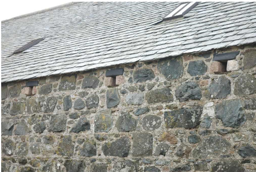
Illus 20 N wall of N Range. Detail of ventilators for byre. These go down diagonally through the wall to avoid draughts.
