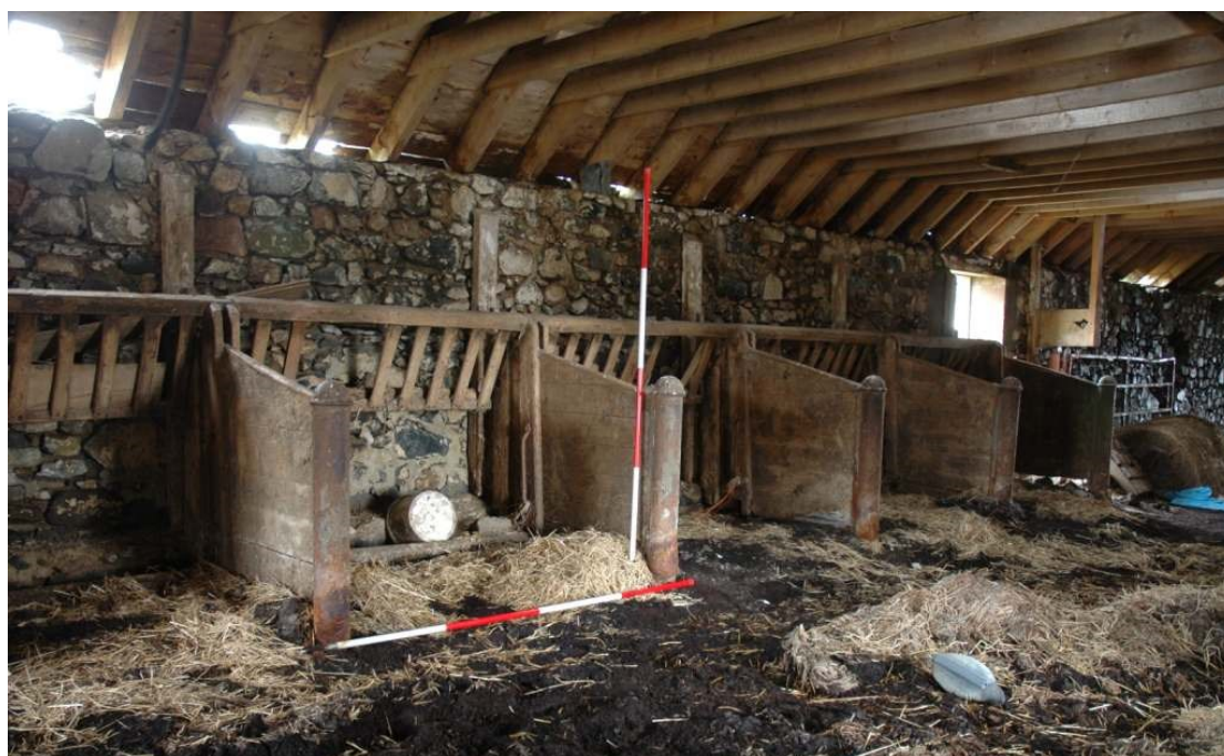
Illus 17 Interior of W Range showing tied cow stalls on W wall
