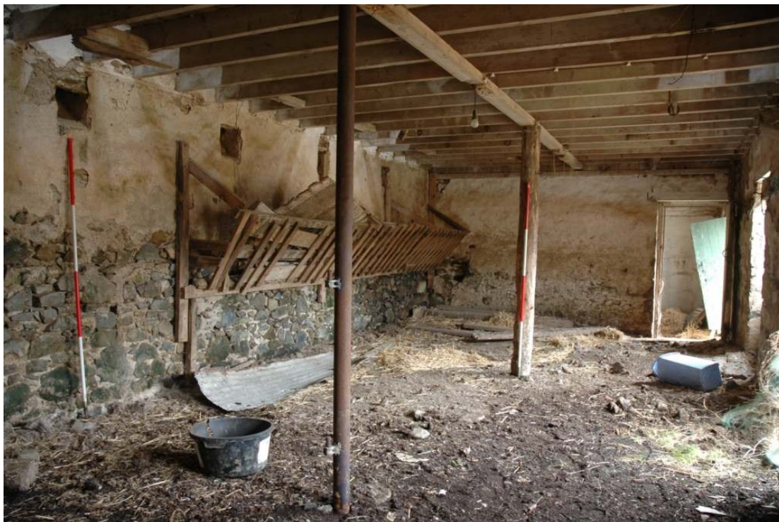
Illus 27 N Range byre. Note the inside of the ventilation shafts in N wall (LHS).
