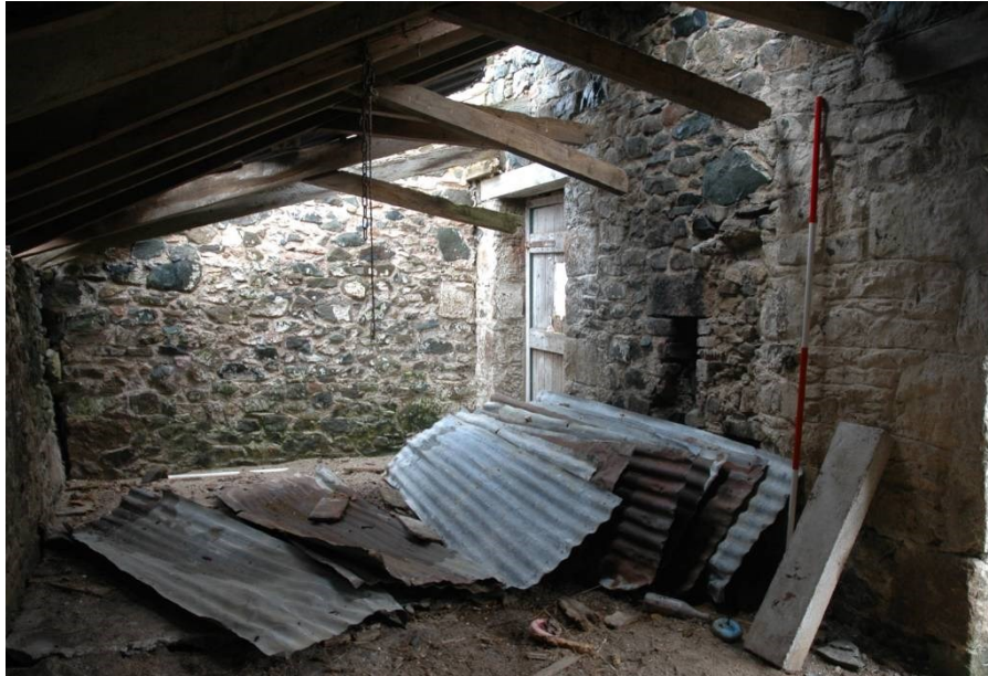
Illus 11 E range interior showing flue below dark coloured lintel in centre of wall. Ranging rod lies just to RHS of former partition.
