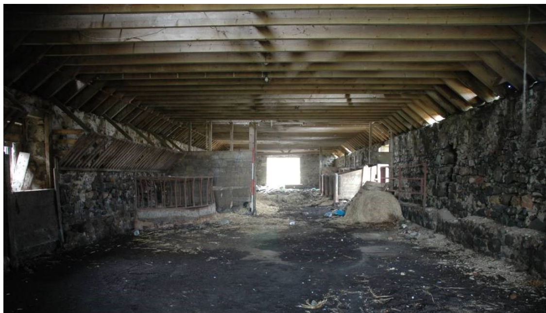
Illus 18 Looking S through W Range with open cattle area in foreground with hay hakes showing on LHS. Wider footings on both sides for feed trough. Tied cow stalls in background.
