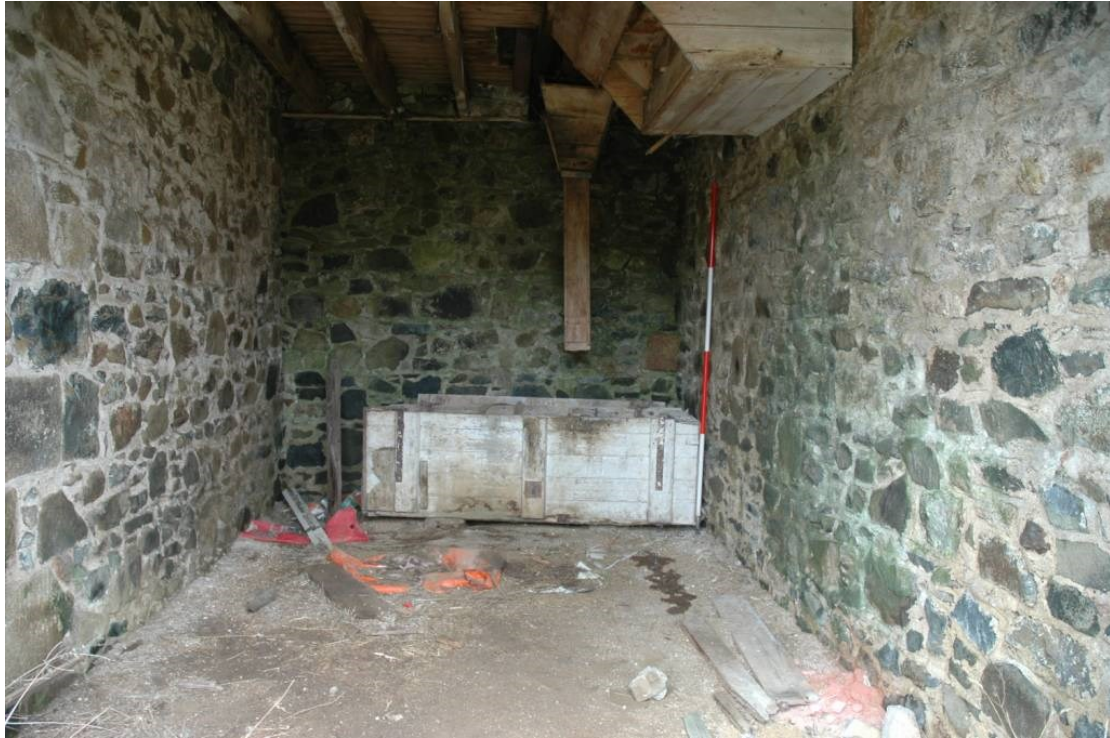
Illus 24 N Range E room with chutes for grain from bruiser (background) and for chaff from thresher (roof foreground)
