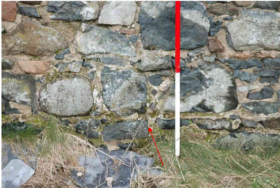
Illus 13 S range. Detail of E end of S wall. Arrow marks the rebuild.
