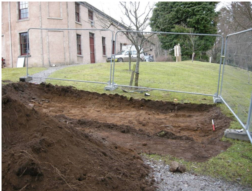
Illus 3 Soakaway in relation to stables, looking N
