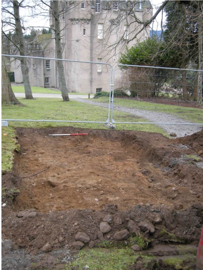
Illus 2 Location of soakaway in relation to castle, looking SE
