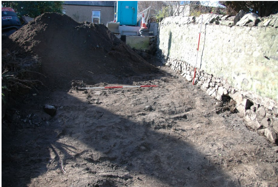
Illus 6: Soil strip over Site 27, looking W
