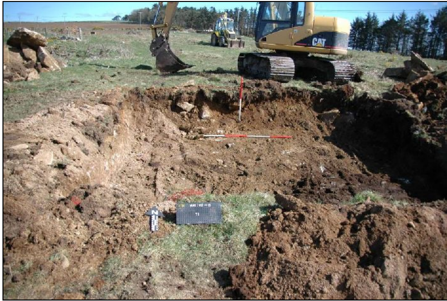
Illus 2: View of base of Turbine 1, looking N
