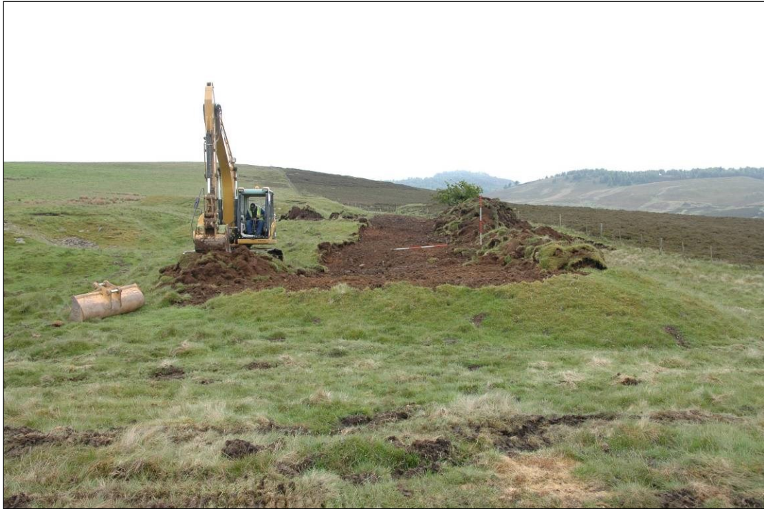
Illus 5: Soil strip on W side of old quarry, looking S.
