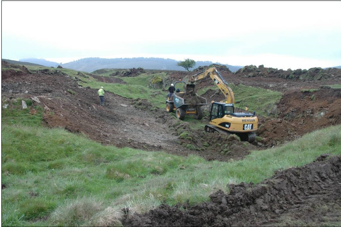
Illus 8: View showing clearance of soil from the W side of the quarry, prior to extraction. Looking SW.
