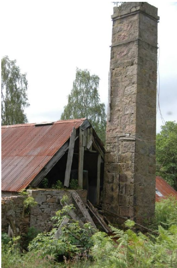
Illus 10 Detail of the chimney
