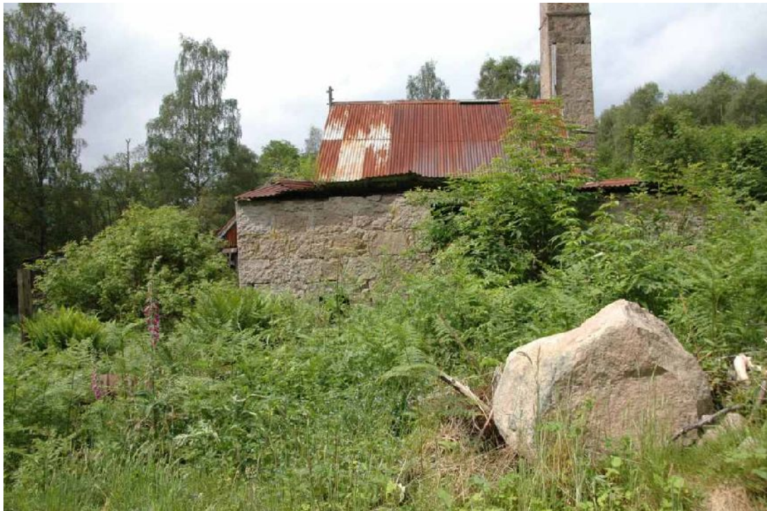
Illus 5 General view E wall Building 1
