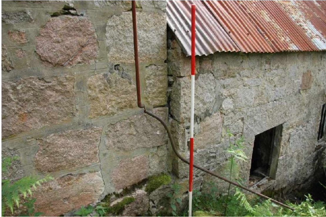
Illus 11 Chimney abutting W wall of Building 1
