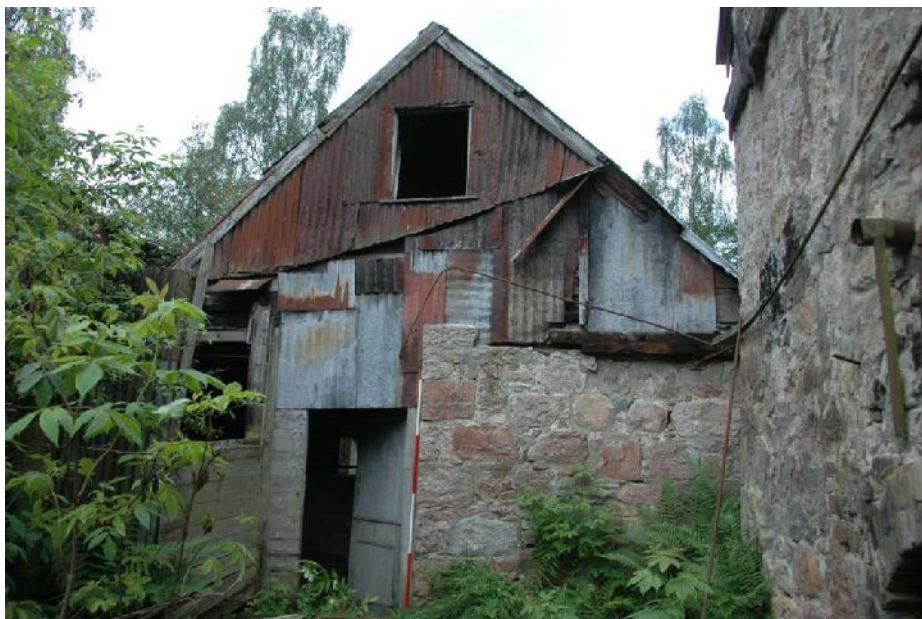
Illus 8 Building 3 E wall, showing fragment of original stone wall
