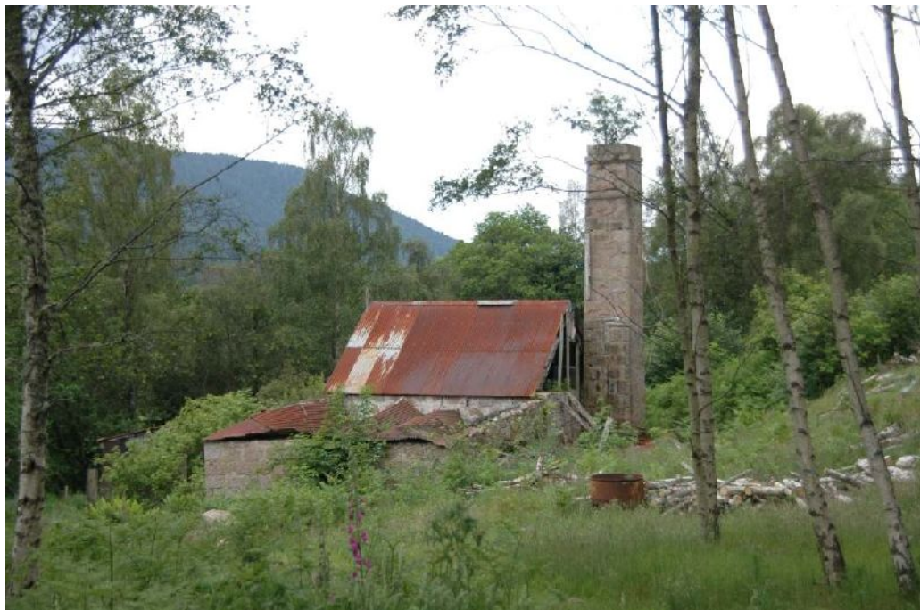
Illus 1 The site, general view looking W
