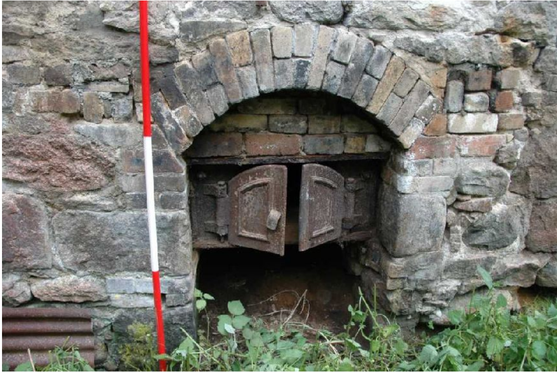
Illus 13 Stoke hole and ash pit (3) in S wall Building 1
