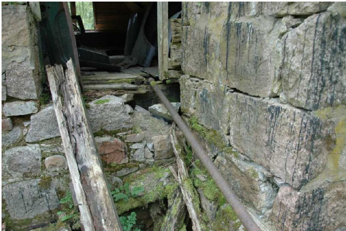
Illus 12 Chimney abutted by N wall Building 1
