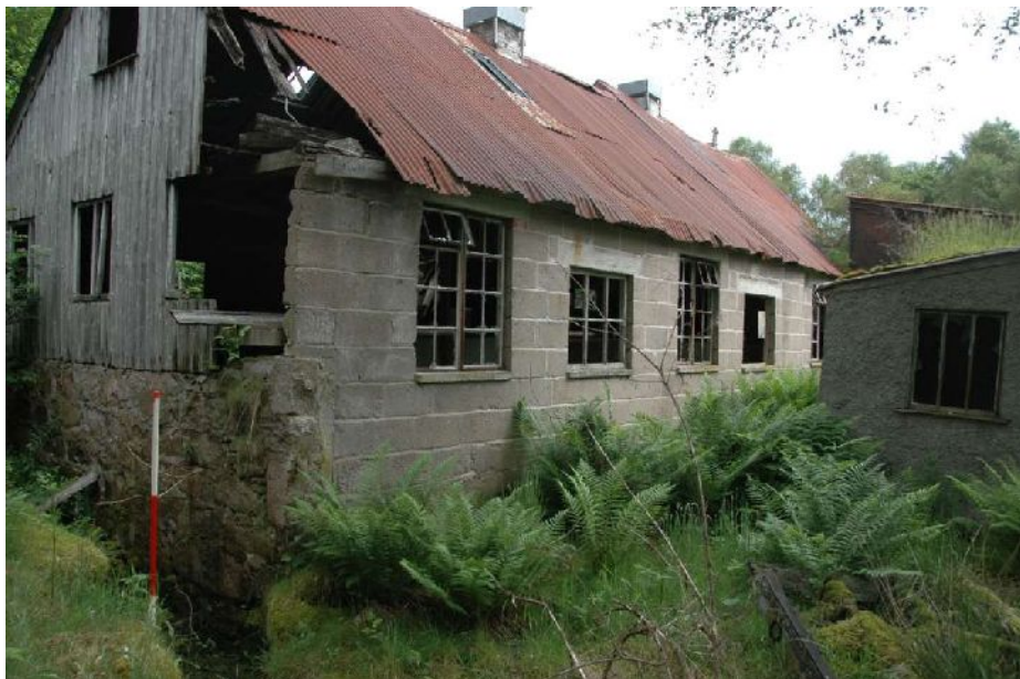
Illus 9 Building 3 SW corner showing fragment of original wall and mill lade
