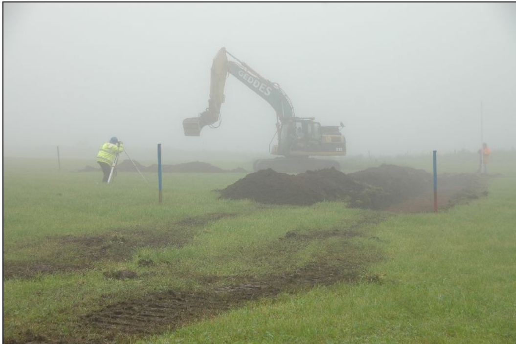
Illus 6: Soil strip over area of Turbine 1, looking NW.
