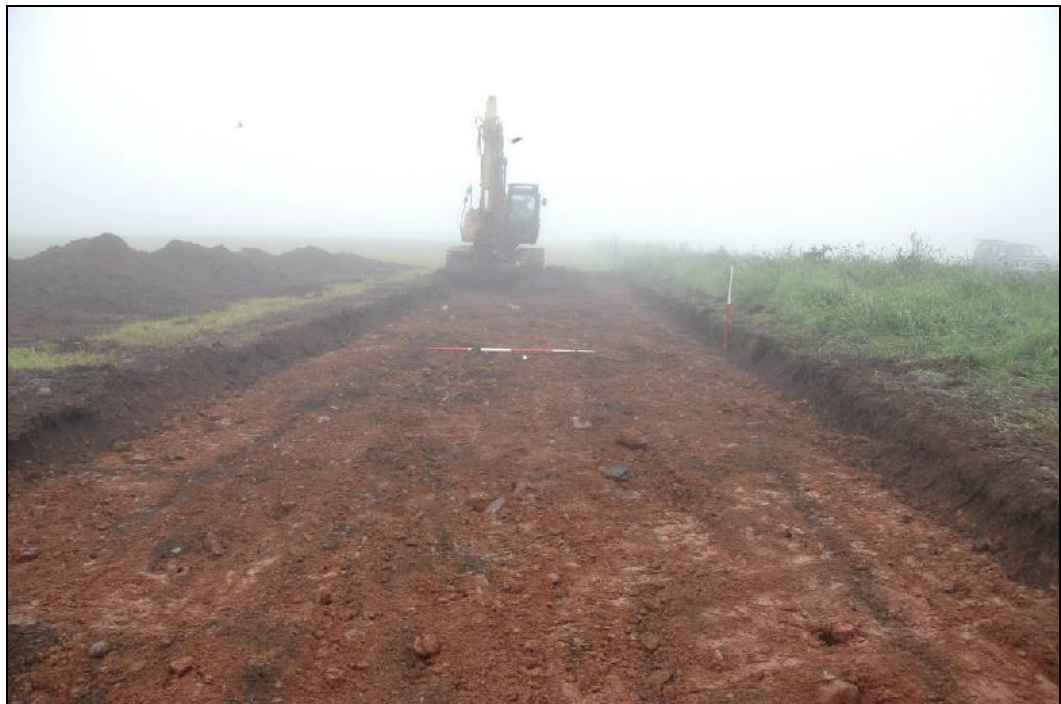
Illus 5: Access track C-D to Turbine 1, looking NW.
