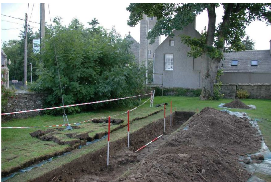
Illus 9 Trench 1 completed, with Parish Church in background
