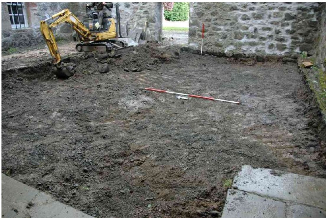
Illus 6 Courtyard from SW corner showing natural rock below the cobbles and leveling topsoil/clay mix.
