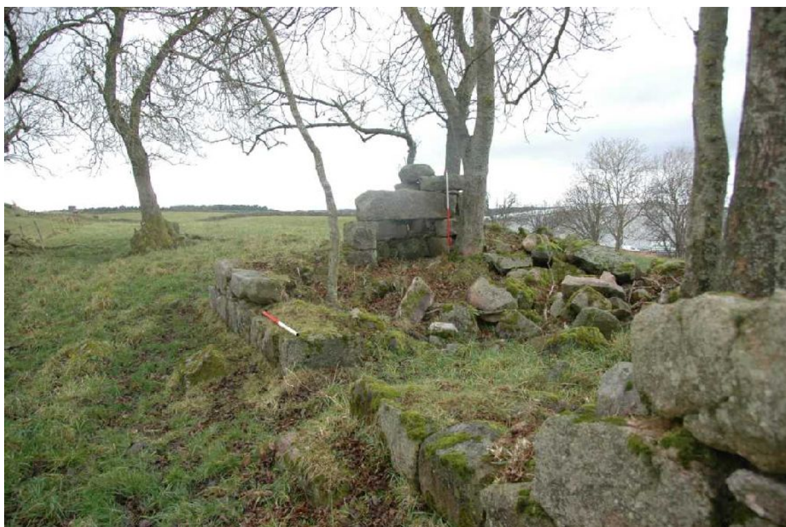
Illus 7 Ruined croft at Denwell. S wall looking towards fireplace
