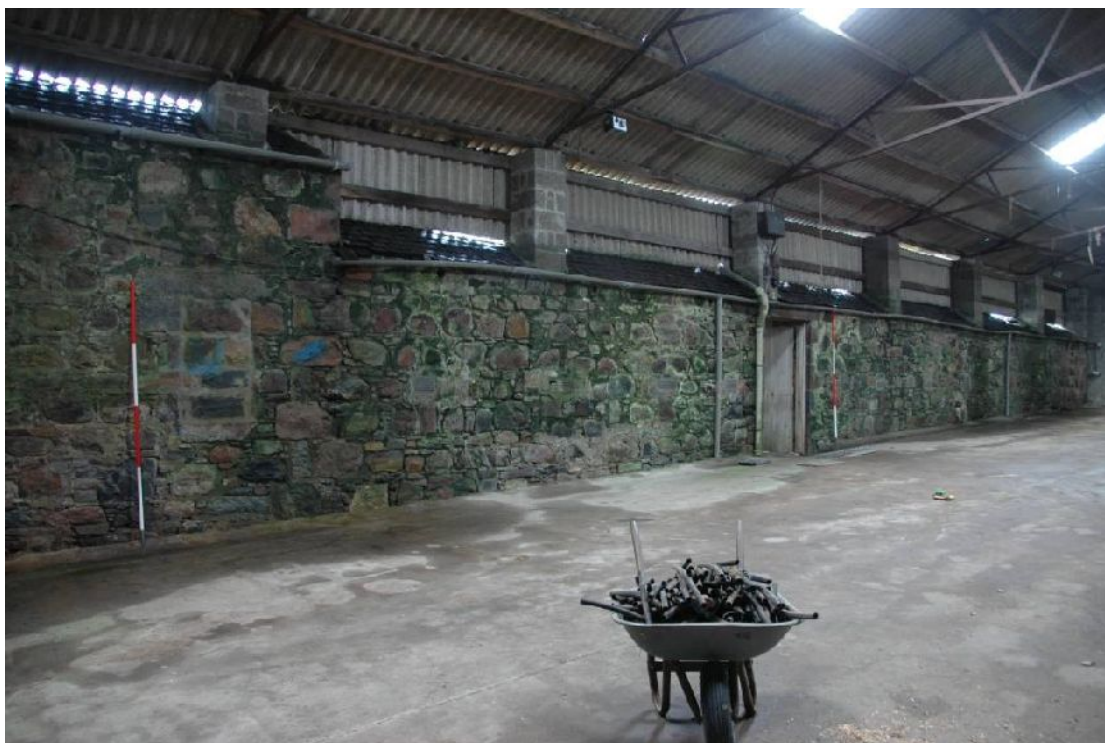
Illus 8 W wall from inside modern shed. Ranging rod in foreground beside W2. Ranging rod in centre beside D5
