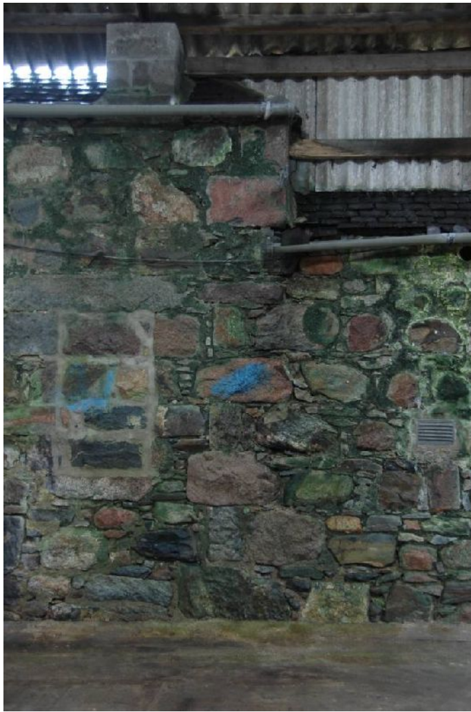
Illus 10 Detail of rybats of original SW corner of N range
