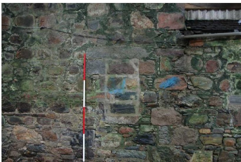
Illus 9 Detail of blocked window W2
