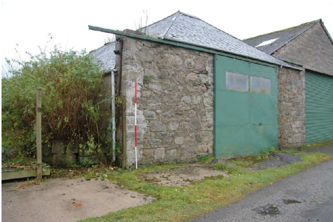
Illus 4 N wall of steading showing concrete block work where the N range had been demolished
