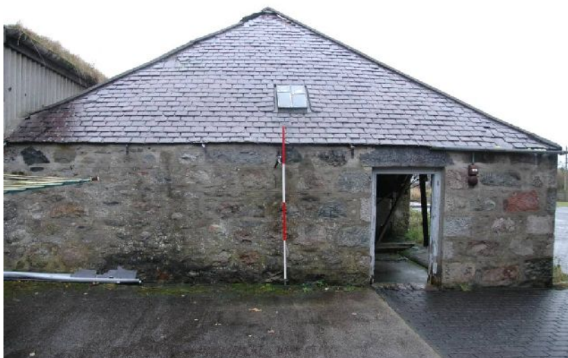
Illus 5 S wall and door D1
